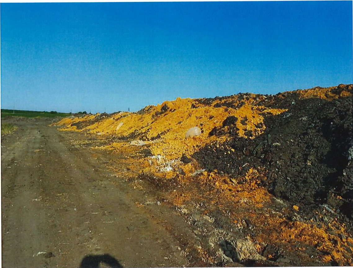
Picture 9. Looking west from the south-central pad perimeter. Compost is off the pad in this area. Material continues to be pushed towards the pad and this berm creates a barrier to keep leachate on the pad.
