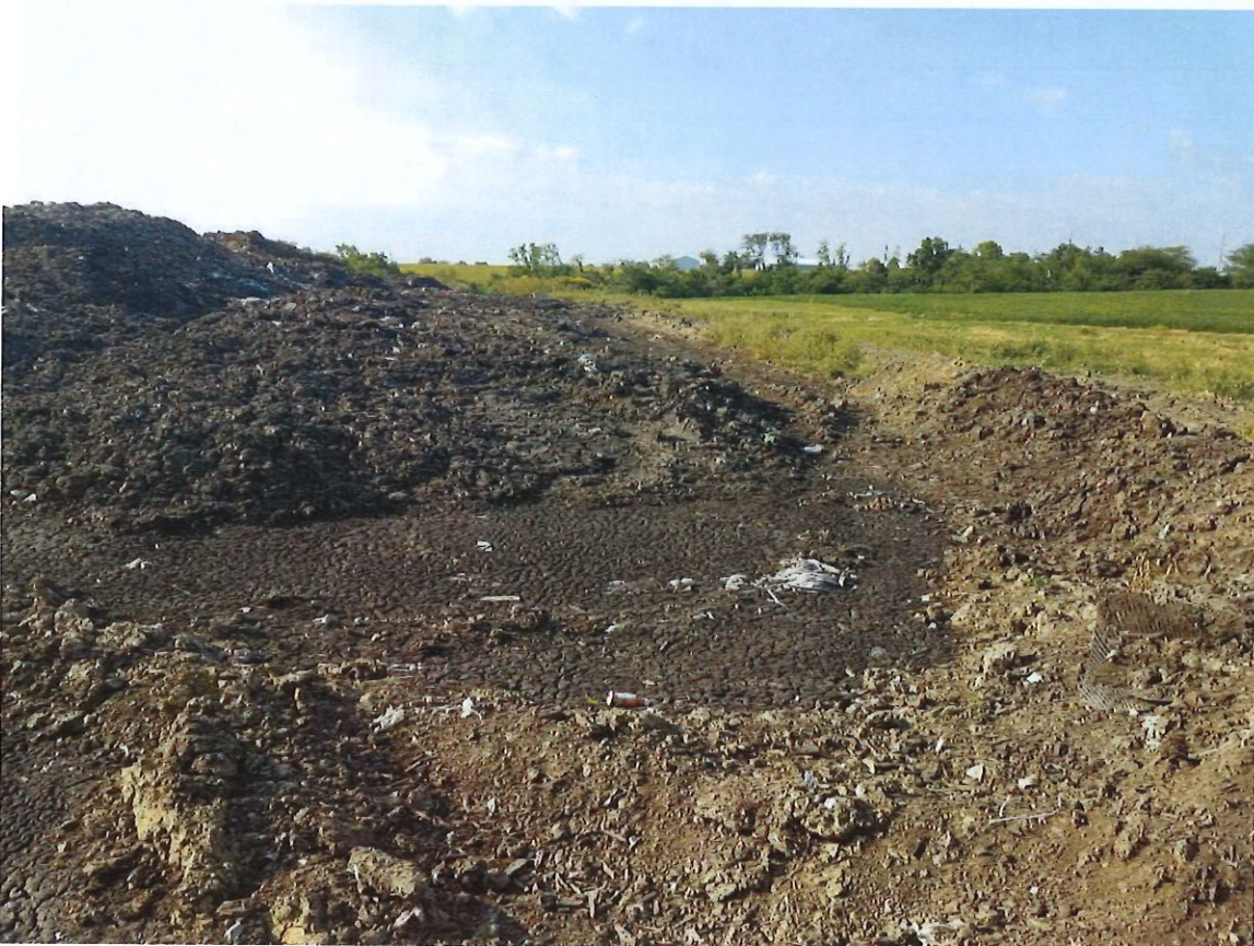
Picture 8. Looking south at the western perimeter. Leachate avenue to southwest drain is not clear. A berm is in place to attempt to keep leachate from migrating of the pad.
