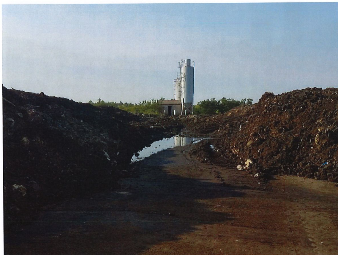
Picture 2. Looking south from the east-central perimeter of the pad. Leachate does not have an open avenue to discharge to the east lagoon. A cut drain through the pad lies just beyond the end of this path.
