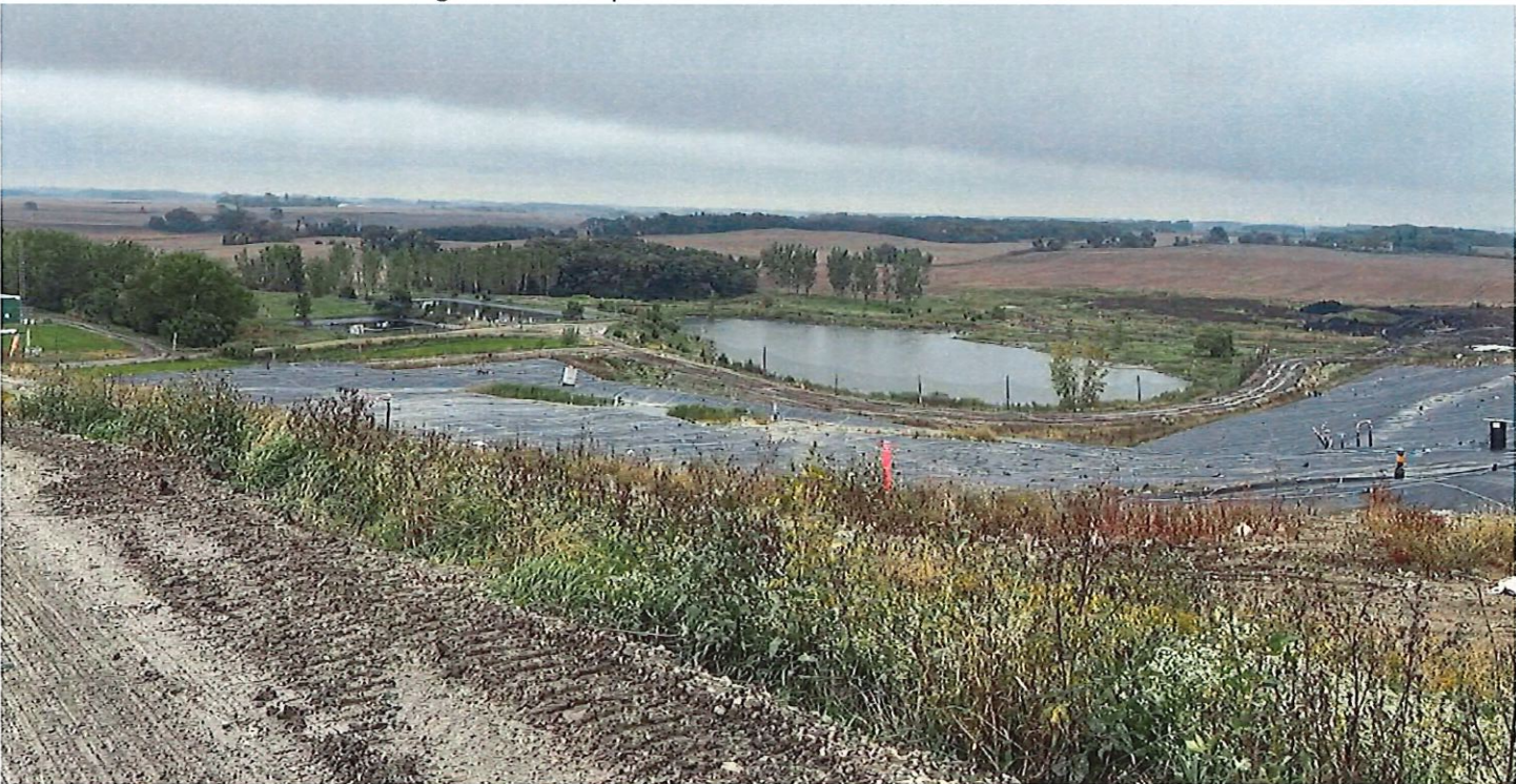
Photo 2. New 20' litter fences along stormwater pond
