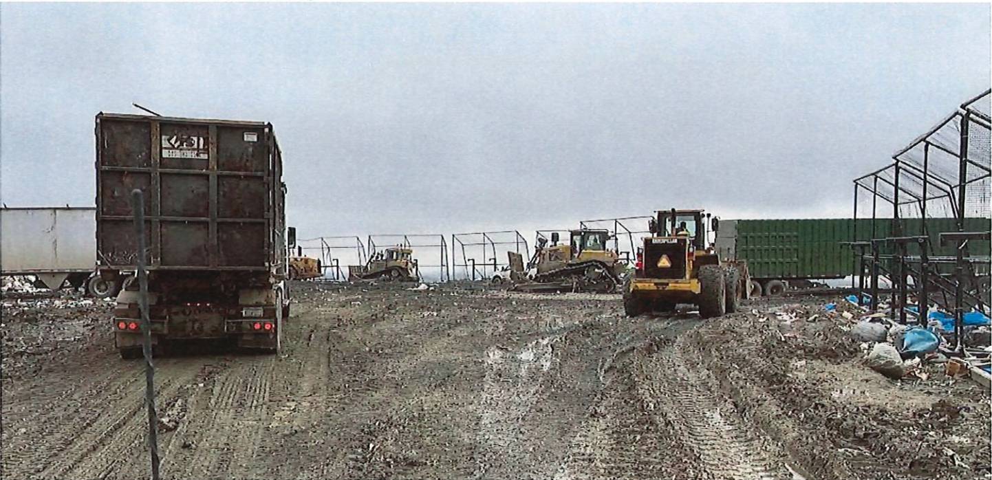
Photo 1. New Litter Fences at Working Face
