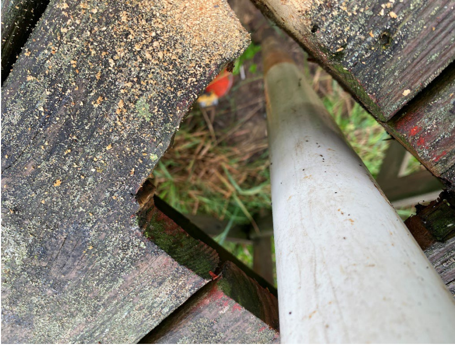
Photo 7: Made minor cuts on either side of well to lift protop off well. (Looking down)
