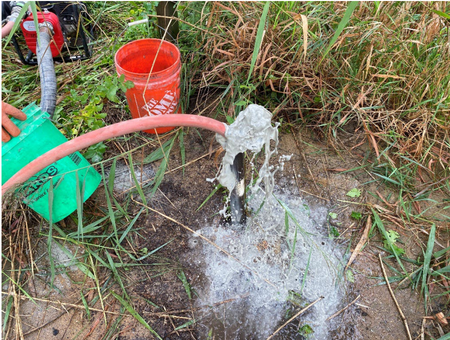
Photo 13: Grout overflowing from well after tremie piping from bottom to surface. (Looking down)
