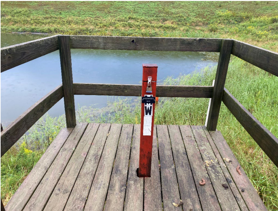
Photo 4: MW-17 condition prior to abandonment. (Looking east)
