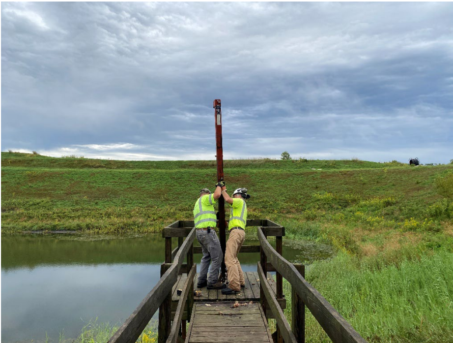
Photo 8: Removing MW-17 protop. (Looking east)
