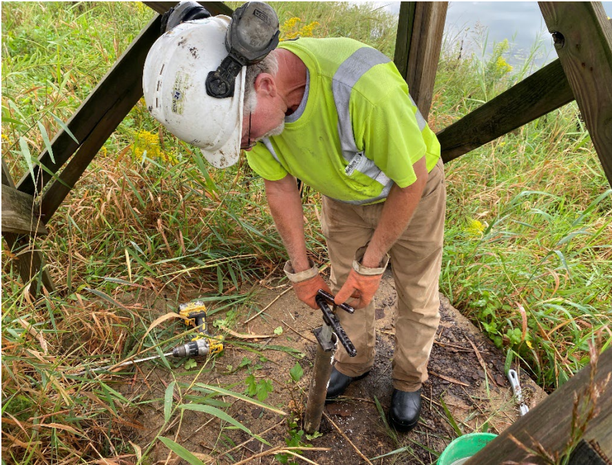
Photo 11: Certified driller cutting PVC to 4 feet below ground surface. (Looking down)
