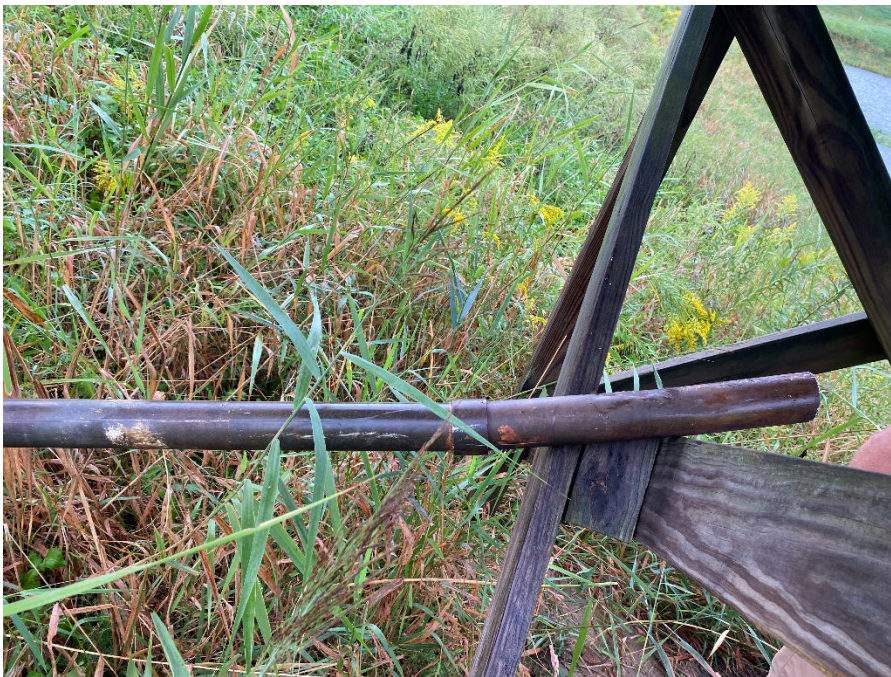
Photo 10: Cut PVC stickup. (Looking down)
