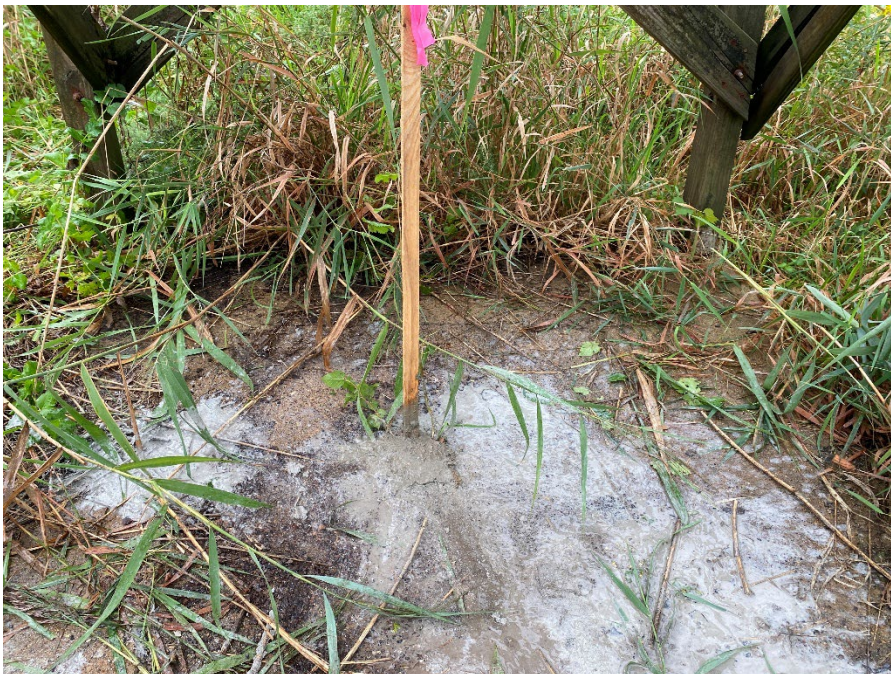
Photo 14: Final abandonment. PVC cut to approximately 4 feet bgs and protop to ground surface. The concrete pad supports the wooden structure so it could not be fully removed. Hole topped with granular bentonite, sealed with concrete.
