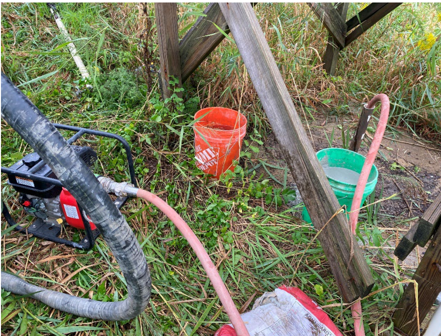
Photo 12: Tremie set up to abandon MW-17 with grouting from the bottom up. (Looking down)
