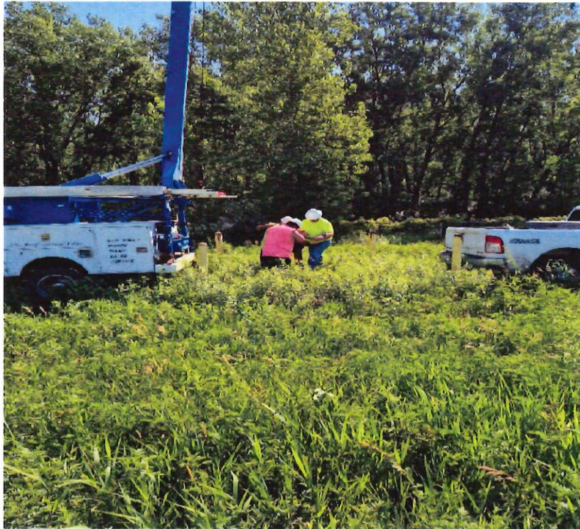
Georgia-Pacific Gypsum North Recycle Pile – Monitoring Well MW1 Removal (July 8, 2026)
