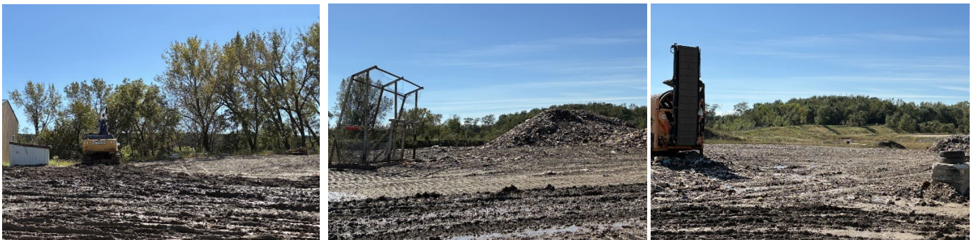
Southwest cell (west of the equipment building), screening area prior to the stormwater basin
