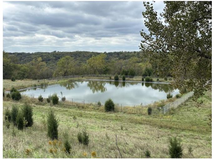
west side leachate lagoon
