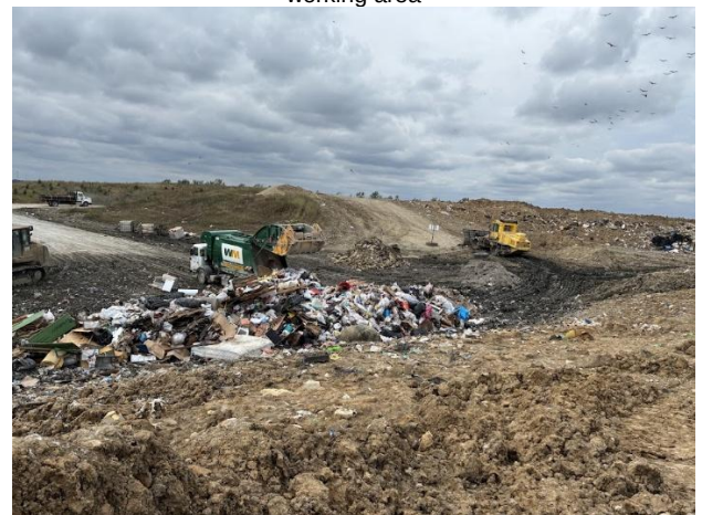
wet weather conditions at working face
