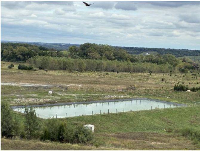
east side leachate lagoon
