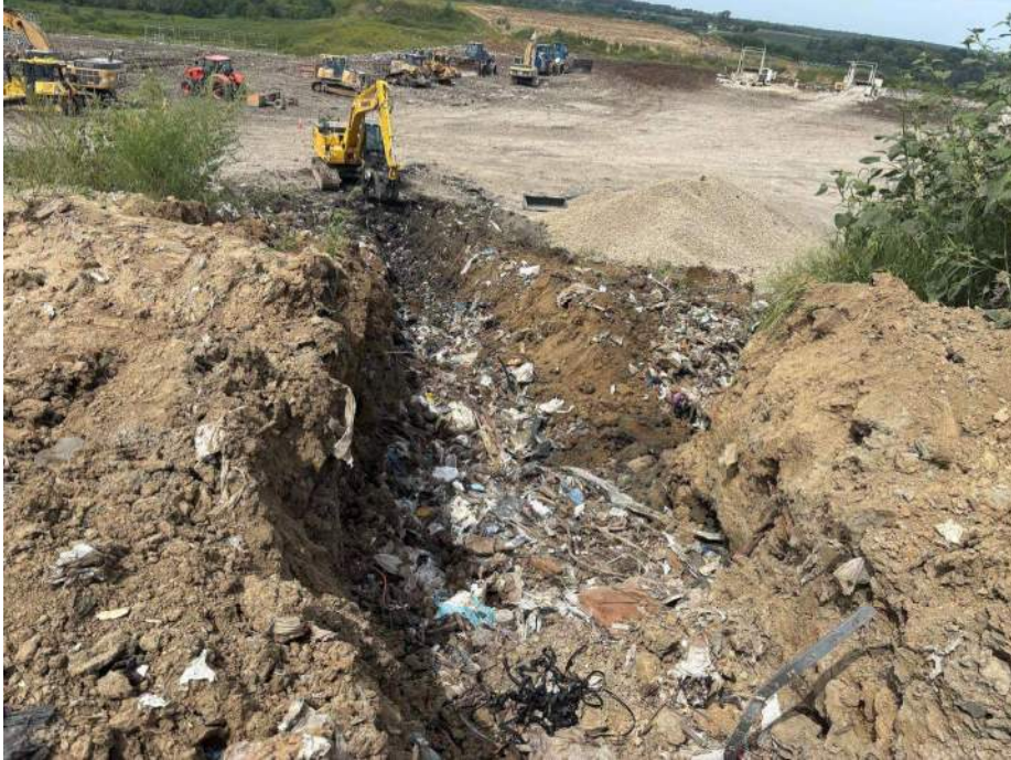
Photo 5: HEW – 9 is trenched.
