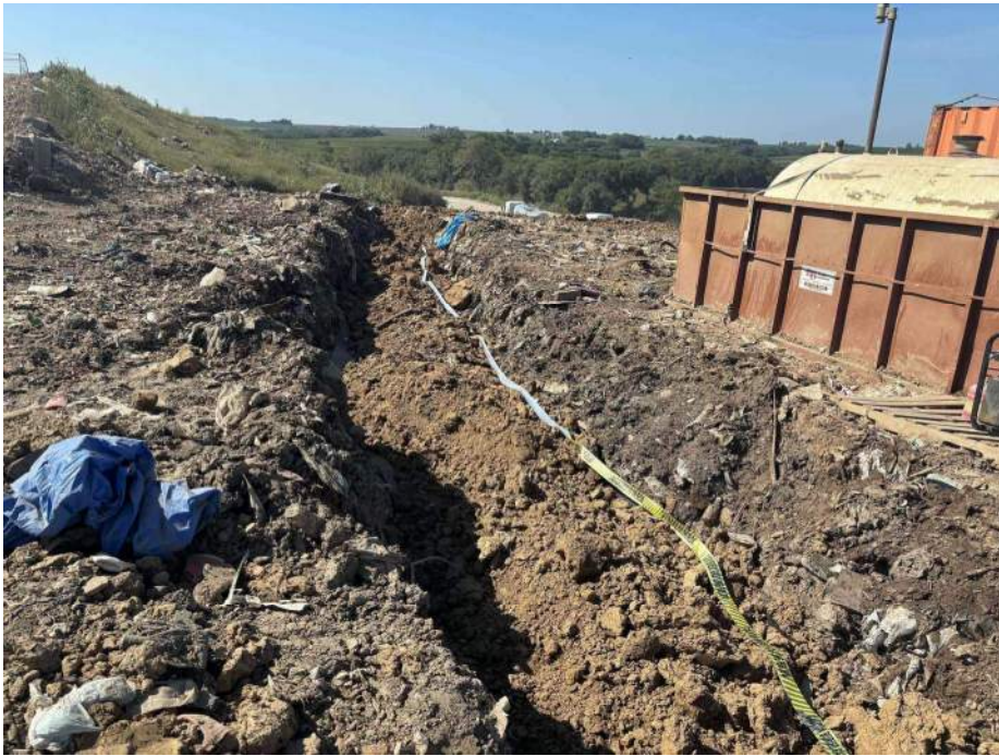
Photo 3: Clean soil and caution tape are placed at HEW – 11.
