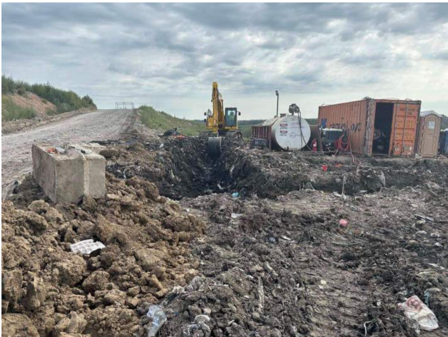
Photo 8: The excavator trenches HEW – 11.
