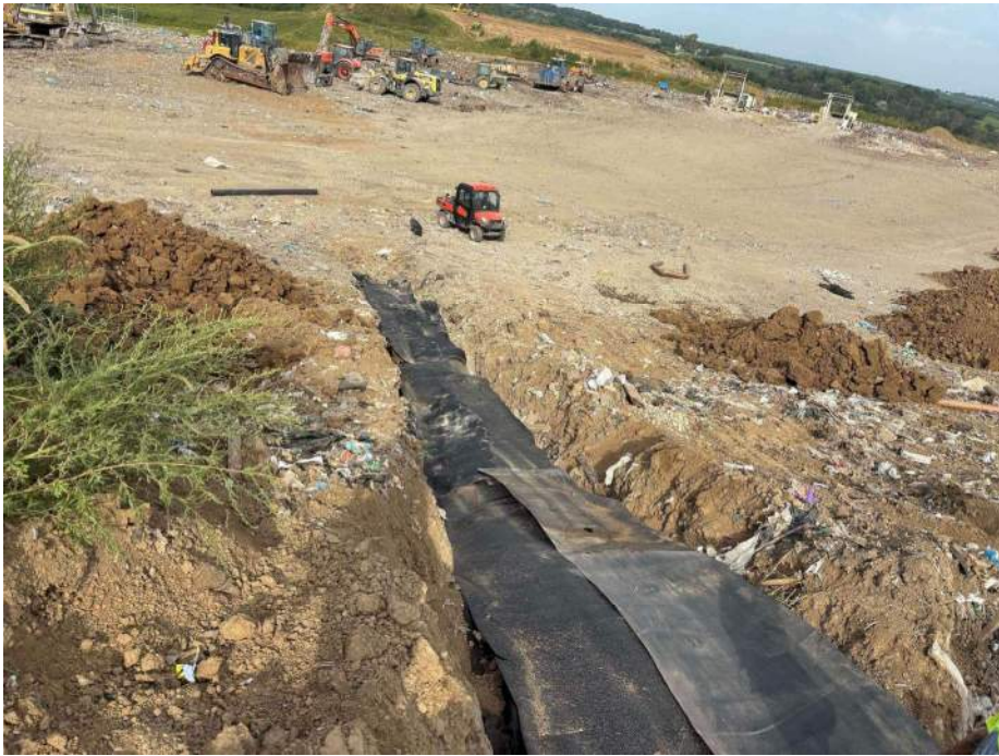
Photo 1: Geomembrane is laid in a wider layer at HEW – 9 (shown) & 8.
