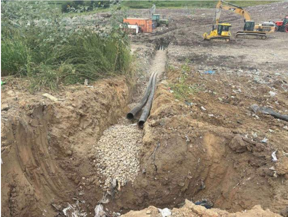
Photo 3: HEW – 10 & 11 are laid and noncalarerous gravel is placed atop.
