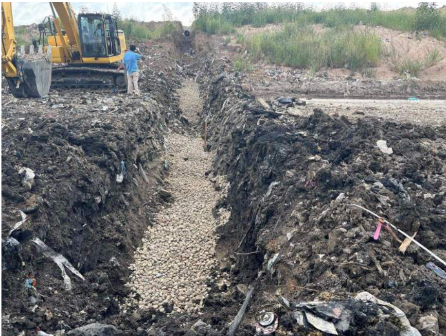
Photo 2: A 1.5' bed of noncalcareous gravel is laid.
