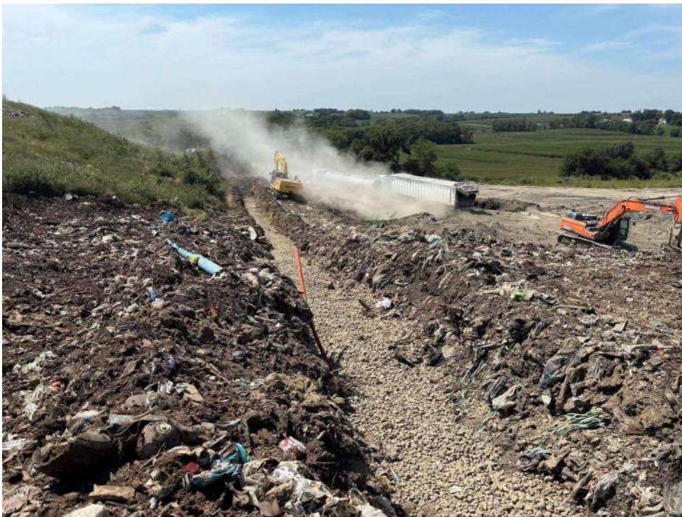
Photo 2: Noncalcareous rock is placed to cover the piping.
