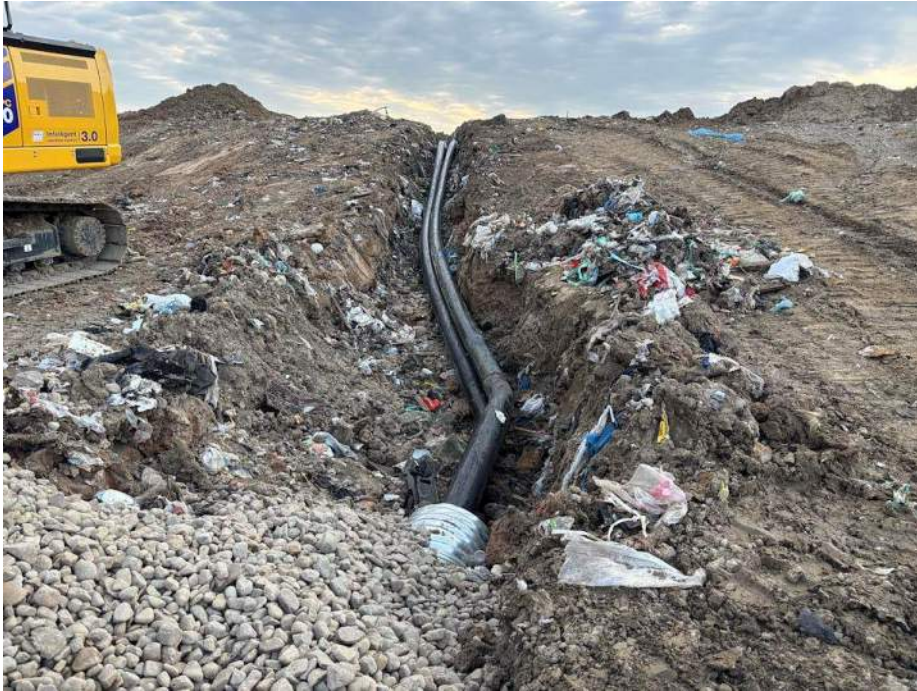
Photo 1: HEW – 10 & 11 are installed from the east point through the road crossing.
