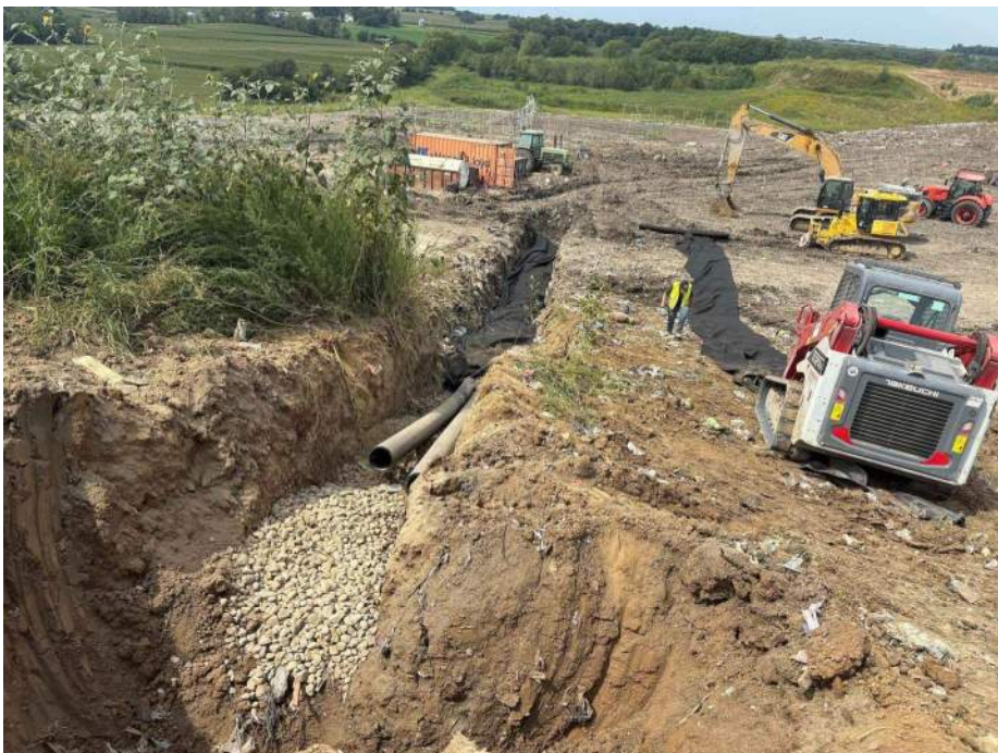
Photo 4: Geotextile is placed
