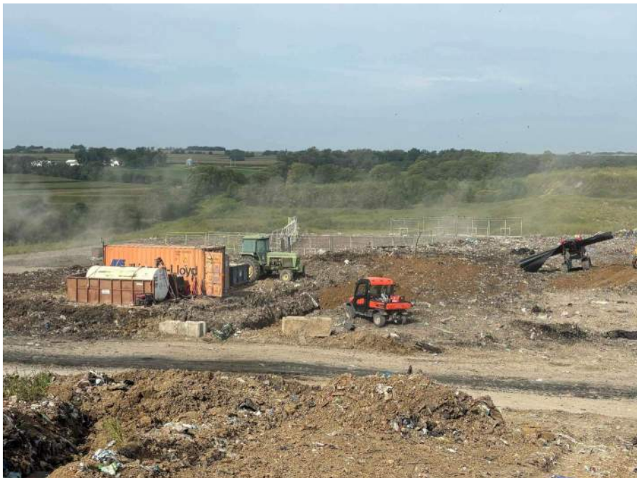
Photo 2: HEW – 10 is backfilled.
