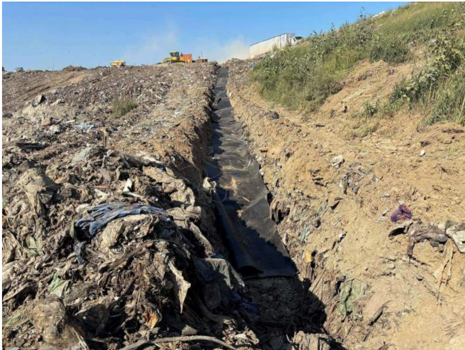
Photo 4: Geotextile at HEW – 11.
