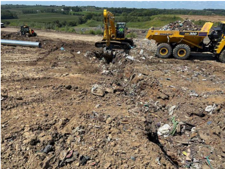
Photo 2: Trenching for the north road crossing.
