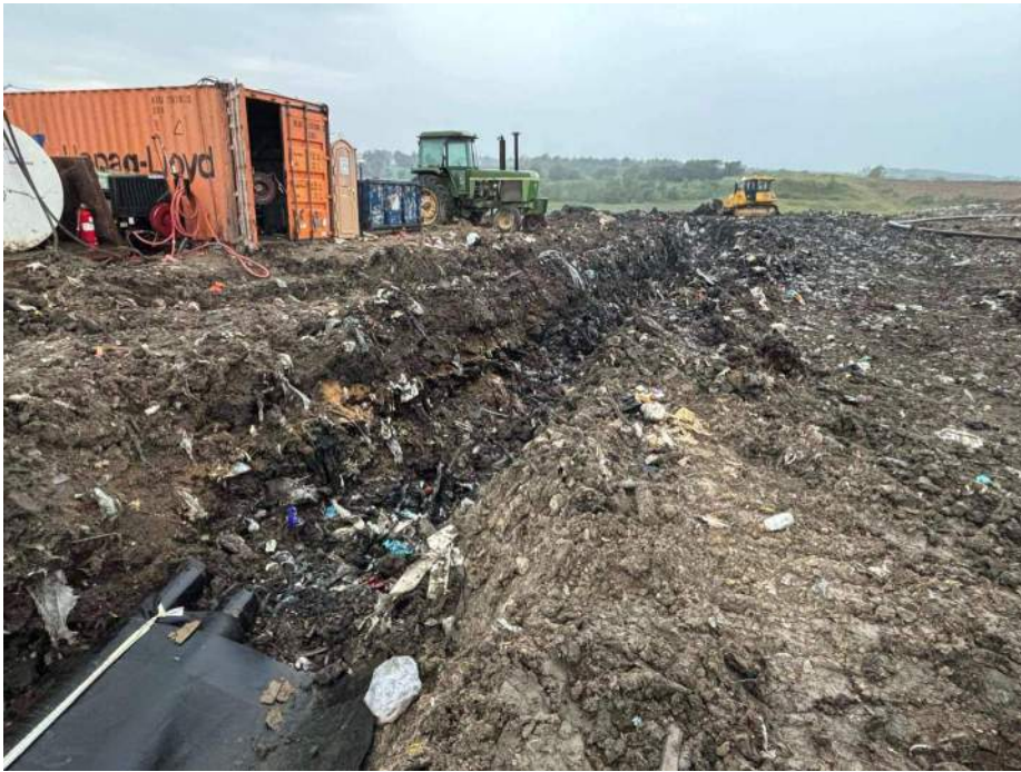
Photo 1: Finished trench for HEW – 10.
