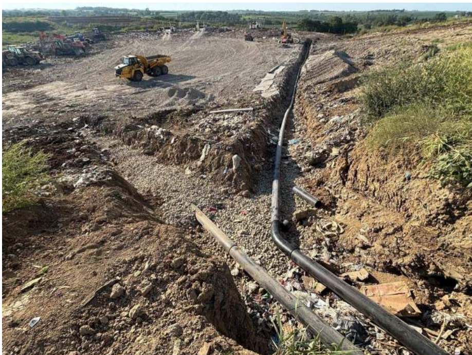
Photo 6: Solid to perforated pipe tie-ins.
