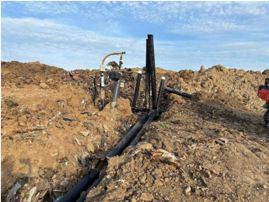
Photo 8: Tie-in is complete at GEW – 87.
