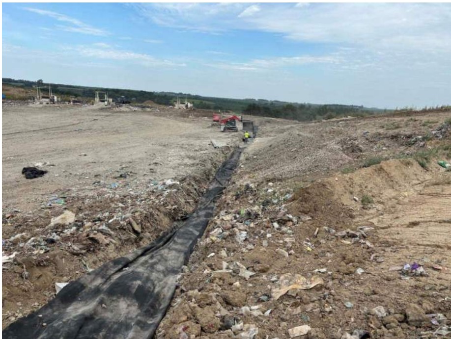
Photo 4: Geotextile is laid in HEW – 8.
