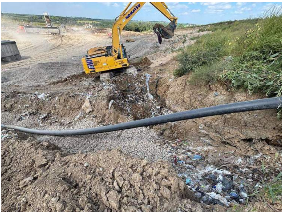
Photo 2: The excavator trenches HEW – 8.
