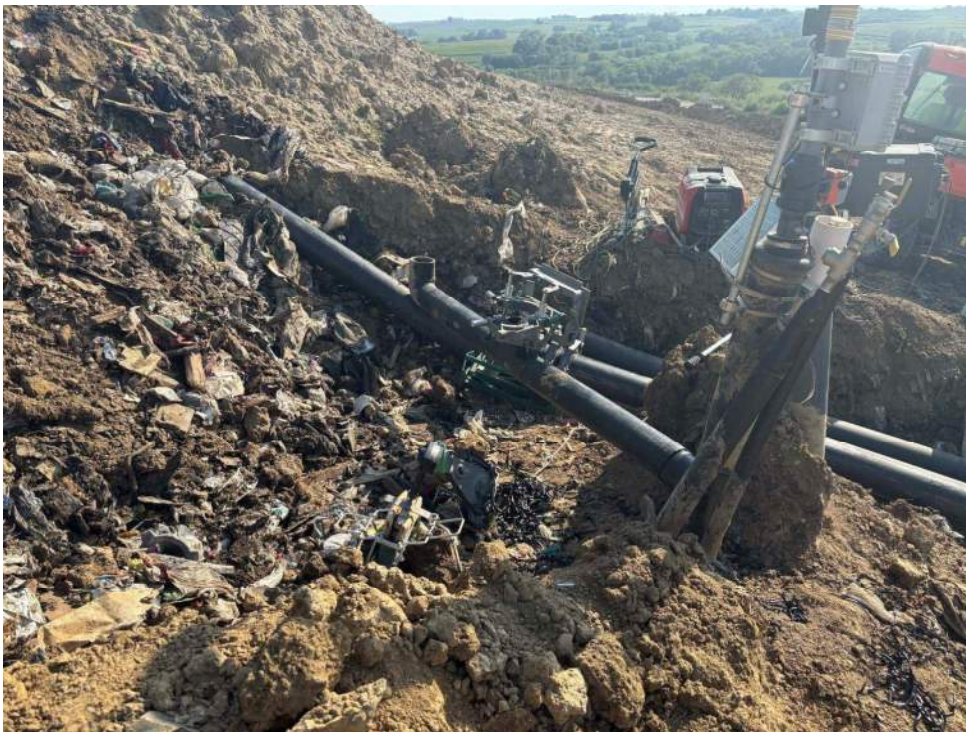
Photo 6: Tie-in at GEW-53R begins.
