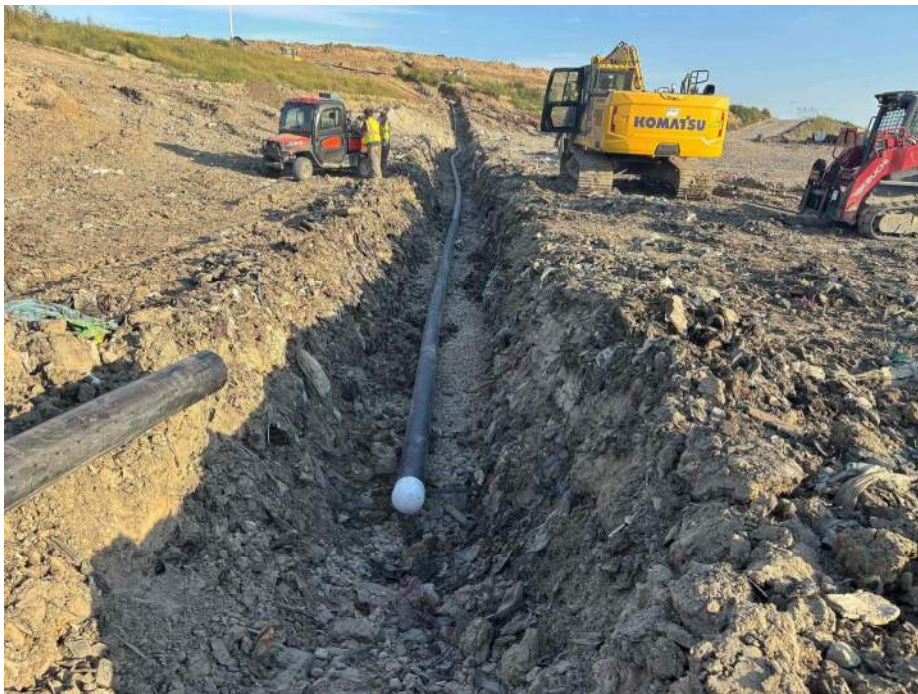
Photo 5: 8" perforated pipe placed at HEW – 8.
