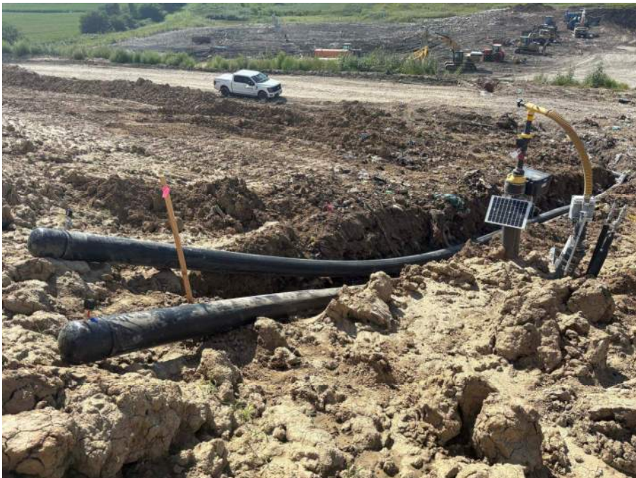
Photo 2: Pressure tests # 1 – 4 are completed (featuring HEW – 10 & 11).
