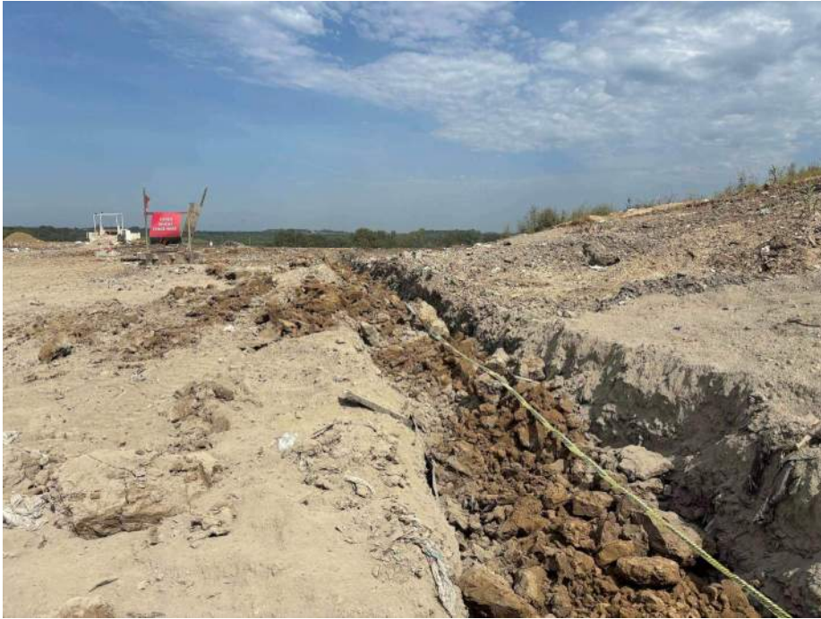
Photo 3: Caution tape and the first layer of clean top soil is placed at HEW – 8, after the branch off point from HEW – 9.
