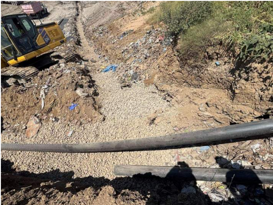
Photo 4: 5' gravel windows extending 3' into each branch, backfilled with noncalcareous gravel.
