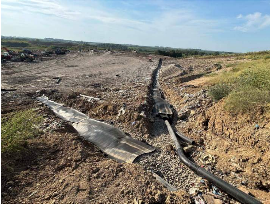
Photo 7: Geotextile laid at HEW – 8 & 9. Skinny pieces will be fixed the following day.
