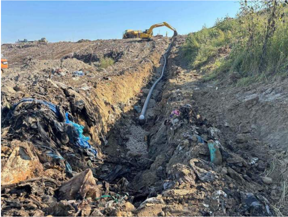
Photo 1: 8" perforated pipe is laid in HEW – 11. Noncalcareous rock is laid atop.
