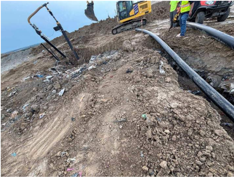
Photo 1: Area around GEW – 87 is getting prepared for the tie-in.
