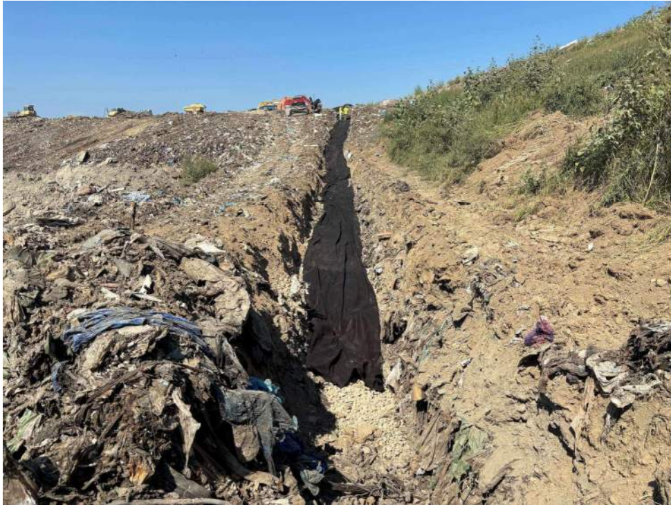
Photo 3: Geomembrane laid at HEW – 11.
