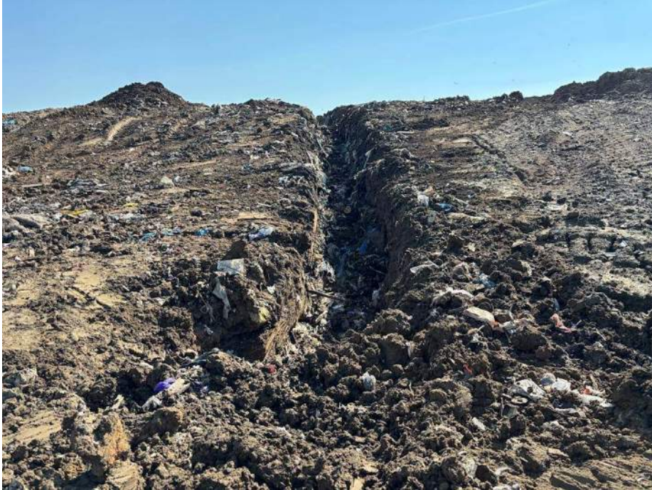
Photo 1: Trench for HEW – 8 & 9 east of the road crossing is complete.
