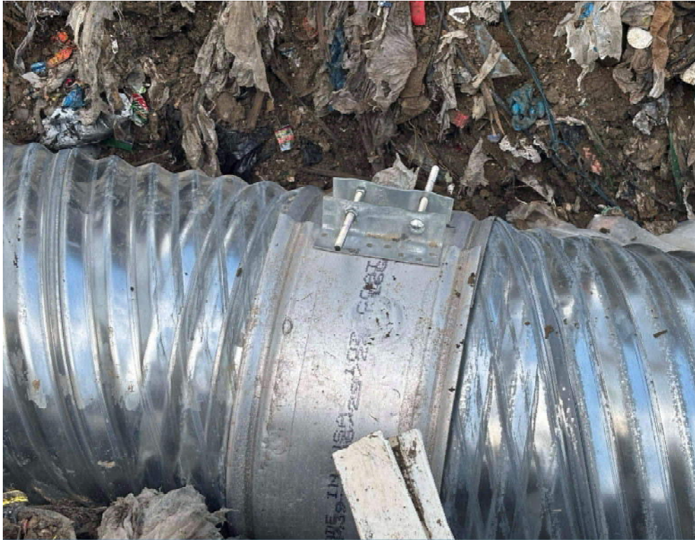
Photo 3: Road crossing casing joint point example.
