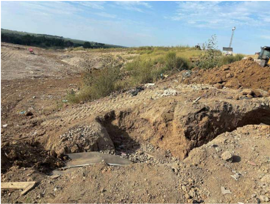
Photo 15: Final conditions documented at the drainage window on the southern line.
