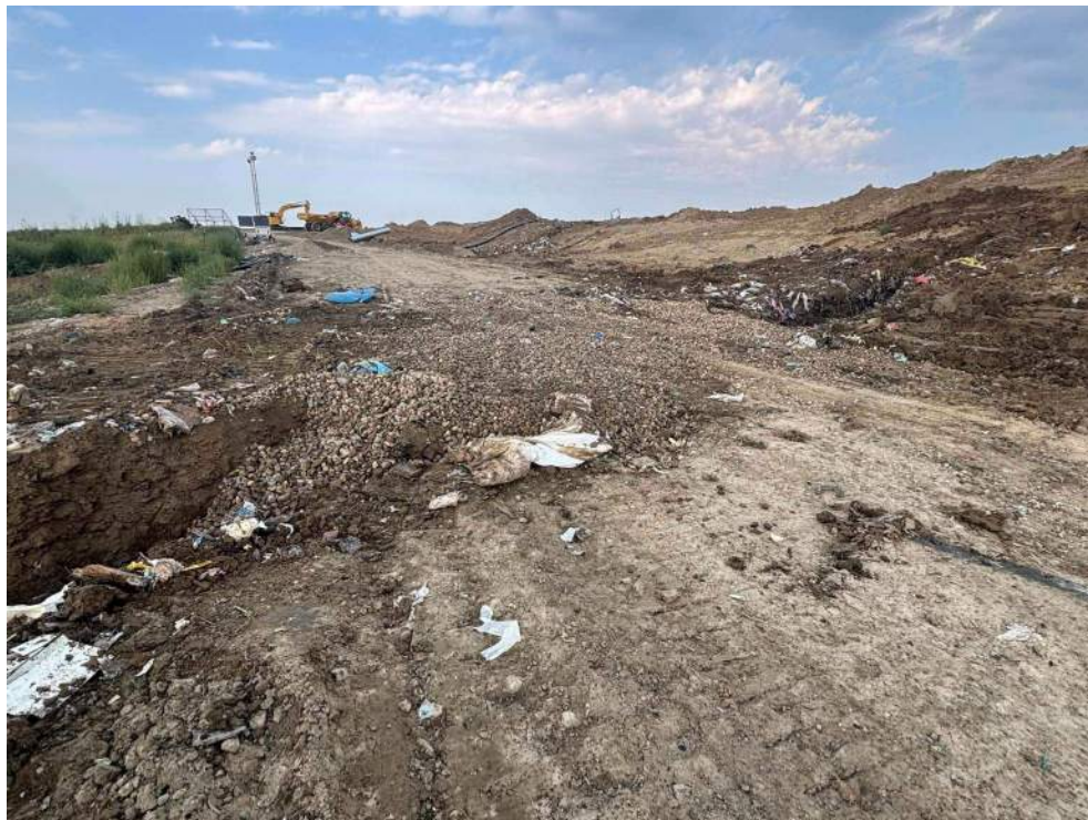
Photo 5: Noncalcareous gravel was backfilled to complete the day.
