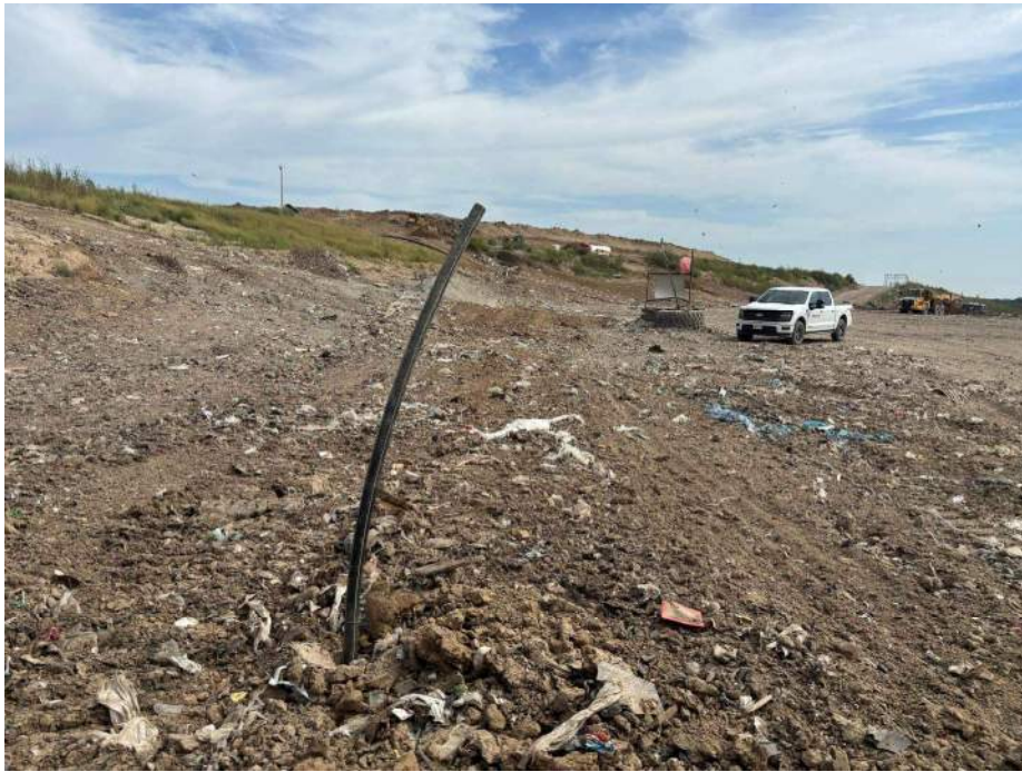
Photo 7: HEW – 8's final grading observed with end survey marker in place.
