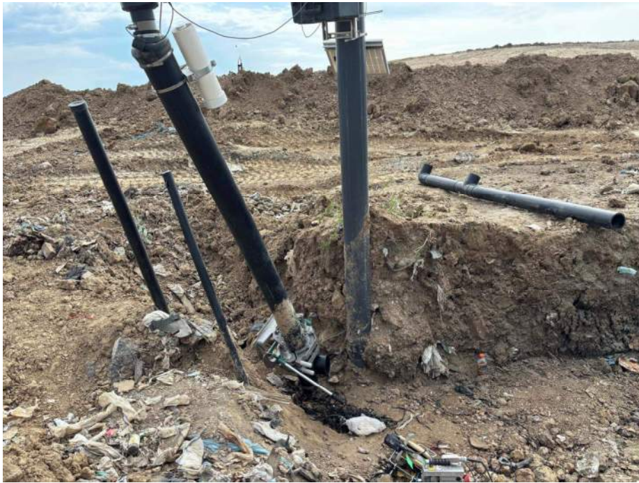
Photo 3: Molded SDR 17 Tee is welded onto the riser pipe.
