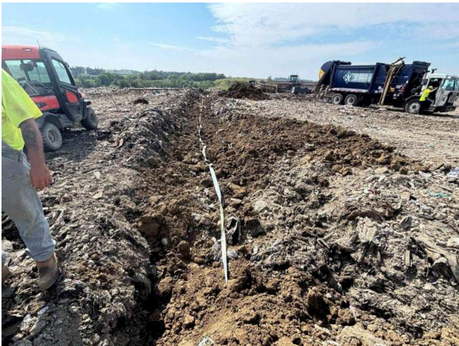
Photo 6: Clean soil and caution tape are placed in HEW – 9.
