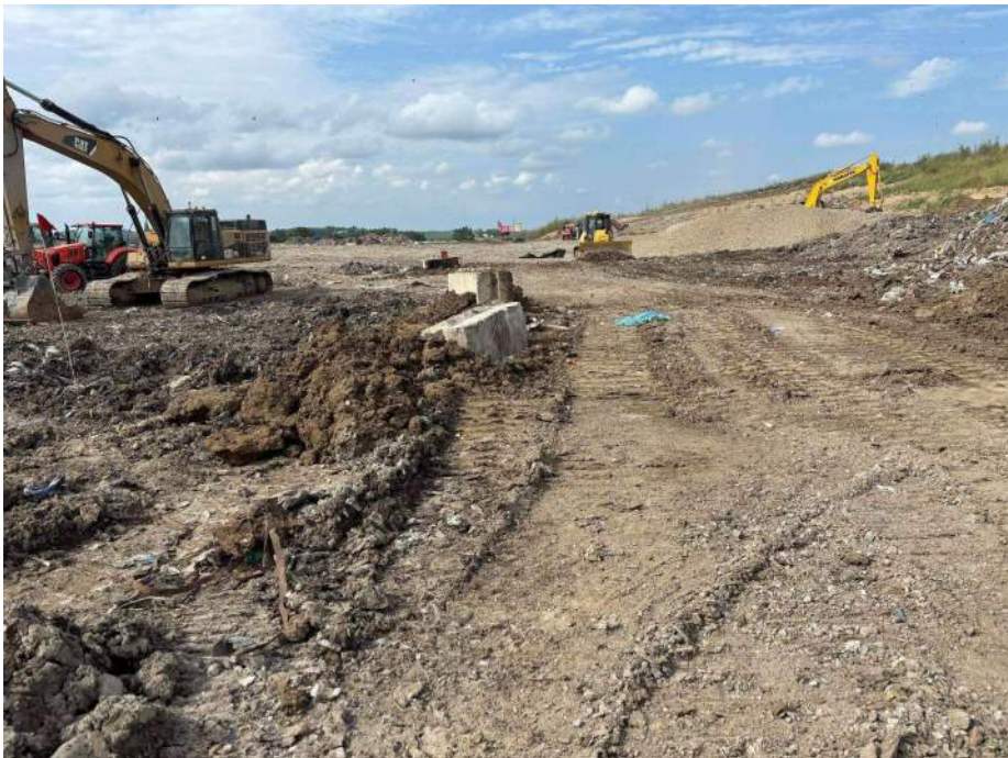
Photo 8: The southern line and HEW – 9 are compacted to grade, and open ends are barricaded.
