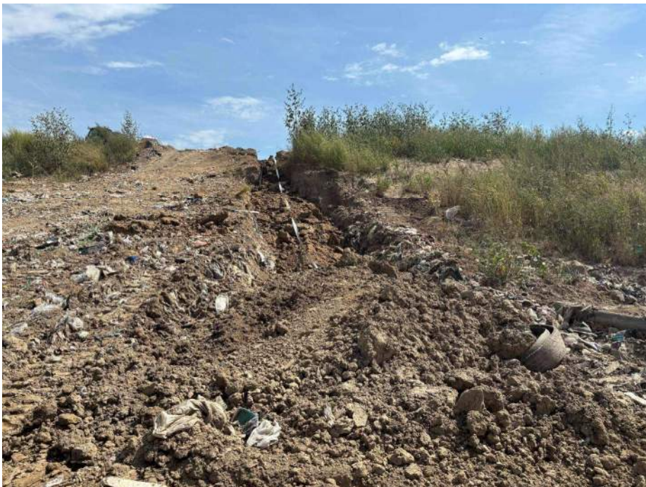
Photo 6: The southern line between the road crossing and active face with the caution tape being sandwiched between clean topsoil layers.
