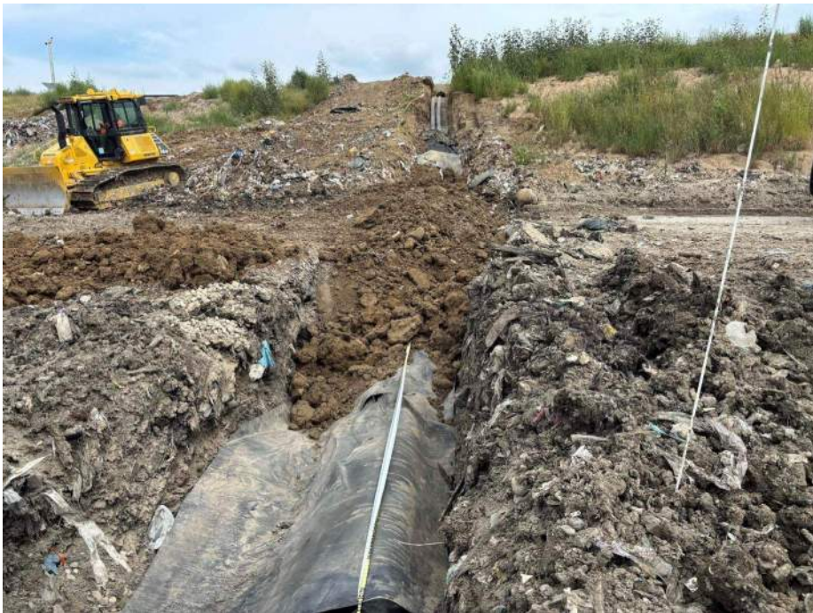
Photo 6: On the southern line geomembrane, clean soil, caution tape, and more clean soil is placed to grade.
