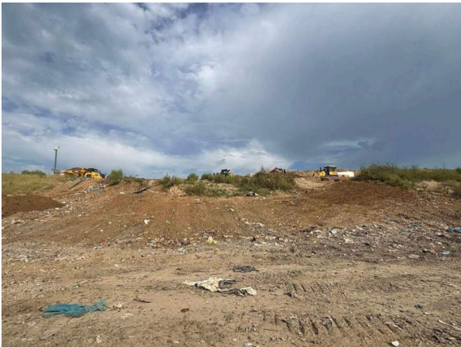
Photo 14: Final grading documented for HEW – 9 and the southern line between the road crossing and the active face.
