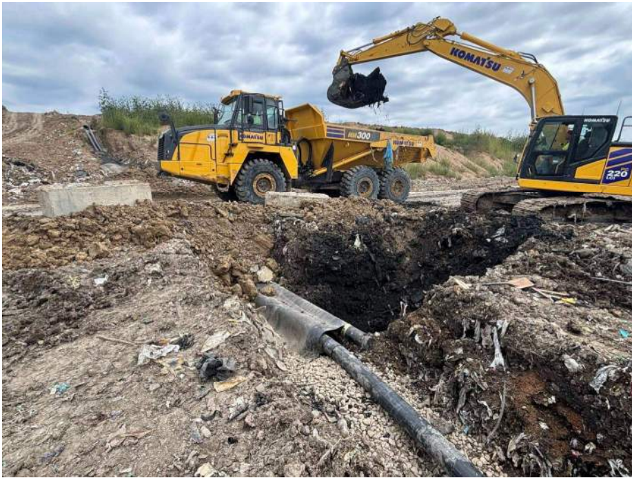
Photo 7: Digging the gravel drain window for HEW – 11.
