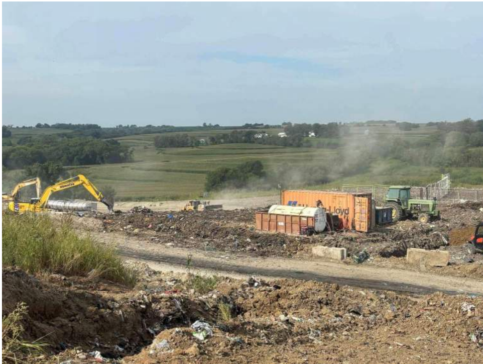
Photo 3: HEW – 11 continues to be trenched.
