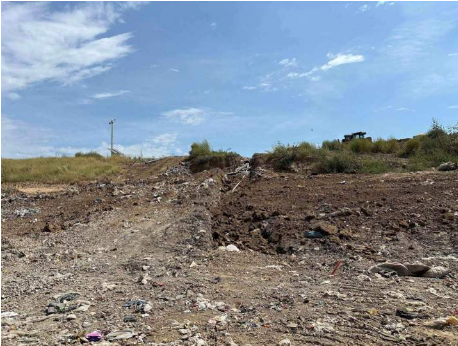
Photo 5: At HEW – 9 caution tape is placed, and clean topsoil is placed to begin final grading.
