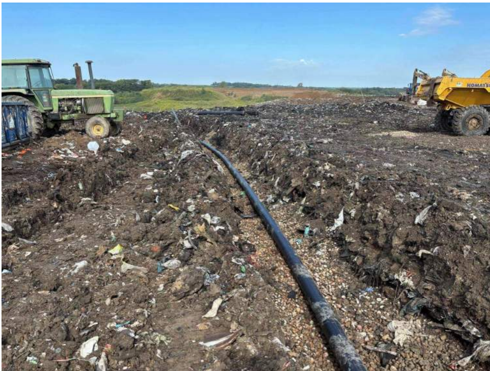
Photo 2: Noncalcareous rock and the 8" perforated pipe placed in HEW – 10.
