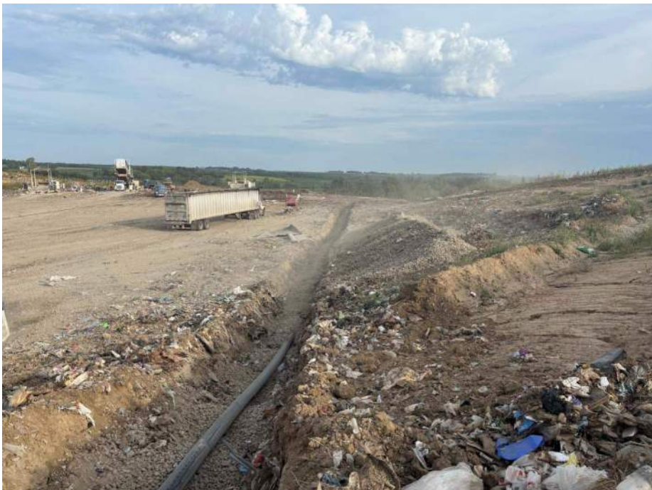
Photo 2: A layer of noncalcareous rock sandwiches the 8" perforated pipe.
