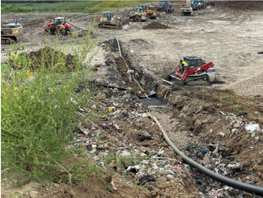
Photo 7: All the same layers are placed on HEW – 9.
