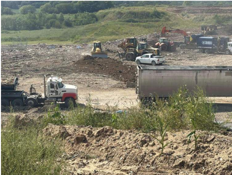
Photo 3: HEW – 9 is backfilled with clean soil to grade.
