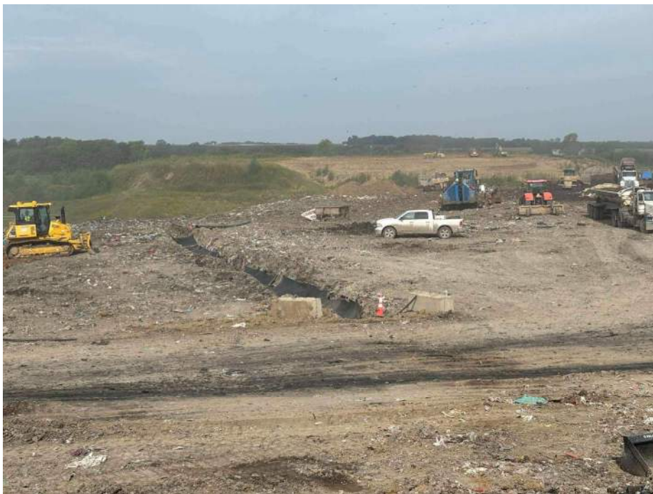
Photo 4: Geotextile and geomembrane are placed at HEW – 9.
