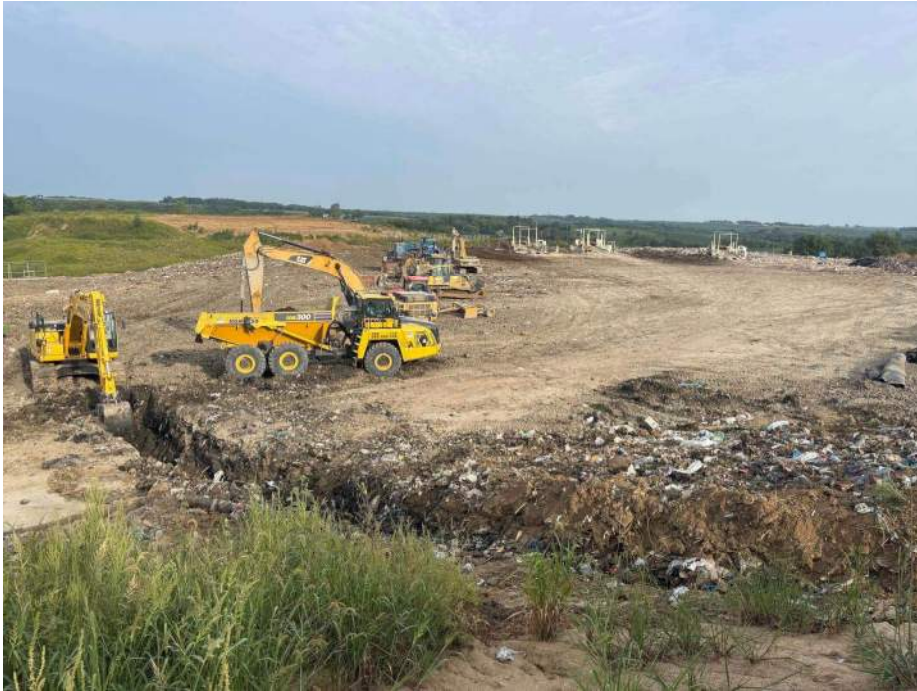
Photo 1: Trenching the southern line until the branch off point
