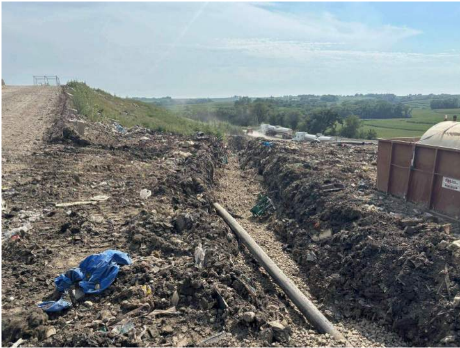
Photo 5: Noncalcareous rock is placed in HEW – 11.
