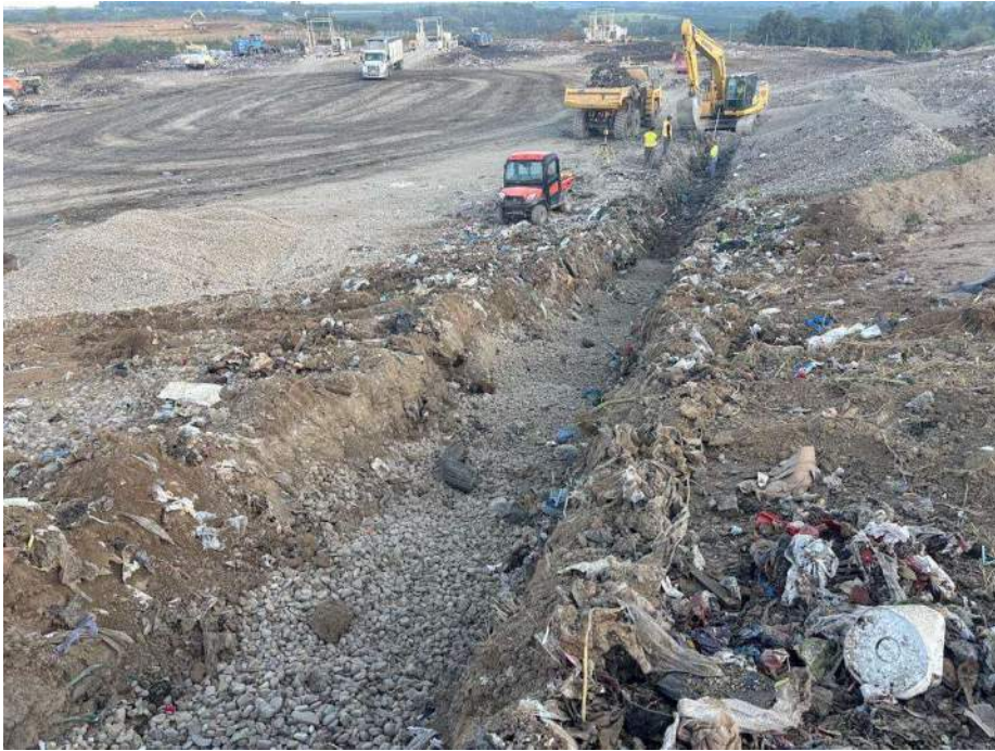
Photo 1: Excavator digs HEW – 8, while the dozer delivers noncalcareous gravel.
