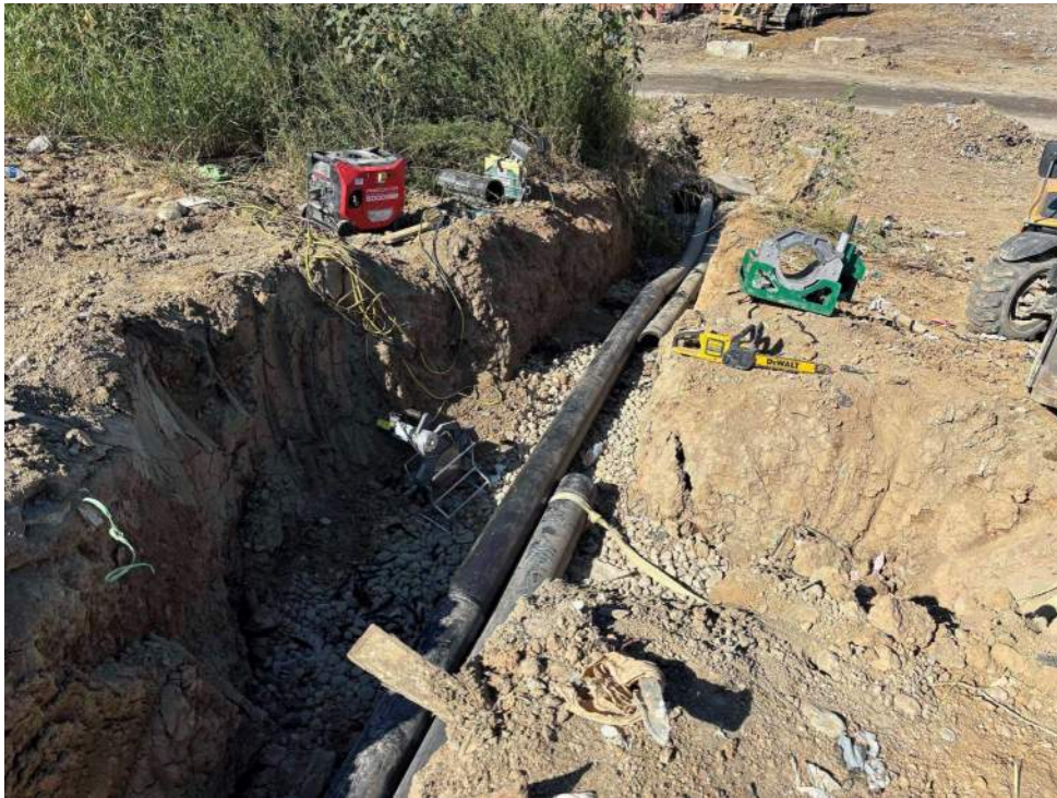
Photo 1: Tie-in on the southern line west of the road crossing. Gravel drain window is located at the bulge point of the trench. HEW – 10: solid to perforated, HEW – 11: solid to solid
