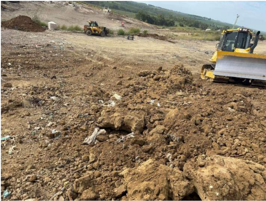
Photo 13: Final grading documented west of GEW – 53R going towards the southern road crossing.
