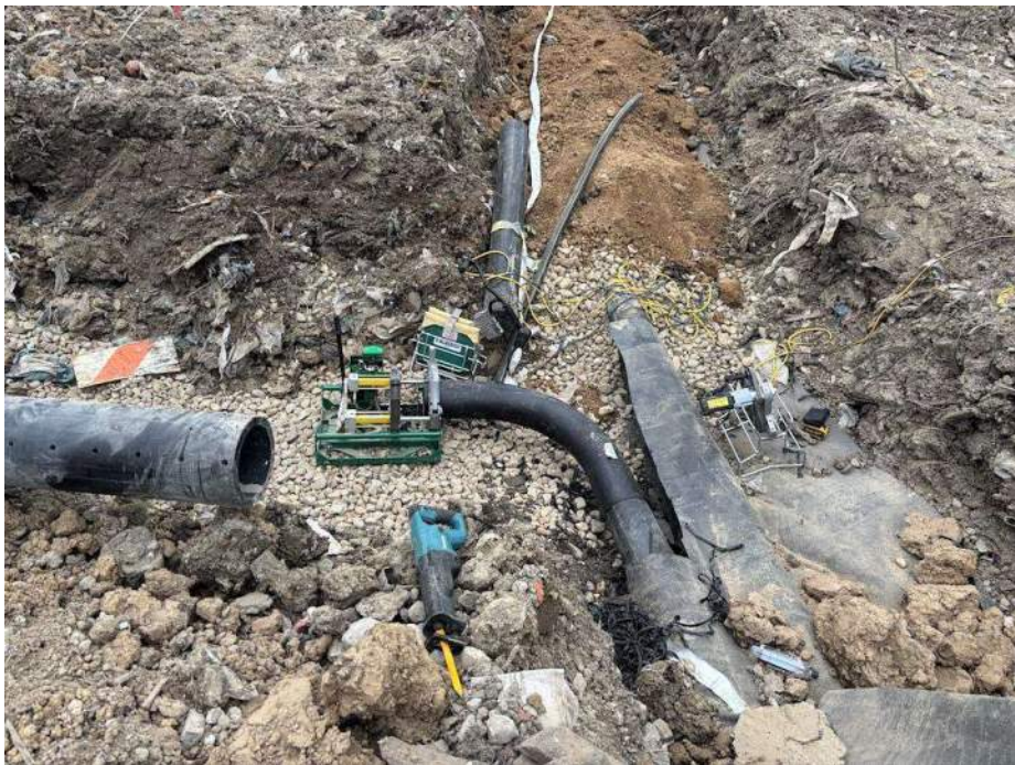
Photo 1: Elbow sweep and some 8" perforated pipe is welded for HEW – 11.
