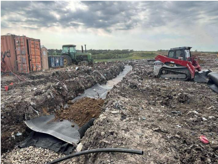
Photo 6: HEW – 10 with noncalcareous rock, geotextile, geomembrane, and soil layers shown.
