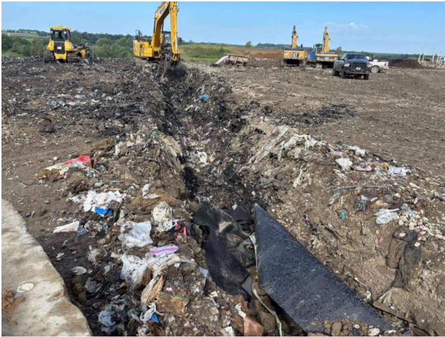
Photo 3: Trenching for HEW – 9.
