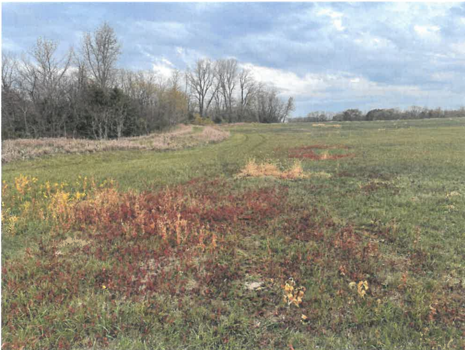
Photo 6: View of fixed berm west of Pizometer 2
