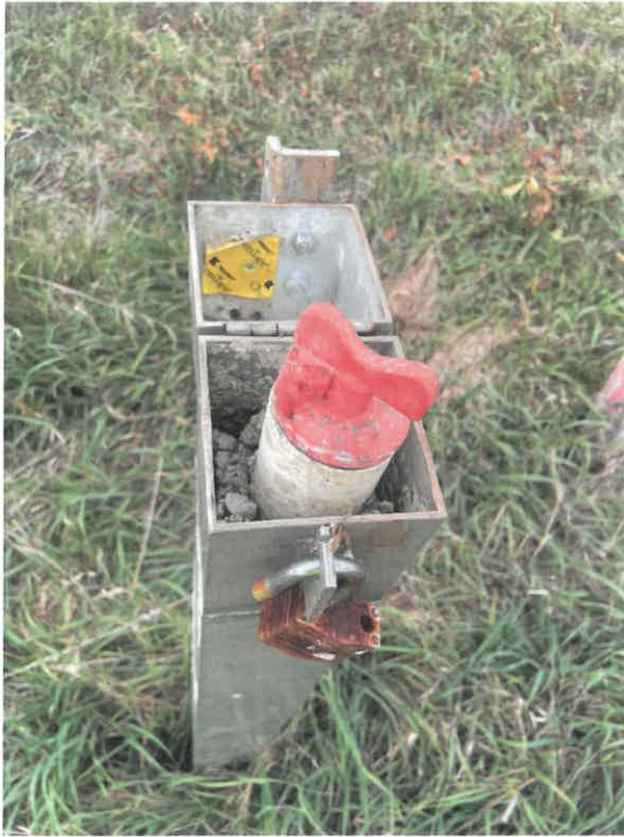
Photo 1: Close up view of Monitoring Well (P3)
