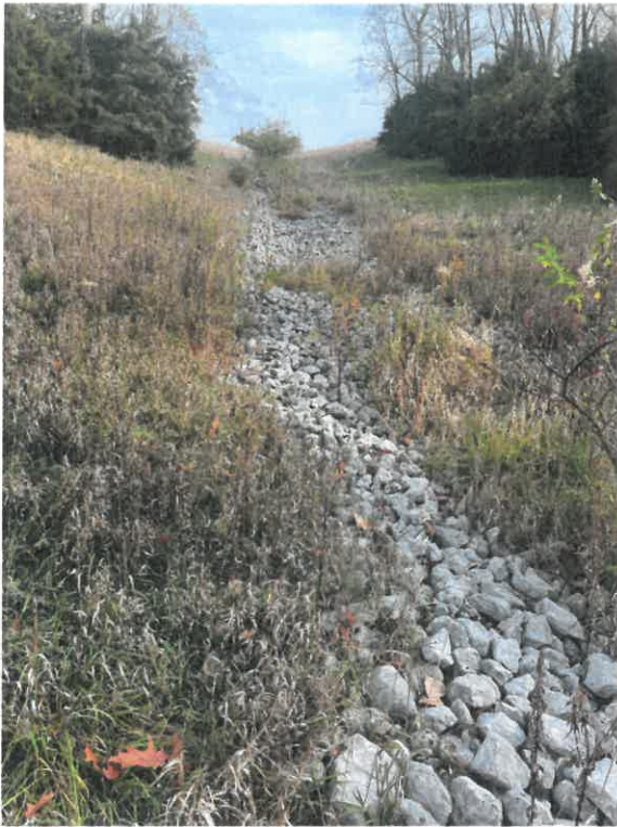
Photo 3: View of the gully with intact rip rap upgradient of MW4
