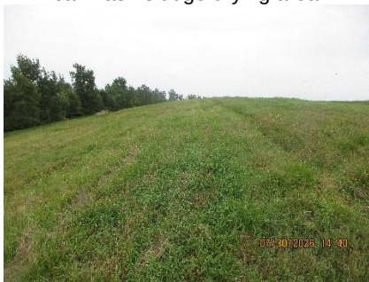
north slope, north filled area
