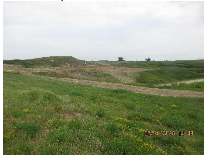
west side, north filled area
