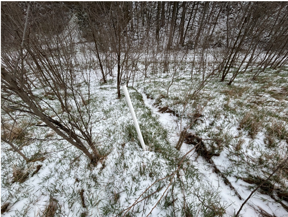
Photo 2: Woody vegetation and Erosion rill on the east sideslope.
