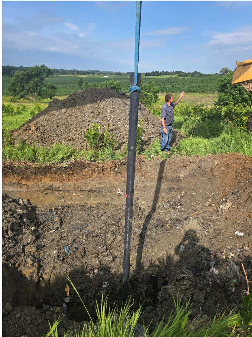
Photo 3: Gas collection pipe installation.
