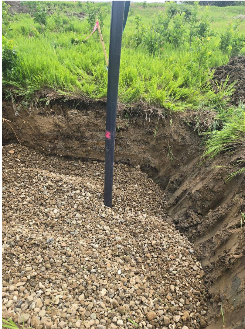
Photo 5: Installation of clean granular backfill around piping.
