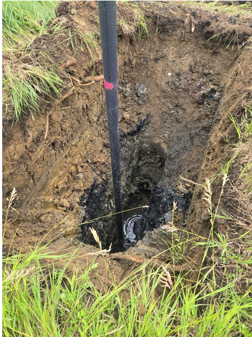
Photo 4: Gas collection pipe installation.
