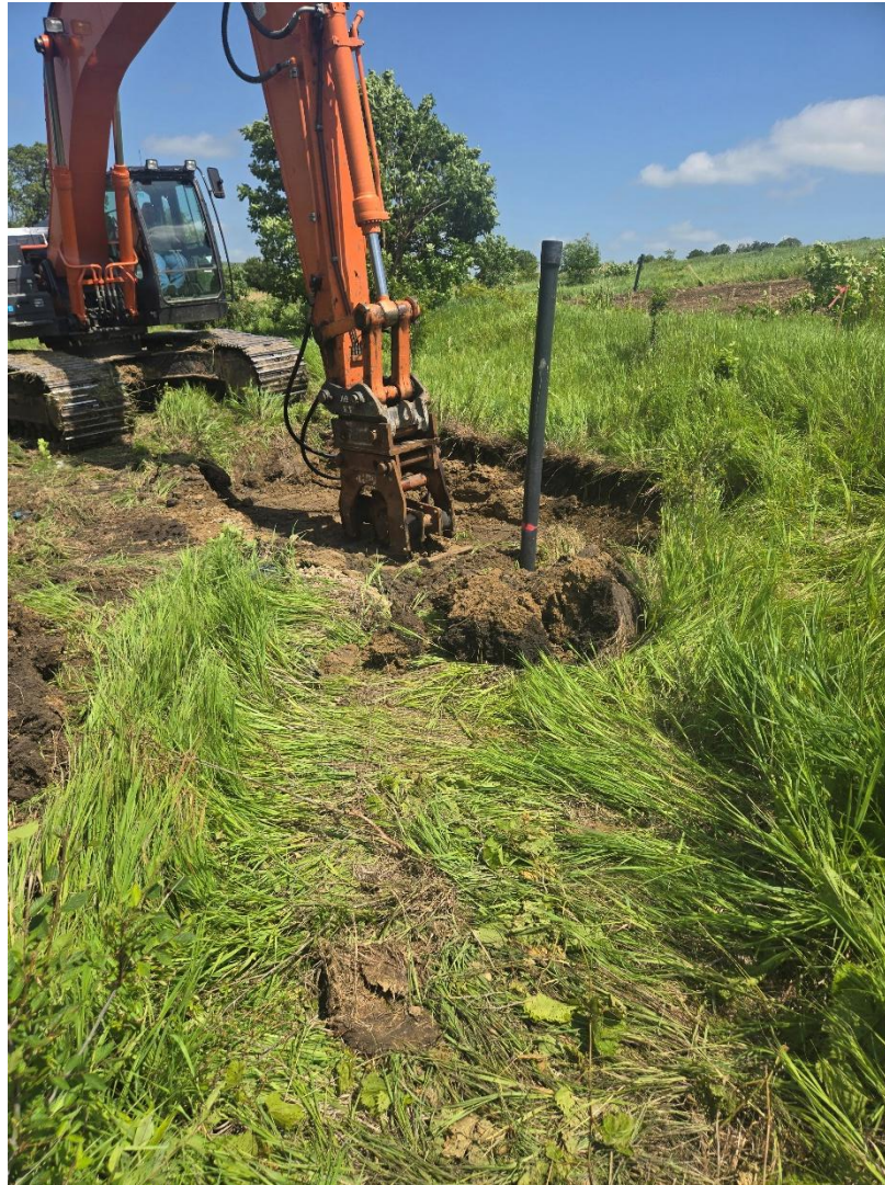
Photo 6: Compacting soil backfill.
