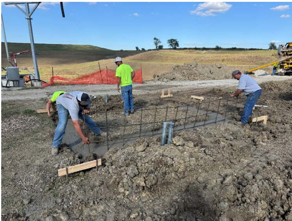
Photo 12: Rebar caging installation in footing for treatment building.
