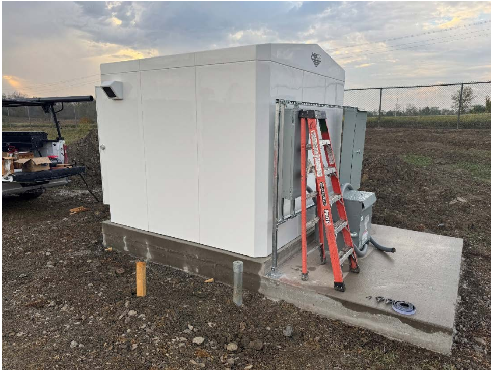
Photo 25: Installation of Treatment Building.
