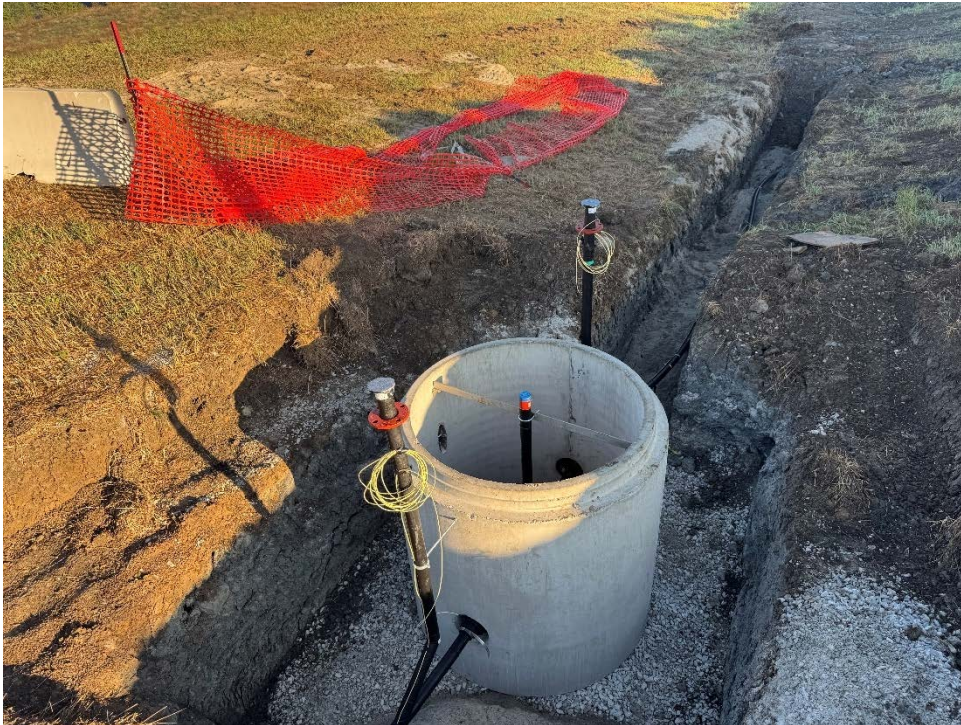
Photo 9: Air/vacuum release manhole and cleanout installation.
