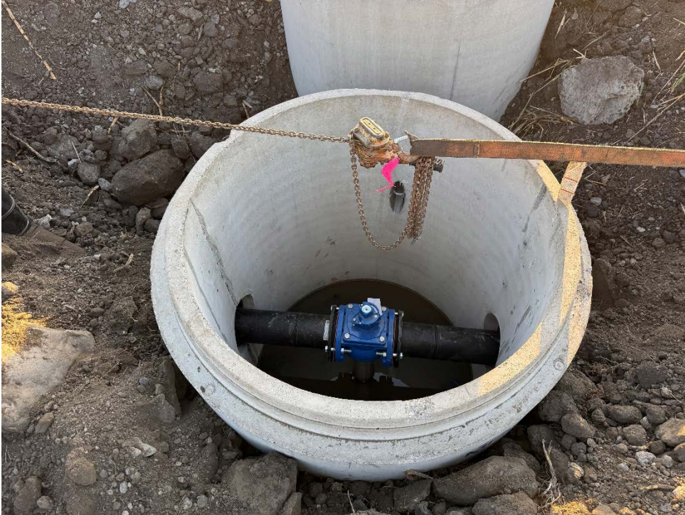
Photo 15: Leachate valve manhole, LVMH-1 manhole installation north of sedimentation pond.
