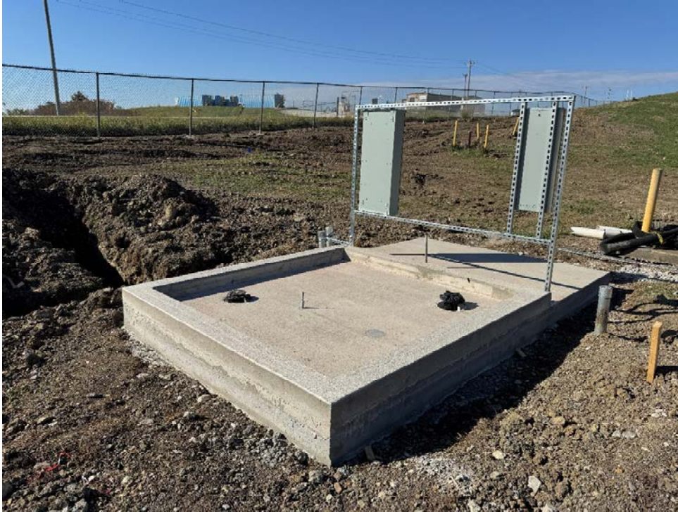
Photo 23: Completed foundation for treatment building.
