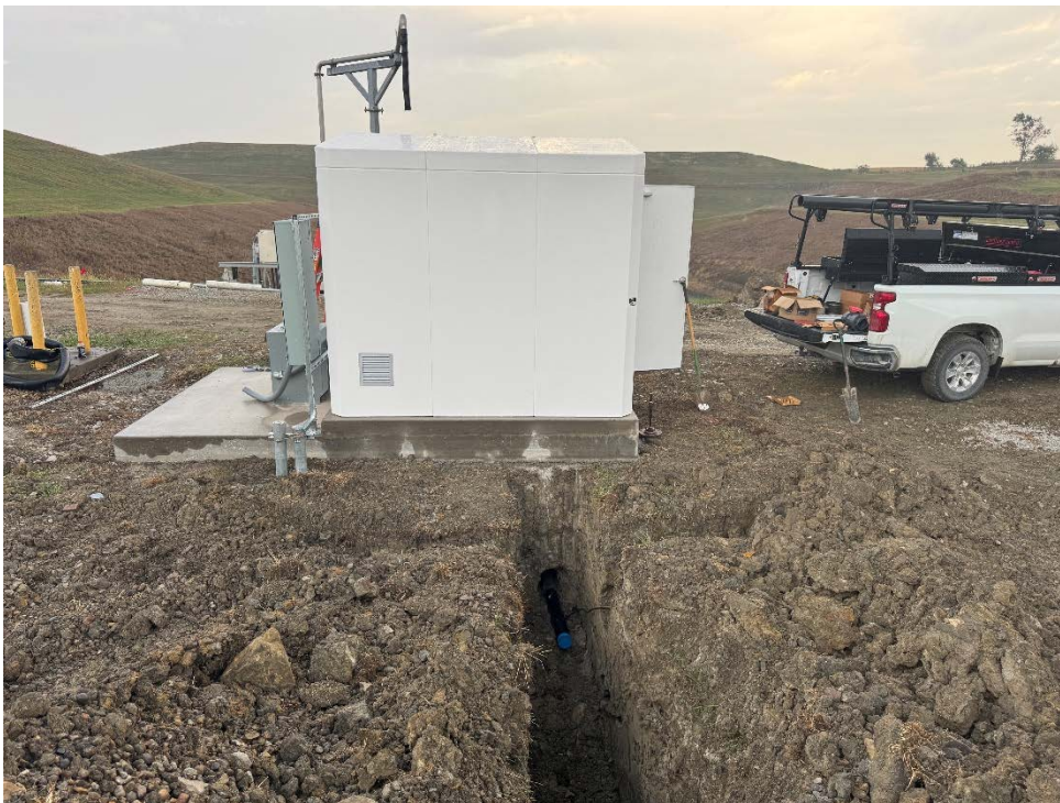
Photo 26: Installation of Treatment Building.
