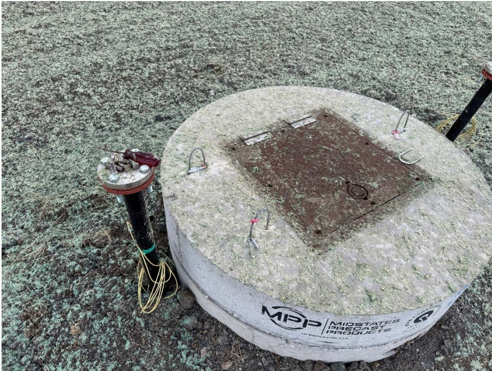
Photo 37: Completed air/vacuum release manhole.
