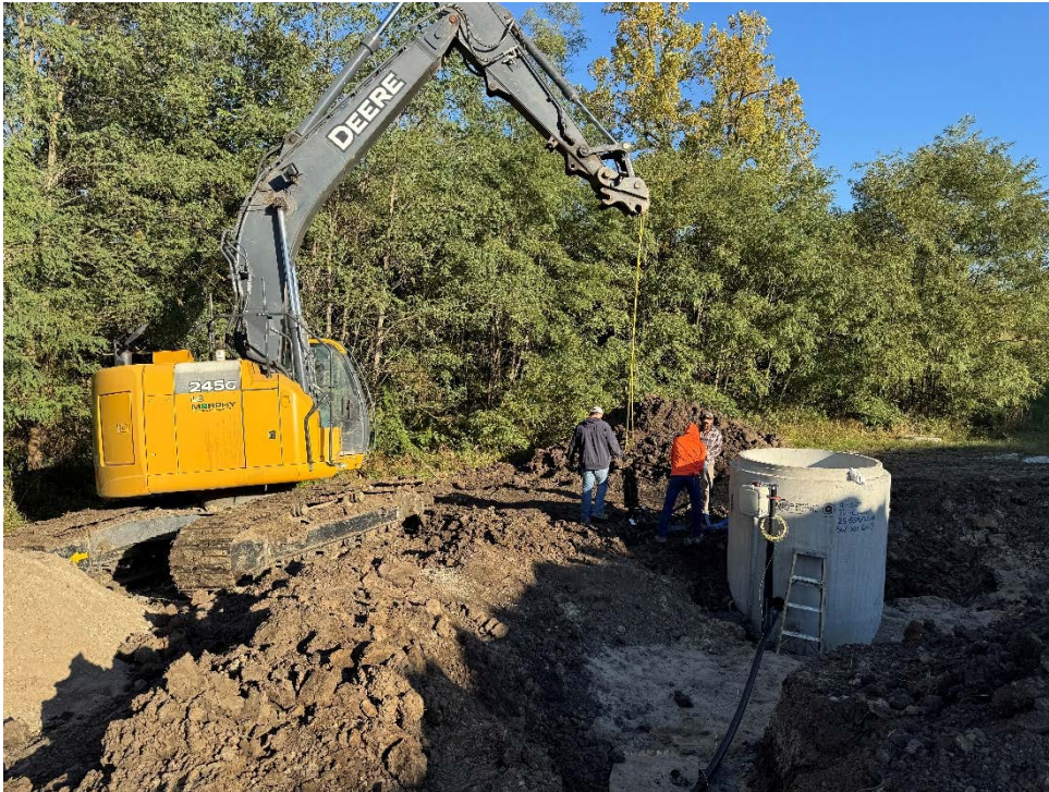
Photo 19: North Lift Station, LS-1 installation.
