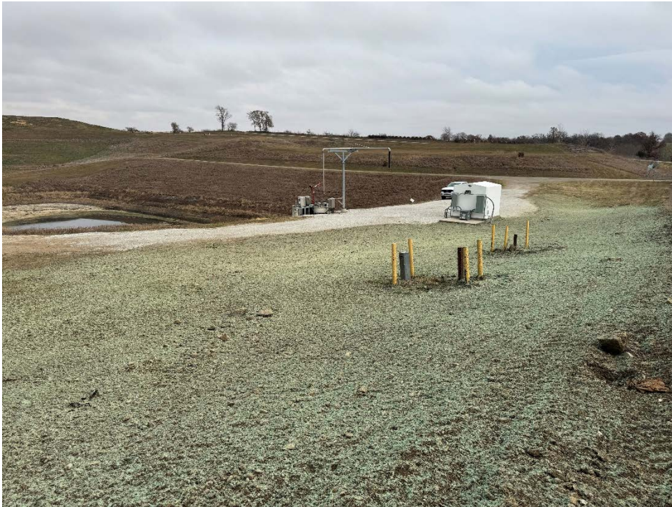
Photo 31: Final grading and seeding near Treatment Building.
