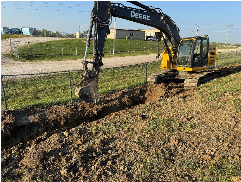
Photo 1: Force main trench along north side of 130 th Street..
