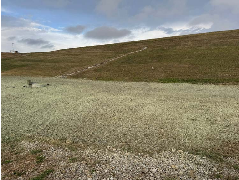
Photo 33: Final grading and seeding around valve manholes area.
