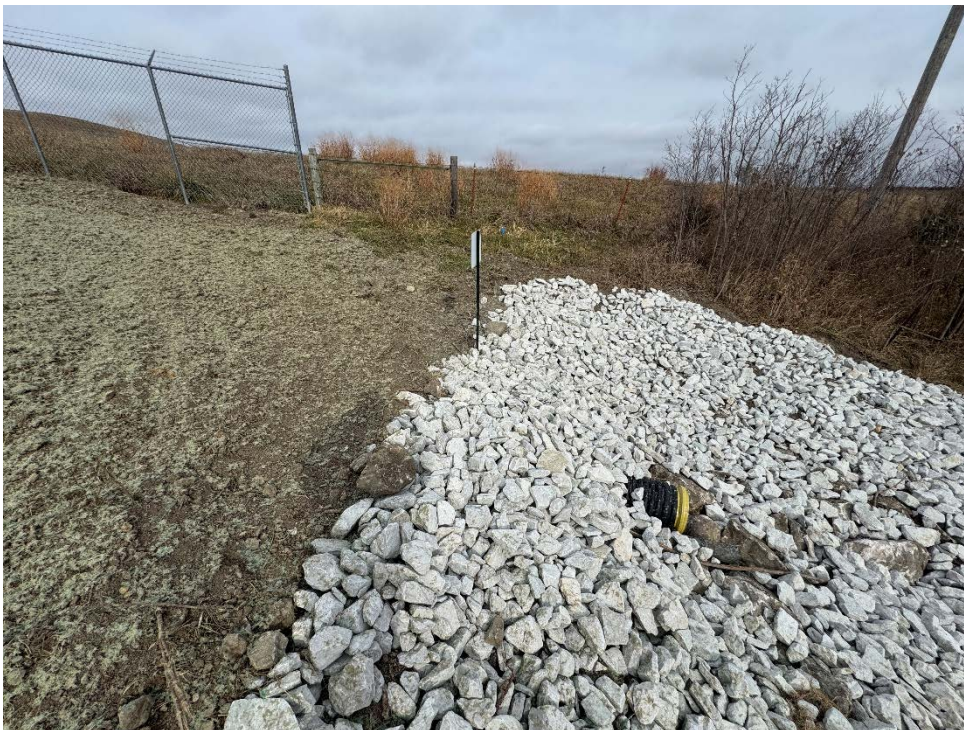
Photo 38: Discharge area final grading and seeding.
