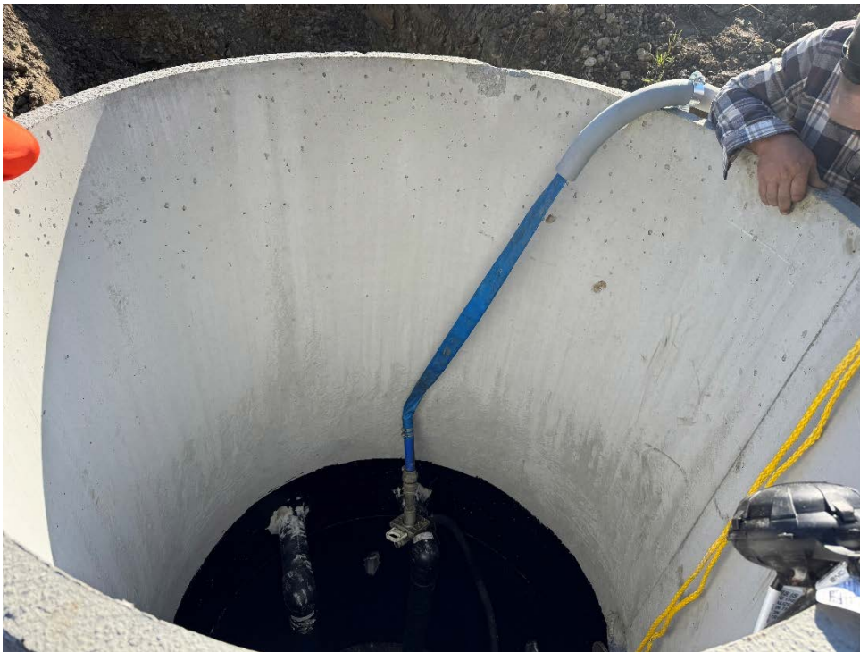
Photo 20: Pump installation in North Lift Station, LS-1.
