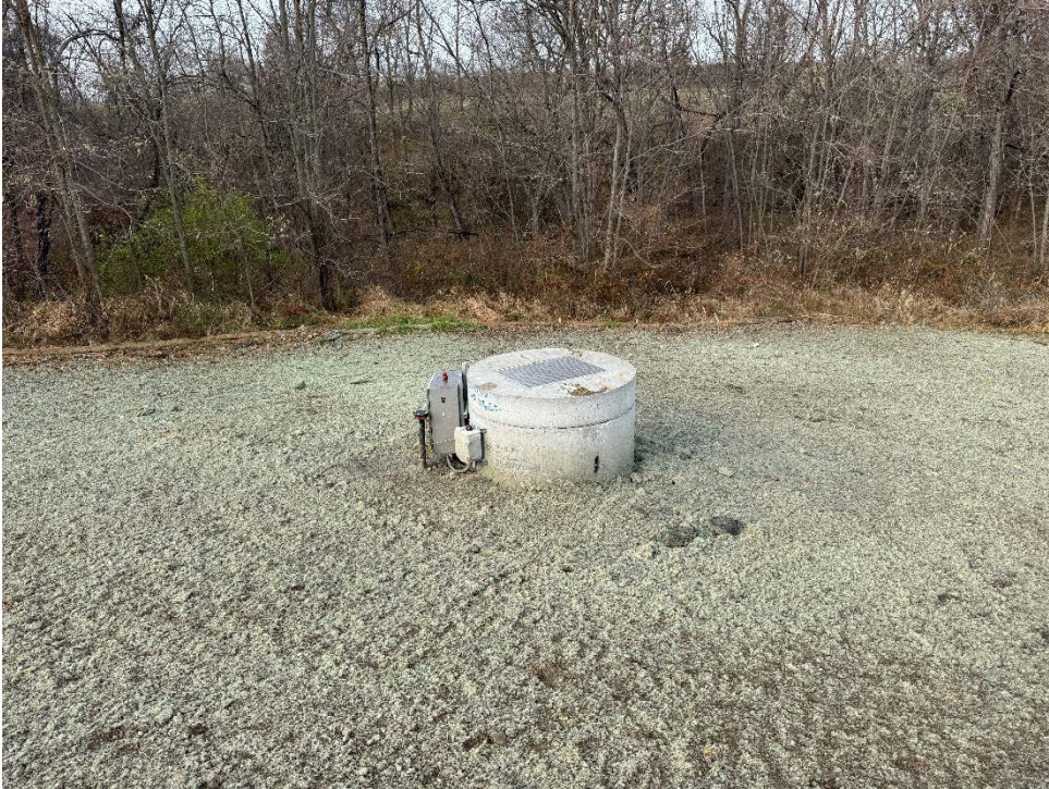
Photo 35: North Lift Station, LS-1 final grading and restoration.
