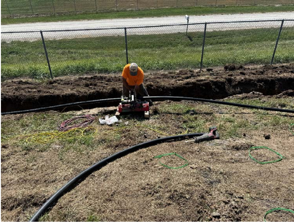
Photo 3: Fusion welding force main pipe.
