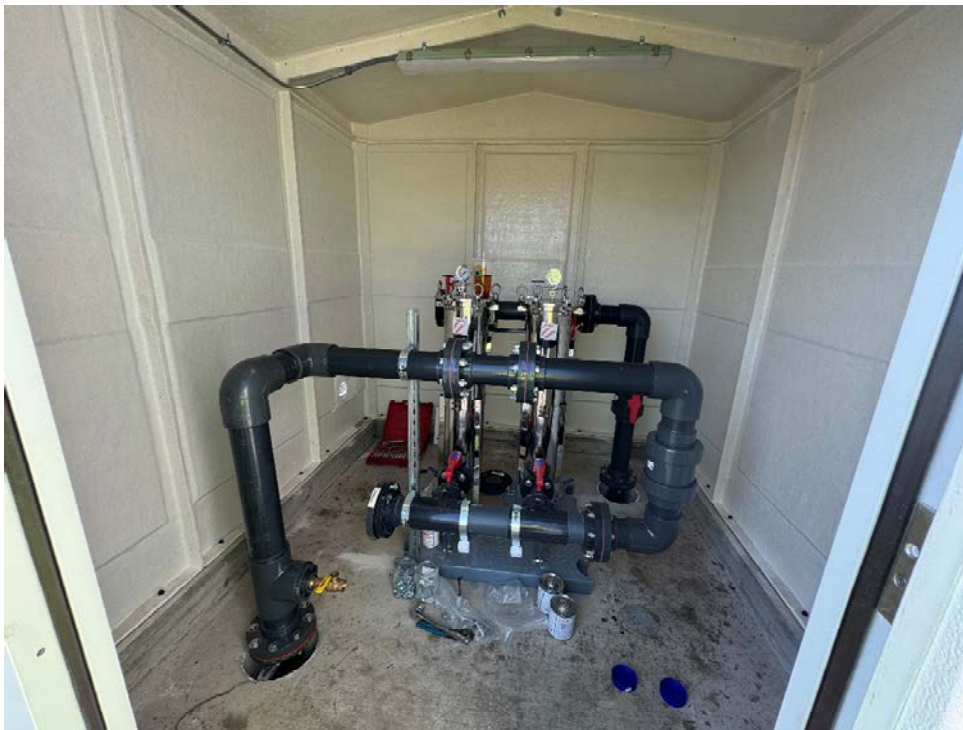
Photo 28: Piping installation in Treatment Building.
