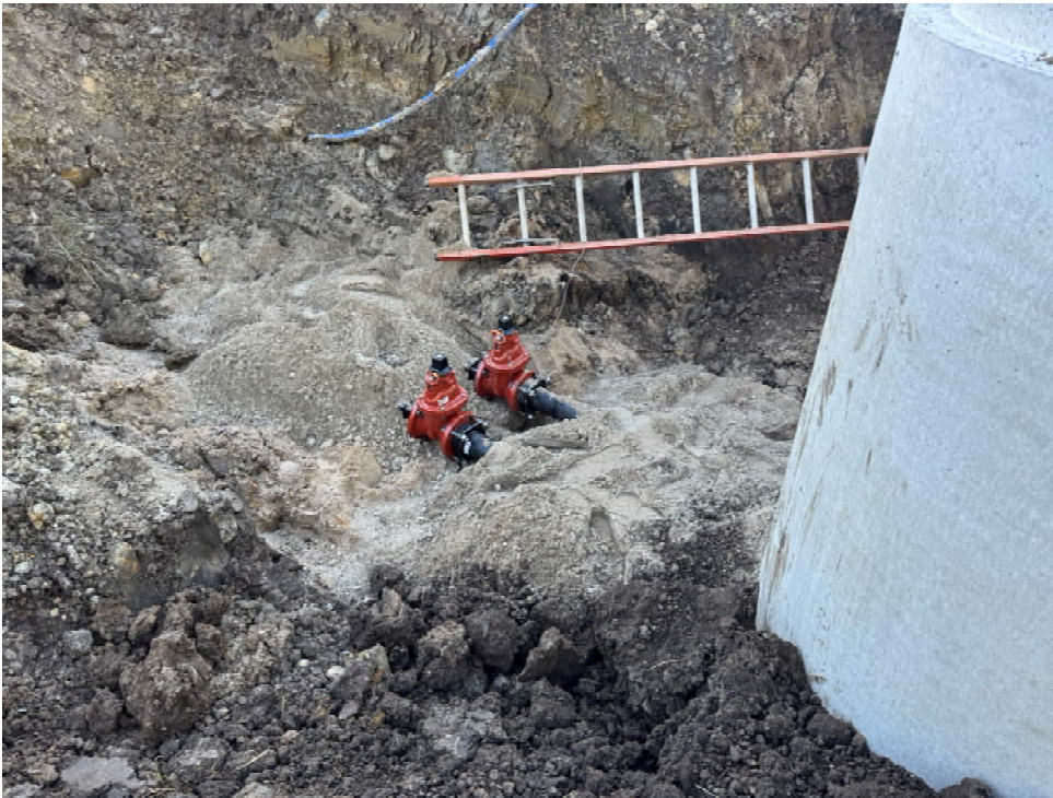
Photo 24: Installation of gate valves on inlet piping to LS-1.
