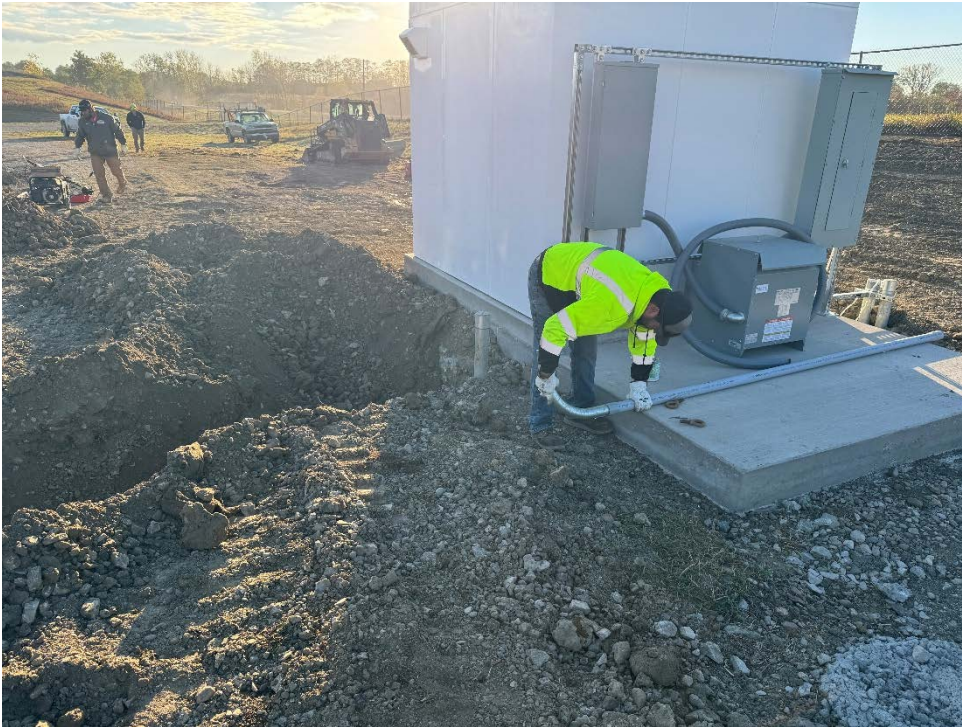
Photo 29: Installation of electrical to the Treatment Building
