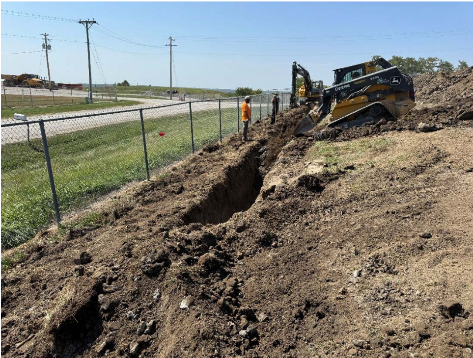
Photo 4: Force main trench backfilling and grading.
