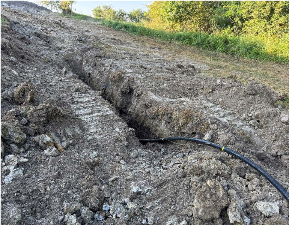
Photo 6: Force main pipe installation west of landfill haul road.
