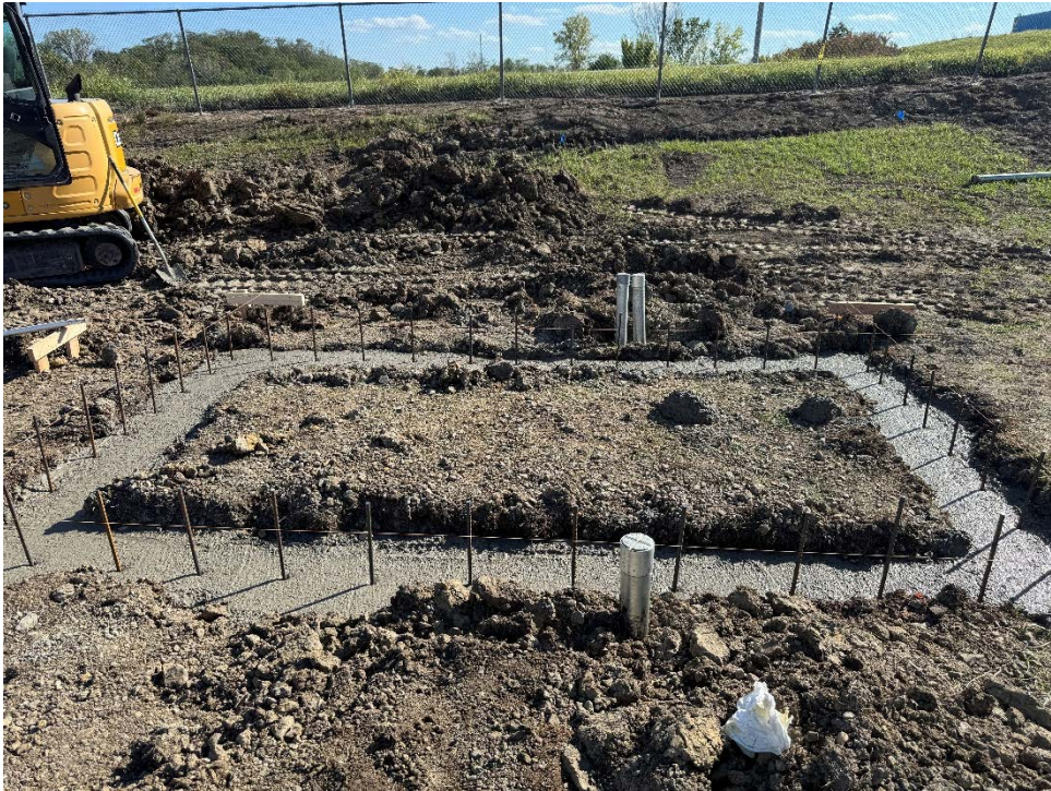
Photo 13: Finished rebar installation treatment building foundation.
