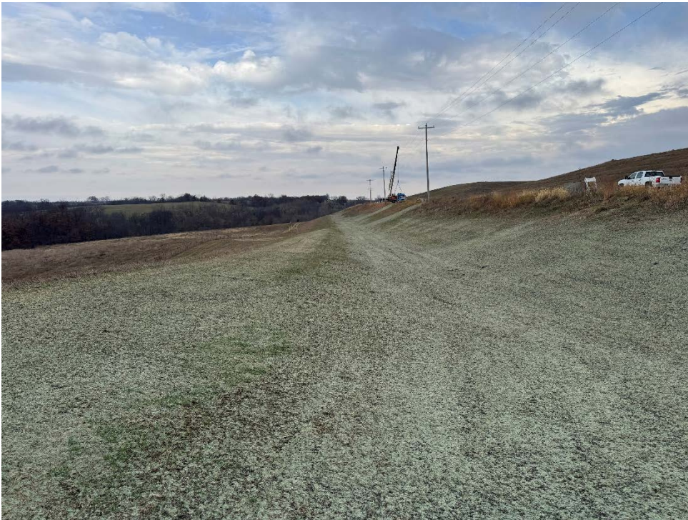
Photo 34: Final grading and seeding along west force main route.
