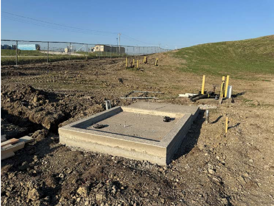
Photo 17: Concrete pad and curbs installed for treatment building foundation.
