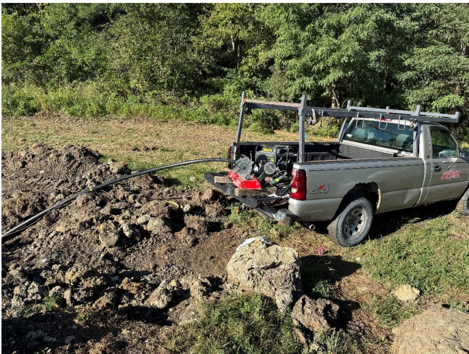
Photo 10: Force main fusion welding in the north section.
