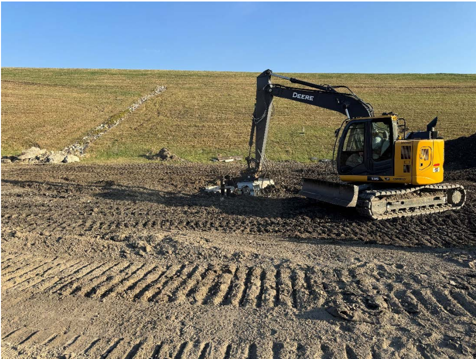
Photo 16: Valve manhole area backfilling and compacting.
