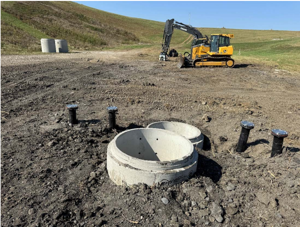
Photo 18: Valve manhole installation.
