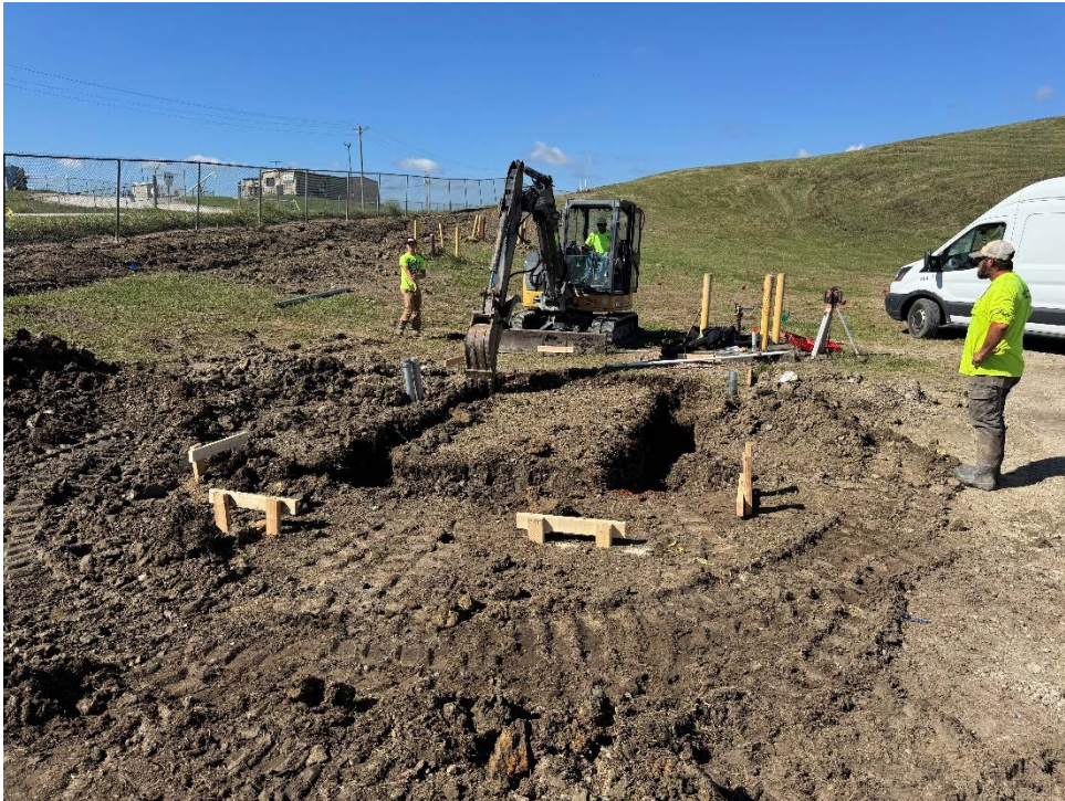
Photo 11: Foundation excavation for the Filter Bag Building.
