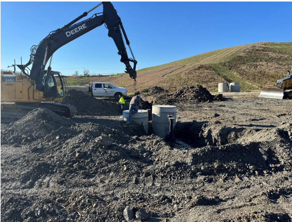
Photo 30: Completion of valve manholes, VMH-1 & LVMH-1.
