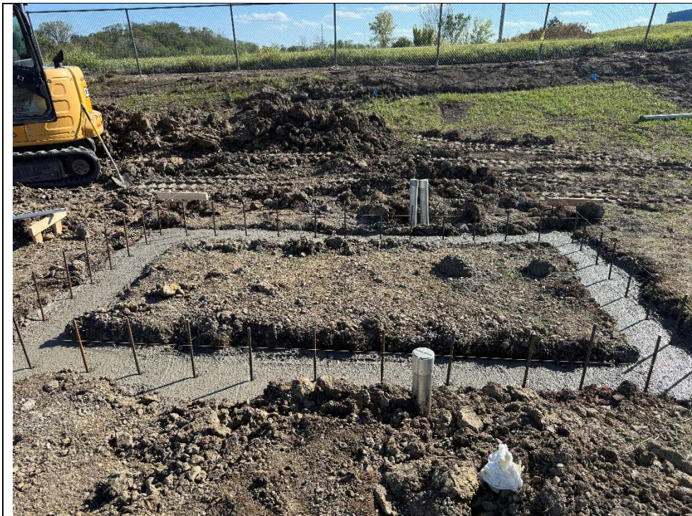
Photo 14: Finished rebar installation treatment building foundation.
