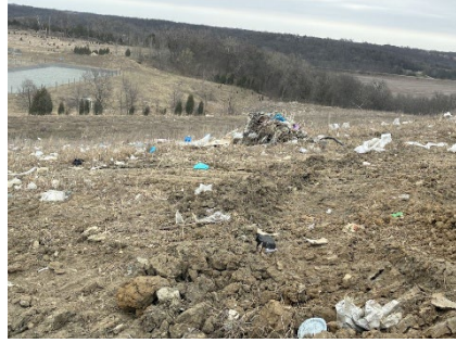
Northeast slope of working face in western area, additional cover needed.
