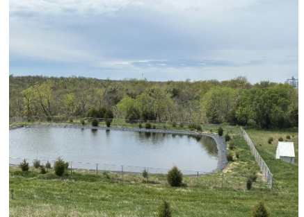
Western leachate lagoon
