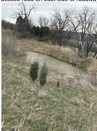
North stormwater basin
