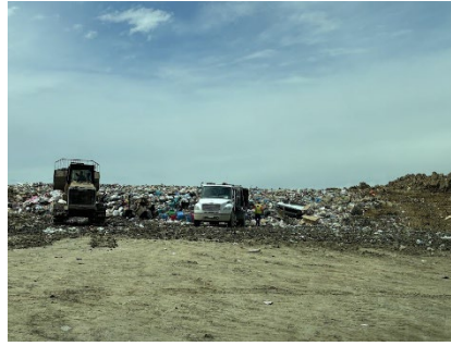
Active working face in western area
