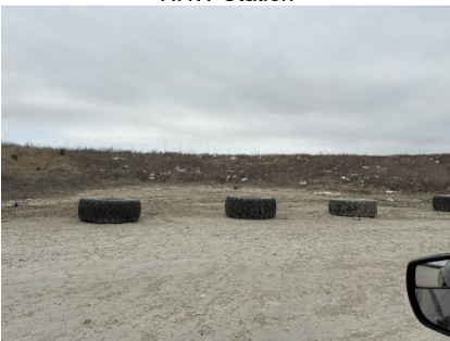
Access barriers along access roadway
