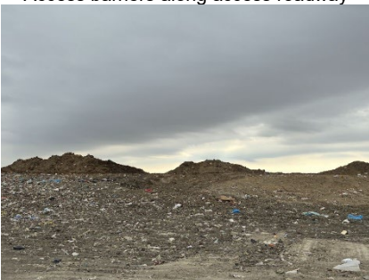
North slope of western area – insufficient cover soil
