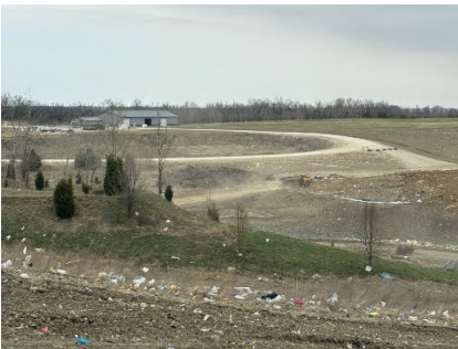
West access road facing east, scale house in background
