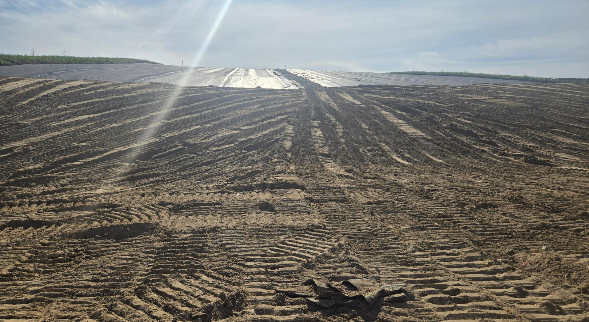
Photo 1: Drainage layer sand coverage area reviewed 05/06/26. Looking east.
