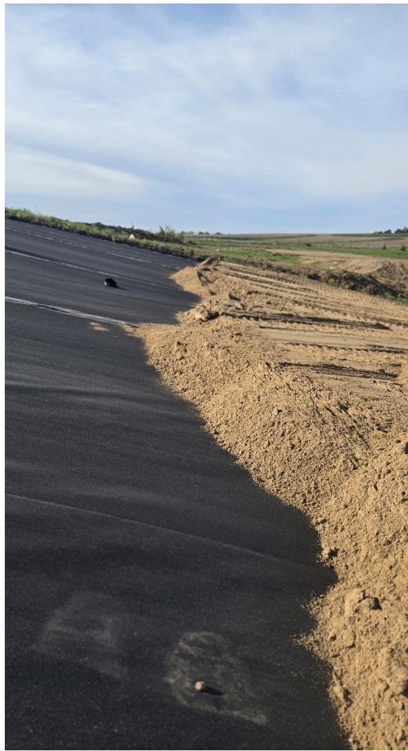
Photo 2: Drainage layer sand coverage area reviewed 05/06/26. Looking south.
