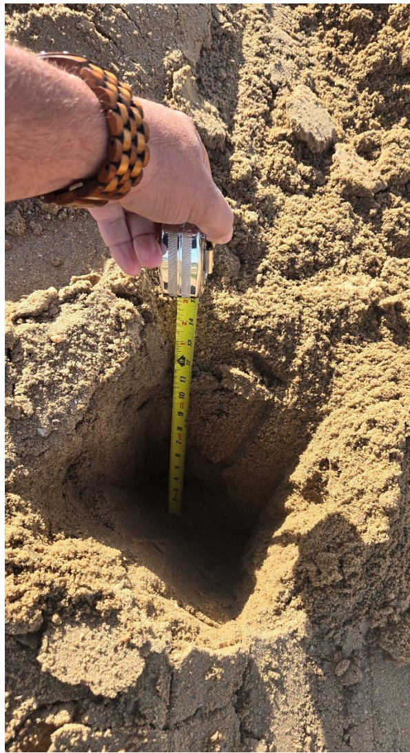
Photo 5: Drainage layer sand measurement 05/06/26.
