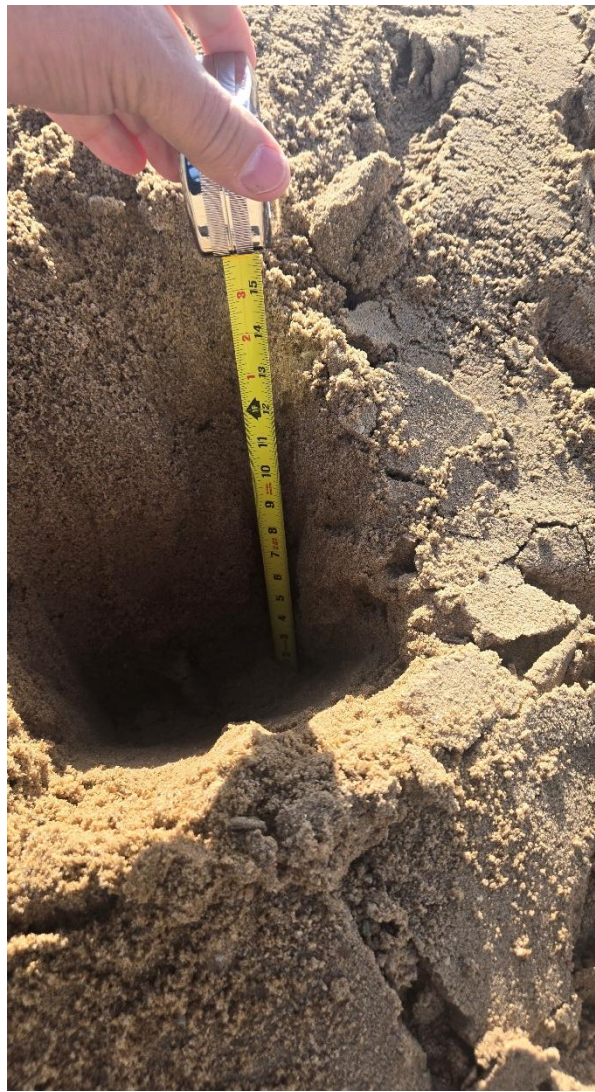
Photo 4: Drainage layer sand measurement 05/06/26.
