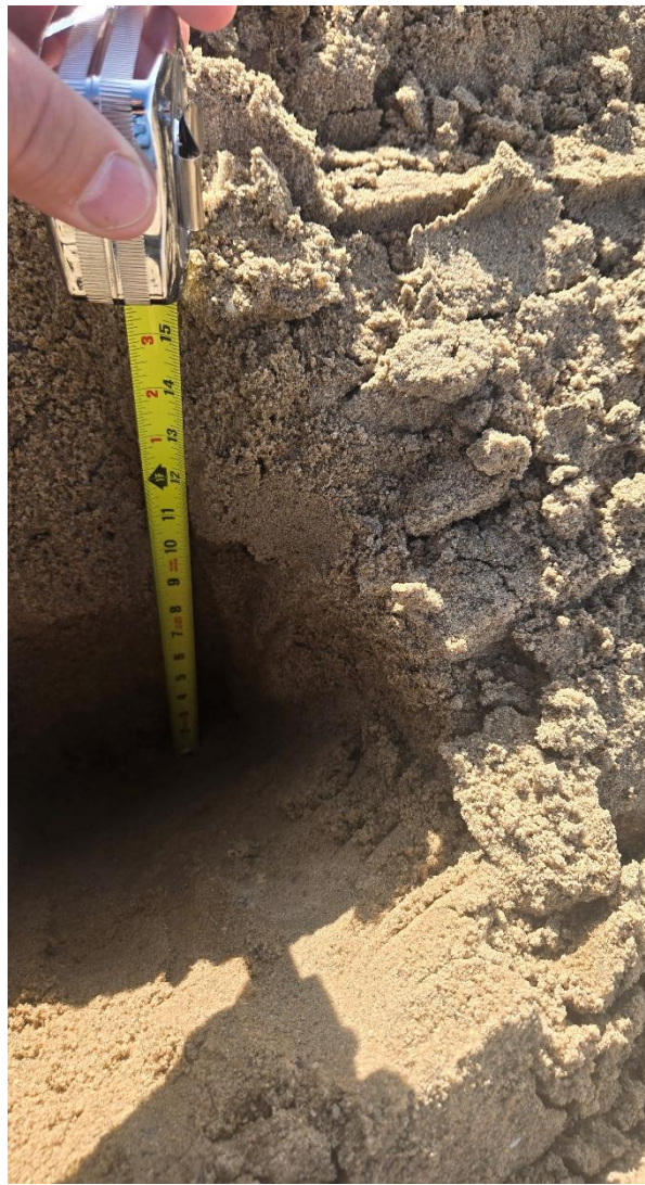
Photo 3: Drainage layer sand measurement 05/06/26.
