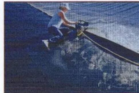
HOT WELDING TWO HDPE LINER SHEETS TOGETHER
