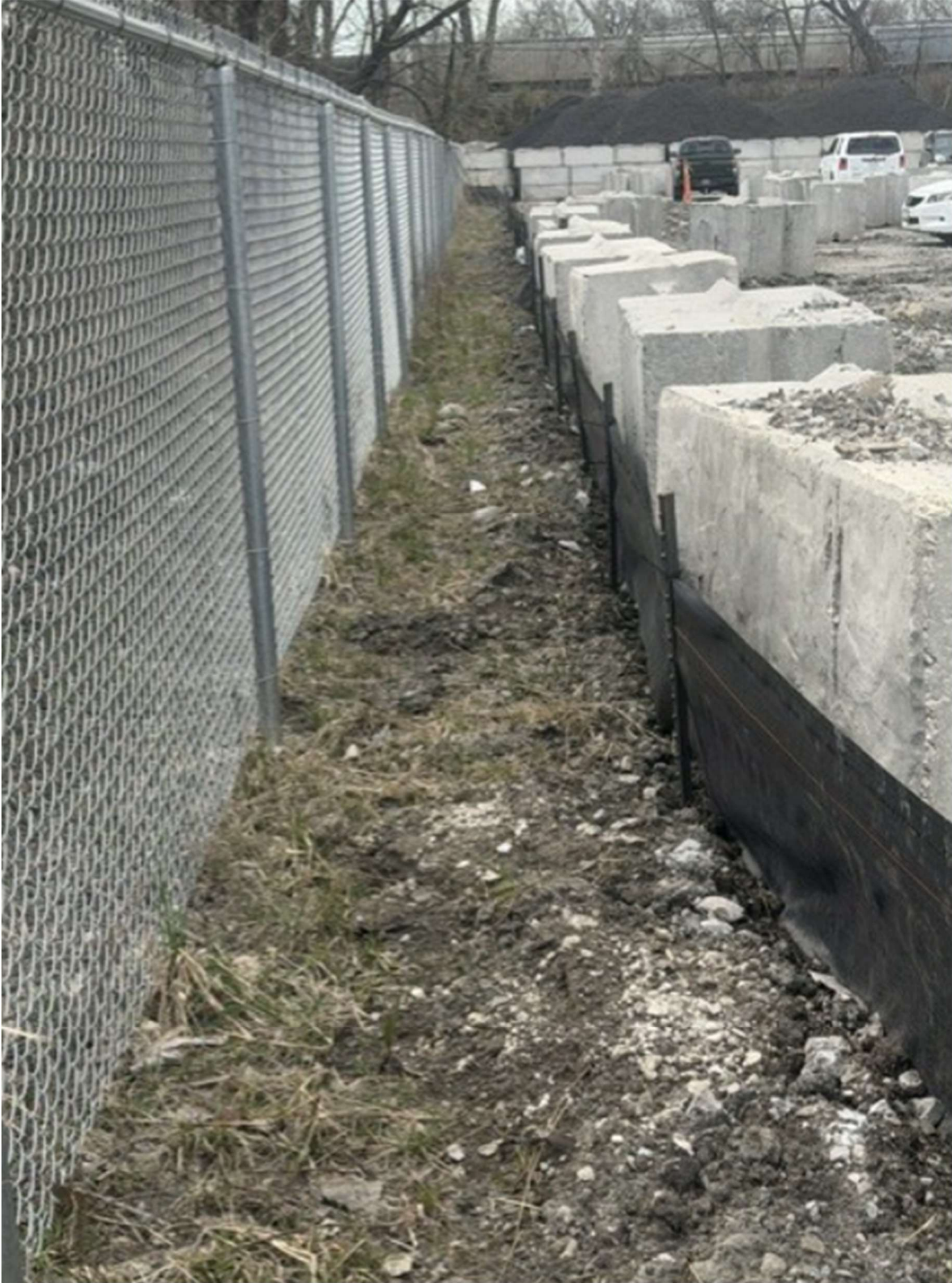
New Silt Fence Installation South Property Line facing West
