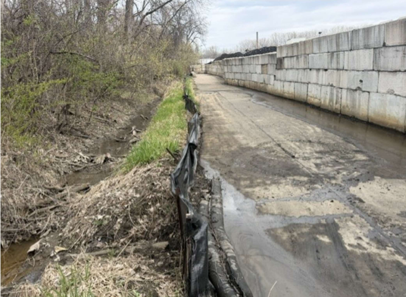
New Silt Fence Installation West Property line facing North
