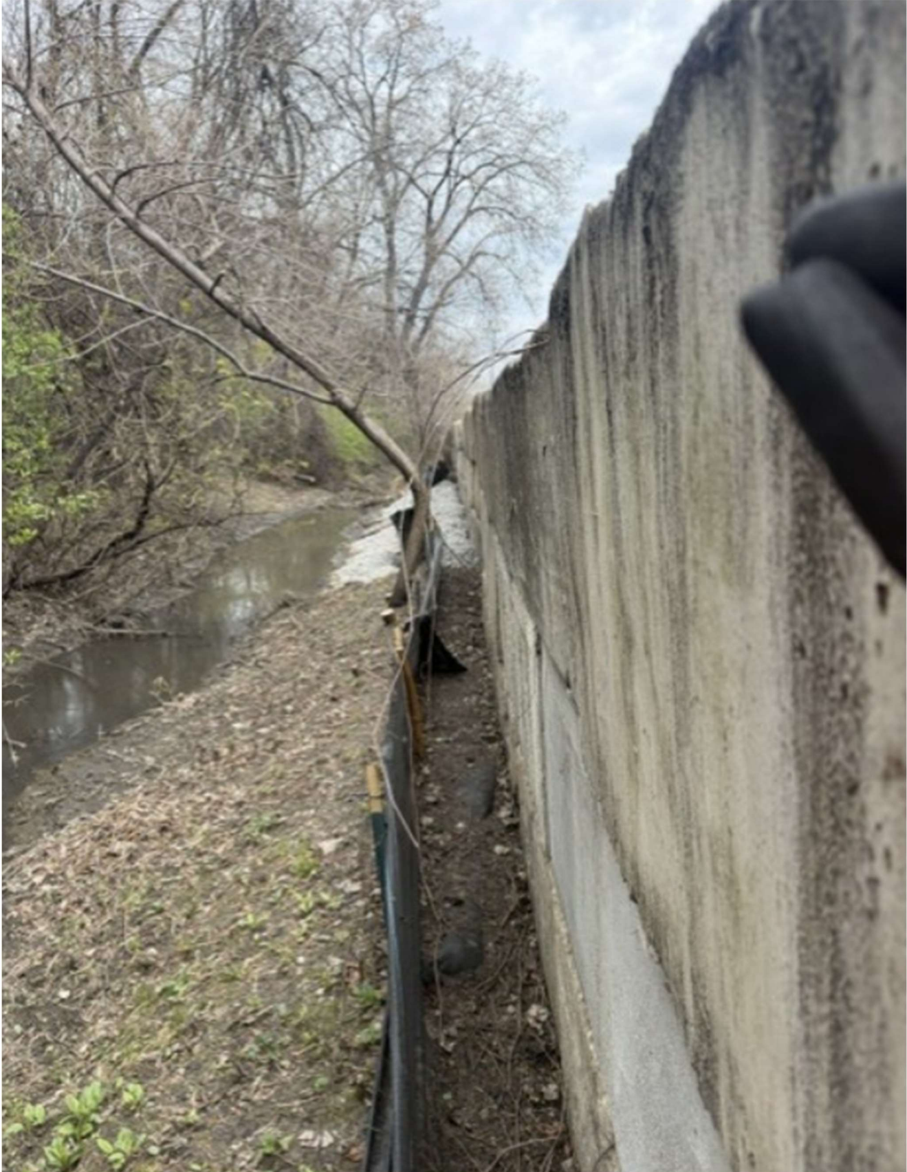
New Silt Fence Installation West property line behind wall facing North
