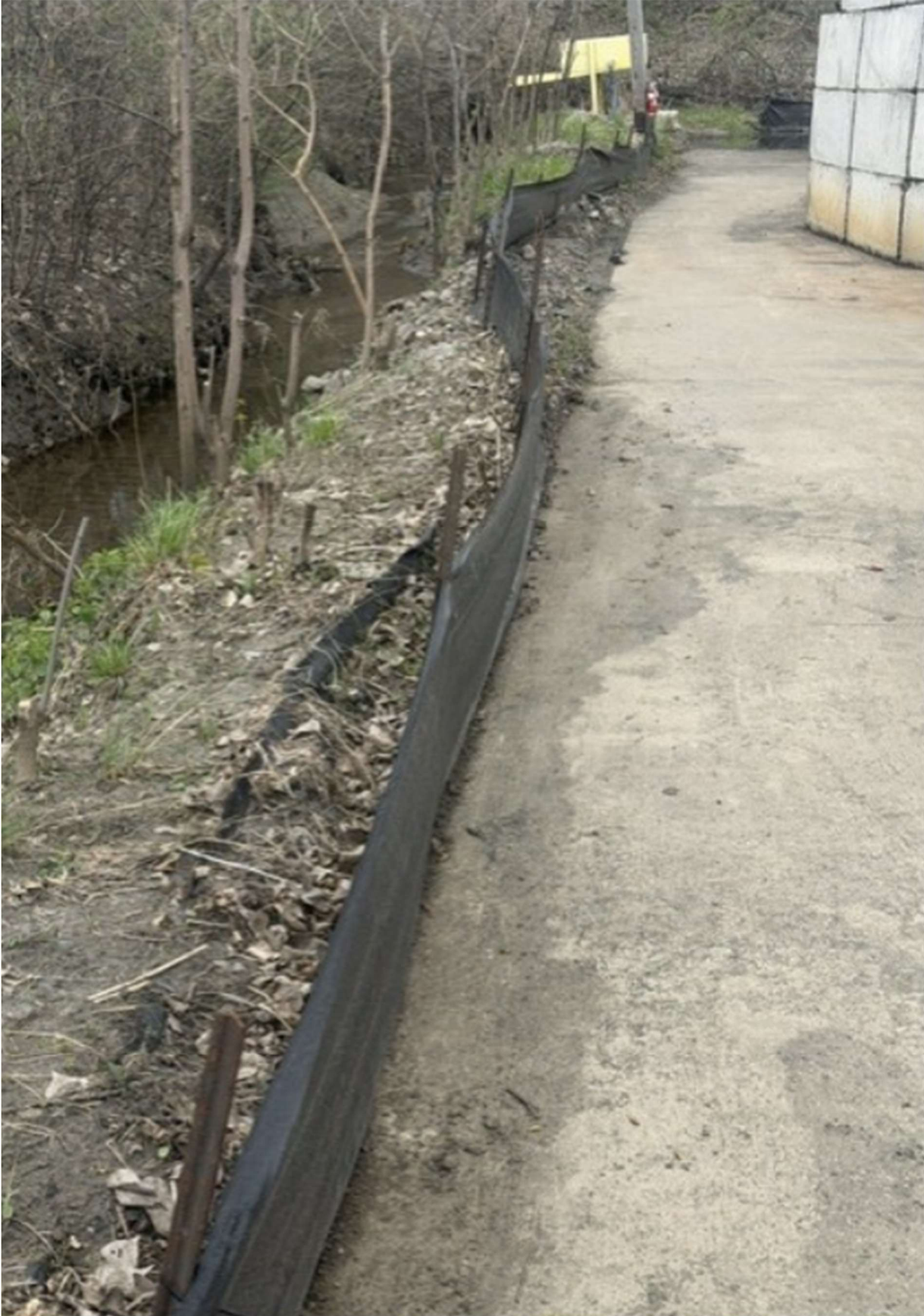
New Silt Fence Installation South Property Line facing West
