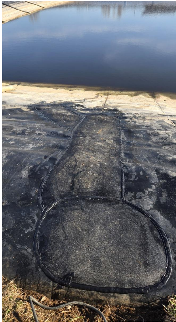
Photo 4: Completed patch in 1991 lagoon, looking north, 03-30-26.
