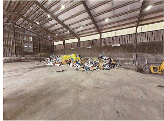
Inside Transfer Building
