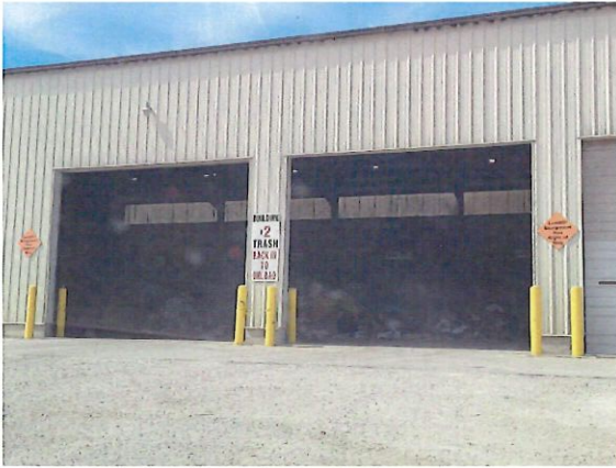
Outside Transfer Building
