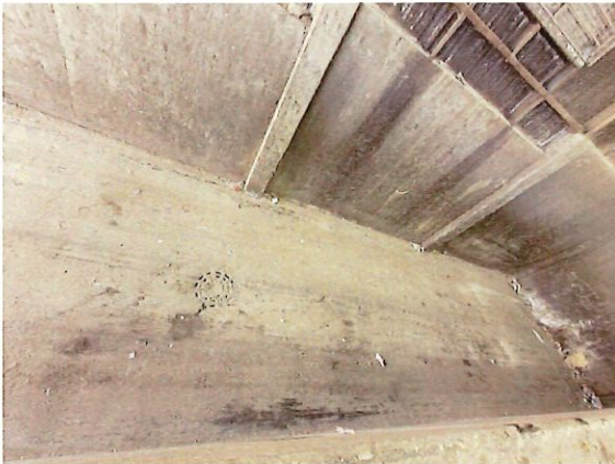
Load Out Pit
