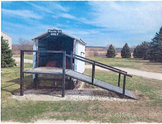
Waste Oil Storage
