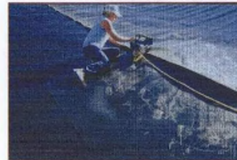
HOT WELDING TWO HDPE LINER SHEETS TOGETHER
