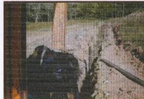
CONNECTING 6 INCH ADS DRAINAGE TILE
