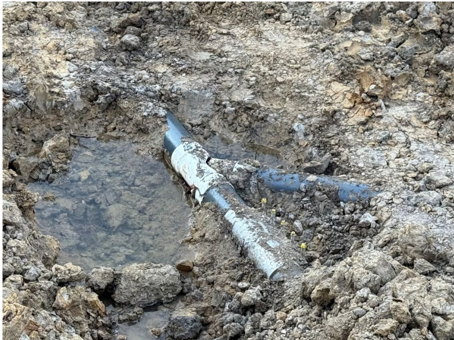
Photo 2 - Repaired leachate line
