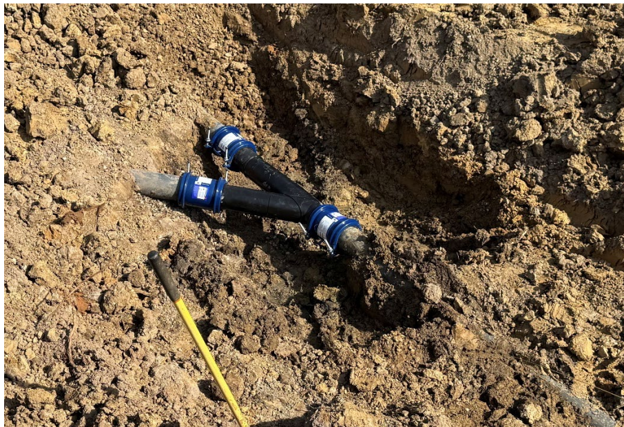
Photo 2 - Repaired leachate line
