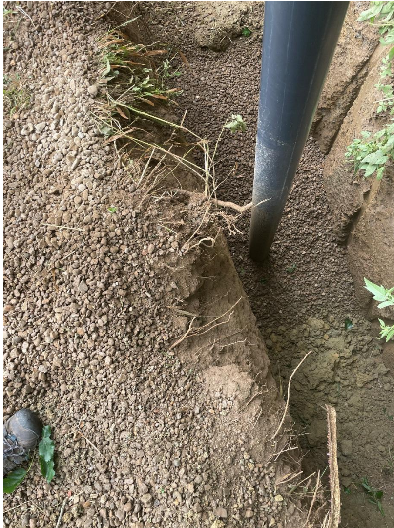
Photo 3: Backfilling trench/riser pipe.
