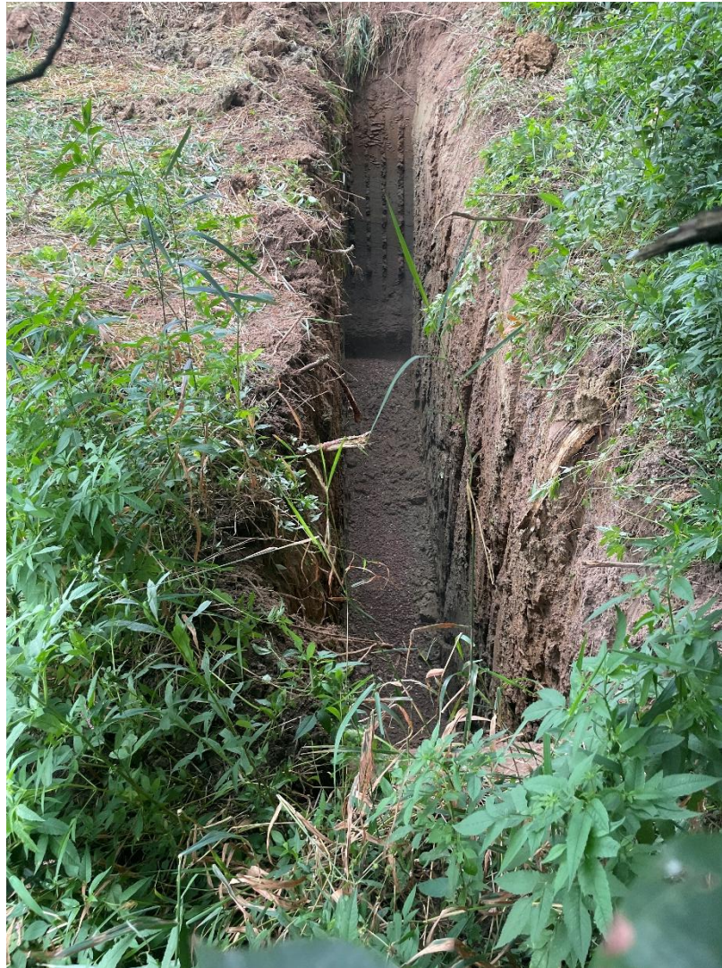
Photo 2: Vent trench excavation.
