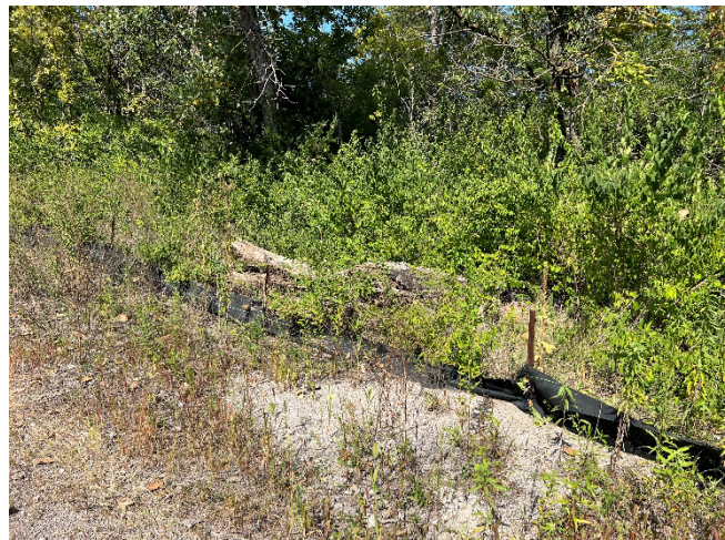
Photo 20: Silt fence damage east of the slag pile
