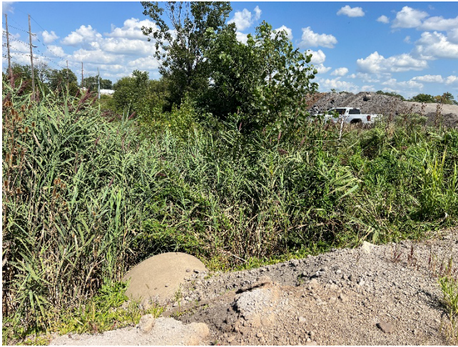
Photo 137: Heavy vegetation around the culvert outlet with riprap erosion protection between the slag storage area and the closed sand storage area
