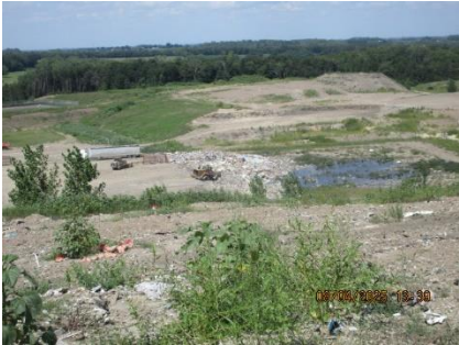
working face in Cell NW2 (ponding)
