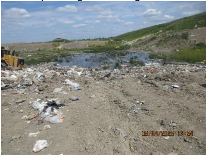
ponding at working face
