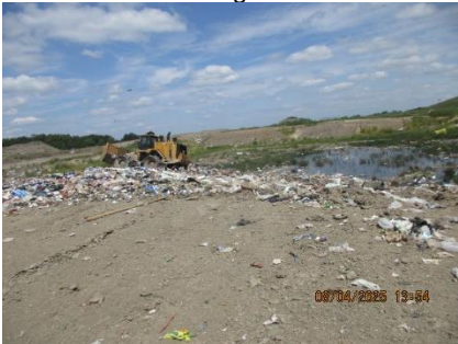
ponding at working face
