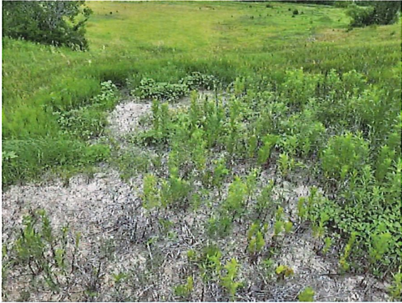
Photo 1: Area of Poor Vegetation on Final Cover
