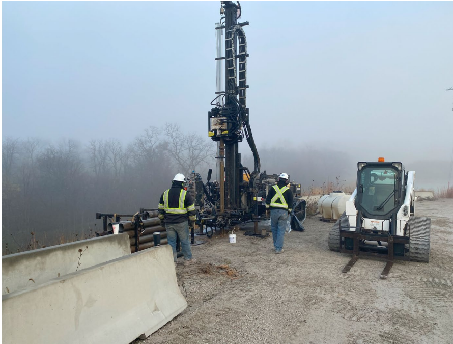
Photo 3: Drilling MW-125. Photo facing Northwest.
