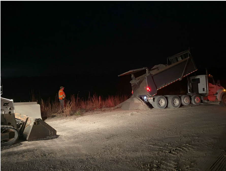
Photo 2: Building pad to drill MW-125 on. Photo facing West.
