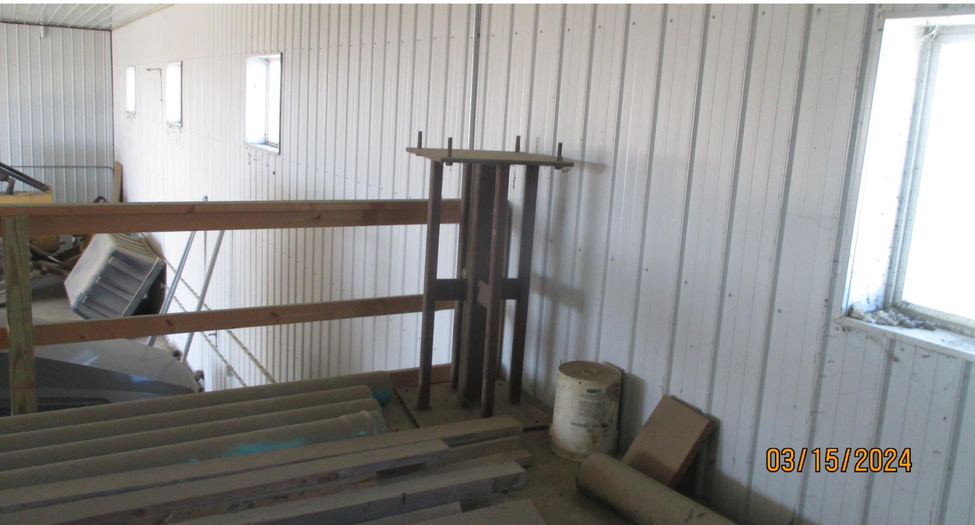
Photo 1: Loadout support base
