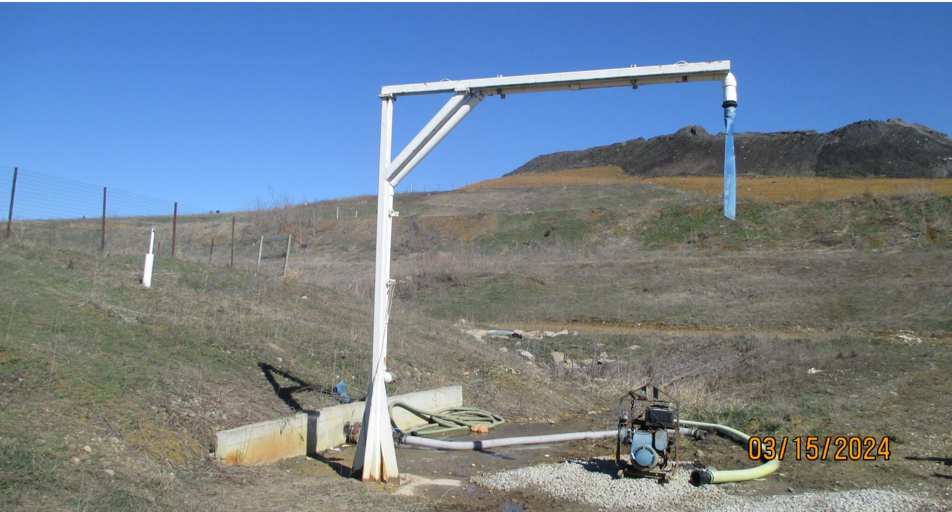
Photo 2: Existing loadout support
