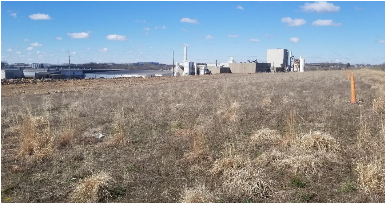
Photo 4 4/19/2019. Top of landfill viewed from the northeast corner looking southwest.
