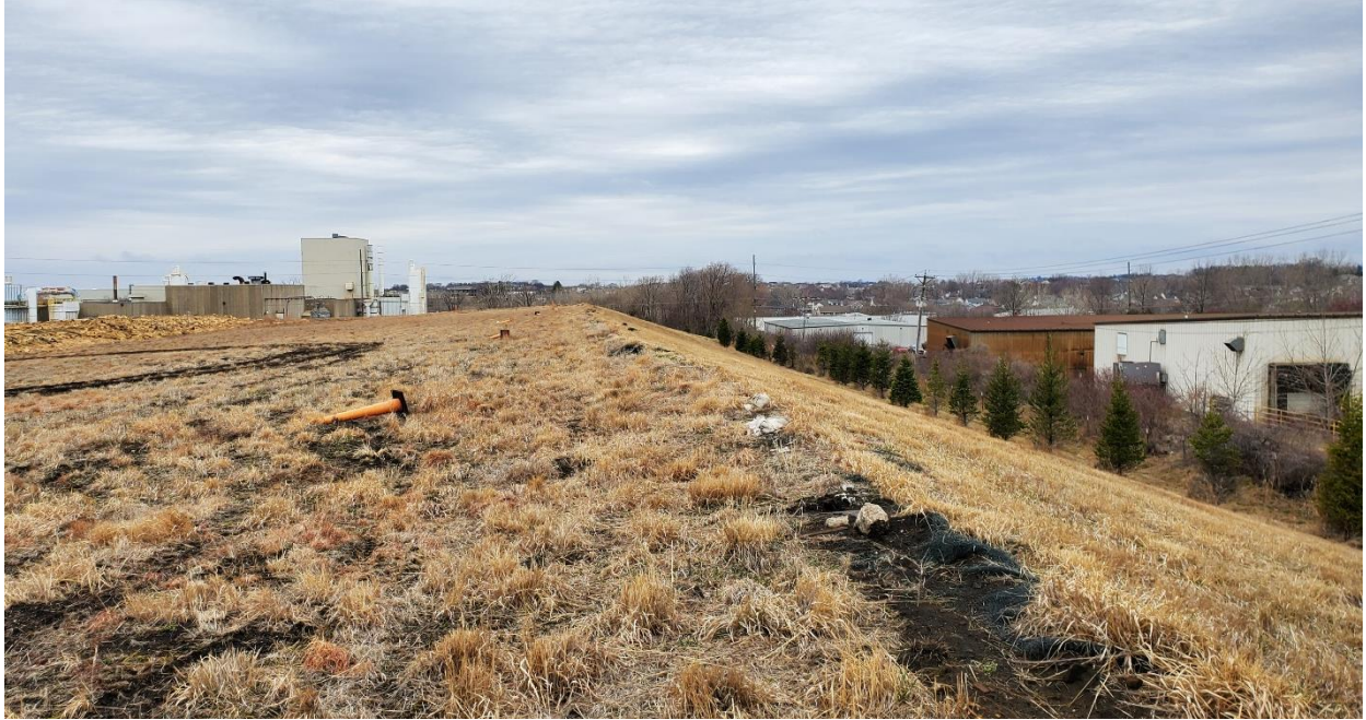
Photo 7 4/13/2022. Top of landfill, facing west from the northeast corner.
