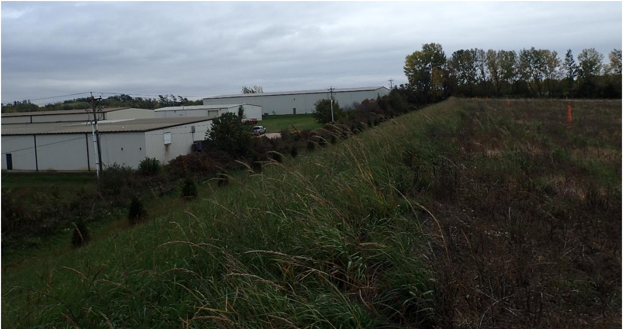
Photo 1 10/14/2016. North area and back side of landfill, looking northeast.
