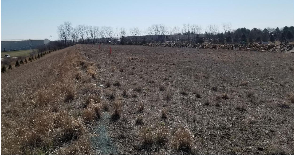
Photo 3 4/24/2018. Top of landfill, facing east.
