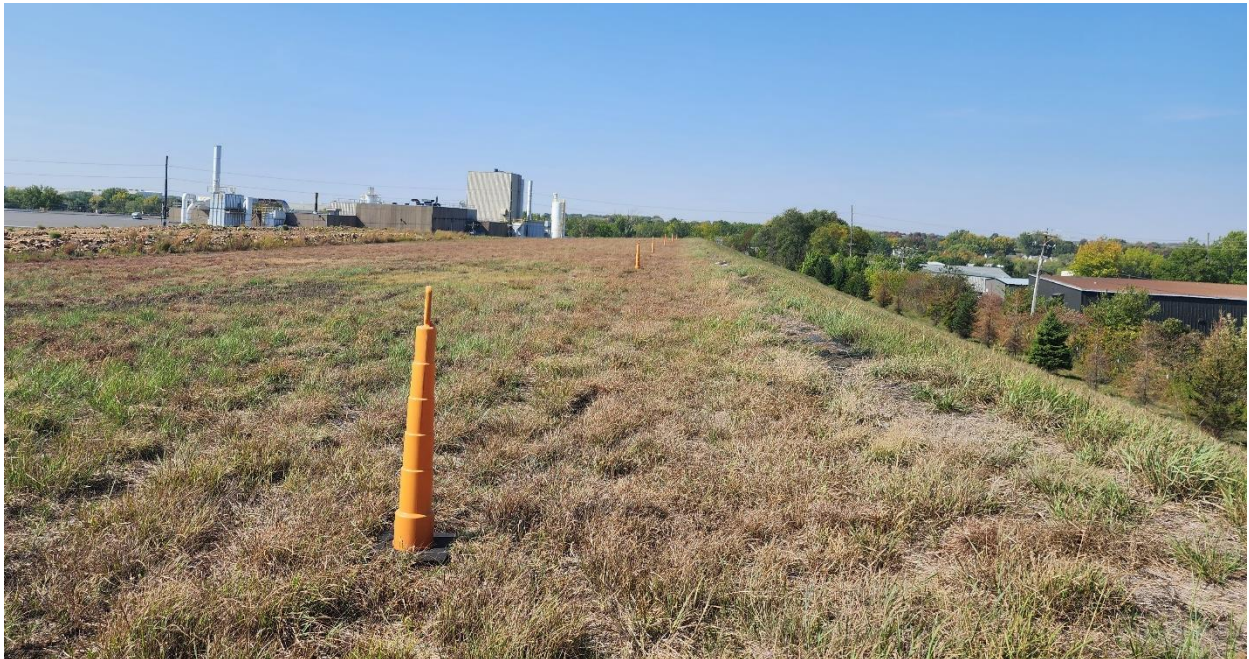
Photo 8 10/2/2023. North area of landfill, looking west.
