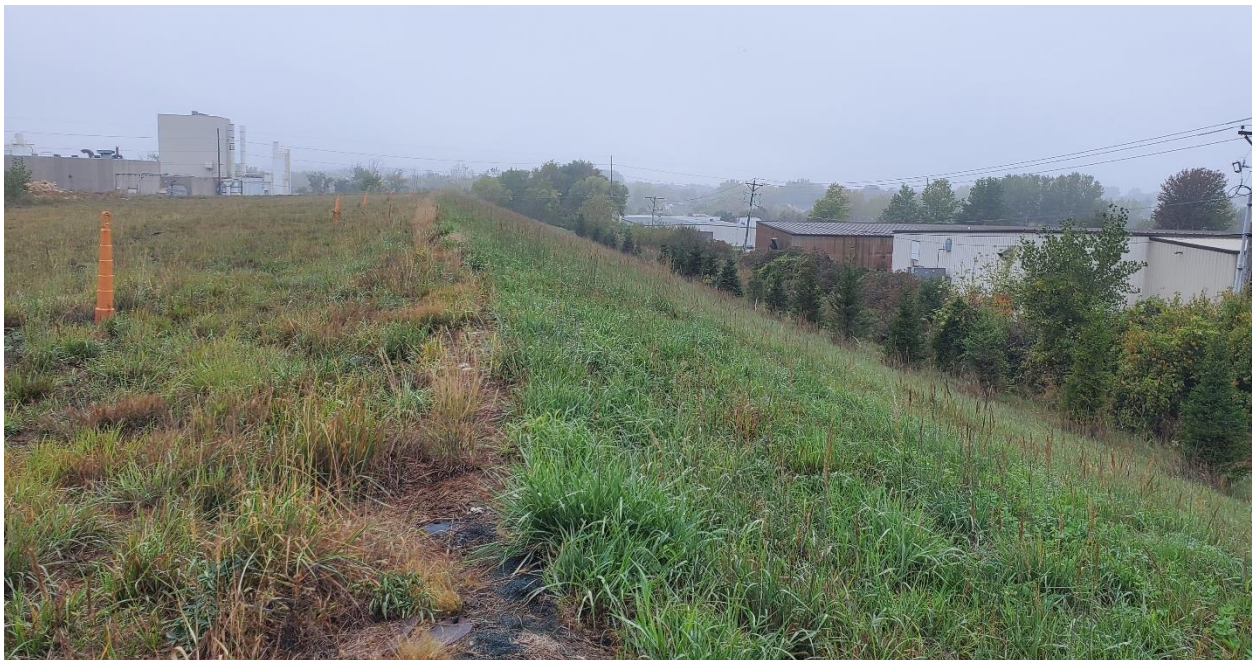
Photo 6 10/7/2021. North area and back side of landfill, facing west.
