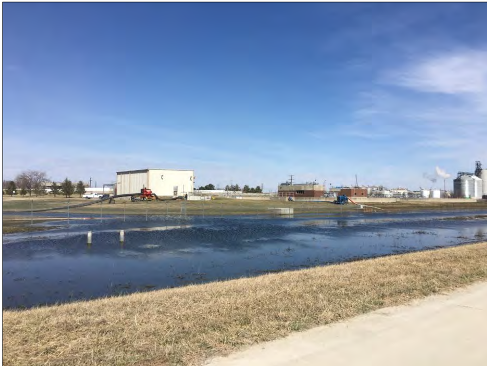
Photo 4 May 2019 treated wastewater release from CBWPCP. View to northeast.
