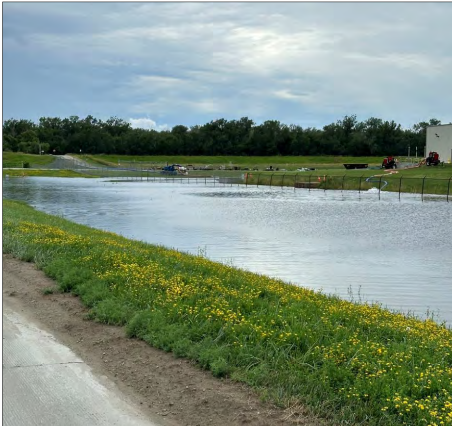
Photo 6 June 2024 treated wastewater release from CBWPCP. View to northwest.
