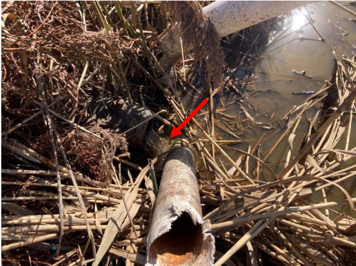
Free flowing water at outlet (during main stem jetting)
