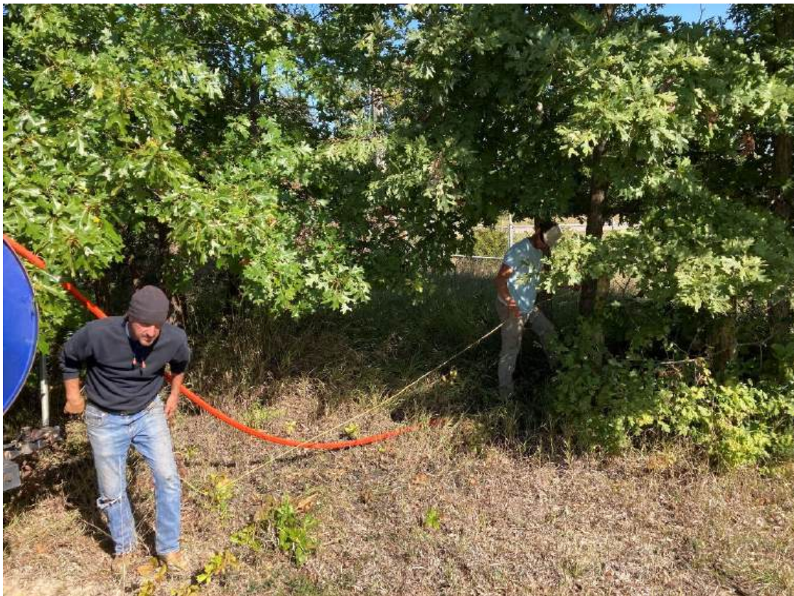
Jetting at northernmost lateral
