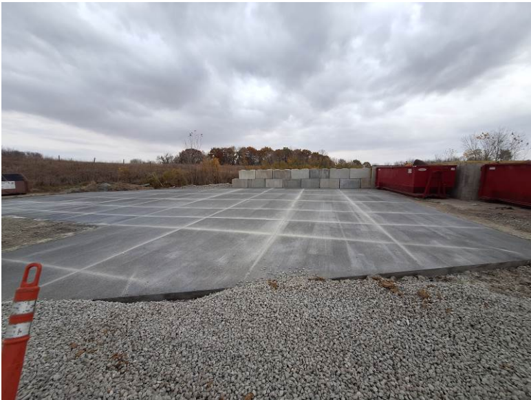
New concrete pad will soon be the scrap metal collection area.
