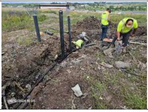
CEC fusing HDPE piping in the trench, facing northeast.
