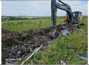
Excavator excavating the trench for HDPE piping, facing southeast.
