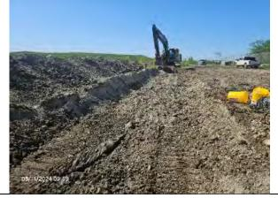
Excavator excavating trench for 12-IN HDPE gas header system, facing south.
