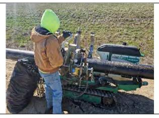
10-IN HDPE piping fusing operations, facing south.
