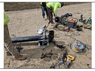
6-IN HDPE piping welding operations, facing southeast.
