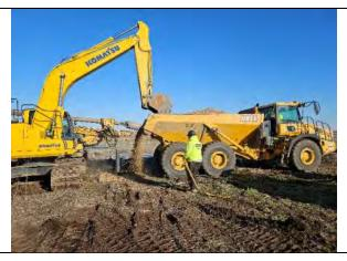
Excavator backfilling well boring with filter pack, facing east.
