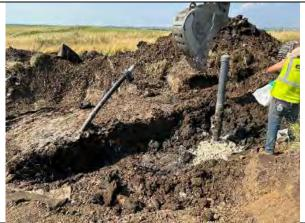
Bentonite plug for the new GW-16R riser and excavation of the GW-16R cap.
