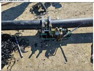
4-IN x 8-IN HDPE piping fusing operations, facing east.
