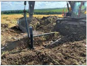
CEC backfilling over the completed geomembrane and geotextile repair maintaining positive drainage for gas extraction lateral, facing south.
