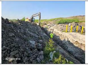
Excavator backfilling the trench and CEC placing warning tape, facing north.
