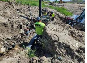
CEC installing 4-IN HDPE caps on condensate cleanout risers, facing south.
