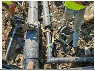
Transition from 4-IN HDPE to 4-IN by 8-IN HDPE piping, facing west.
