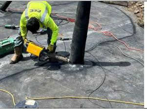
Boot for gas extraction well with liner repair.
