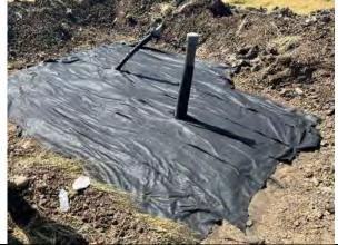
Geotextile placed over the completed geomembrane repair for GW-16R prior to backfilling, facing northwest.
