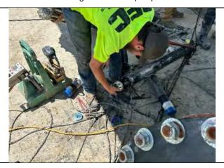
CEC installing new 3-IN fitting on existing leachate pump
