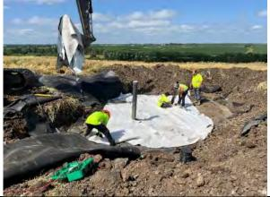
GCL placement for GW-16R liner repair, facing west.
