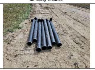
6-IN HDPE piping with 90-degree elbows, facing south.
