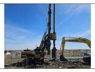
Drilling Rig removing drilled material from its drill, facing east.
