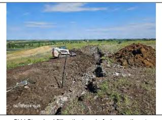
Skid Steer backfilling the trench, facing southeast.
