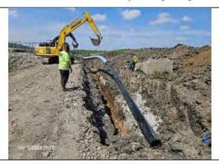
Excavators lowering the 12-IN HDPE gas header pipe, facing north.
