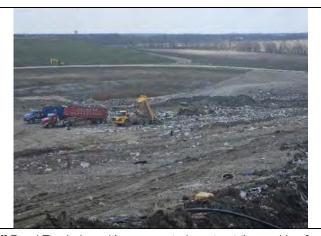
Off-Road Truck depositing excavated waste at the working face, facing southwest.
