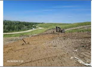
Excavator backfilling portions of previously excavated areas, facing northwest.
