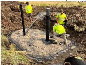
Extrusion welding by CEC for GW-17R, facing northeast.
