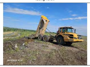
Off-Road Truck depositing soil at the trench, facing southeast.
