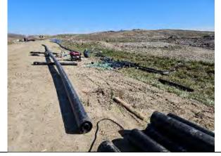
4-IN x 8-IN HDPE piping fusing operations, facing northeast.
