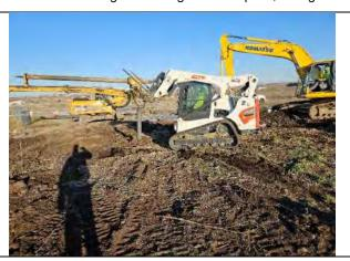
Skid Steer placing well grate over GW-19R, facing east.
