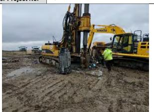
CEC switching to the wet bucket at a depth of 82-FT on GW-26R, facing northeast.
