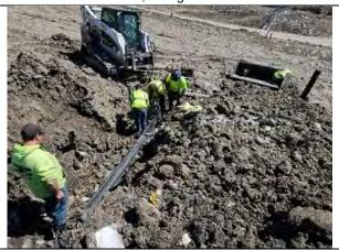
CEC fusing the 6-IN HDPE lateral to the 10-IN HDPE header, facing south.
