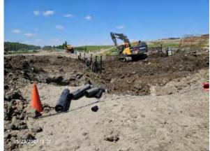
Excavator backfilling the area around the isolation valves, facing north.
