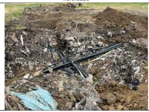
Completed 2" HDPE piping connection near GW-29R, facing east.
