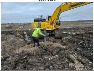
CEC installing the geocomposite ring on GW-27R, facing south.
