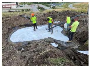
GCL placement for the previous location of GW-16 and gas lateral pipe penetration, facing east.
