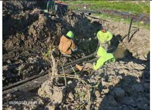
CEC fusing the lateral system to GW-24 to the 12-IN gas header system, facing southwest.
