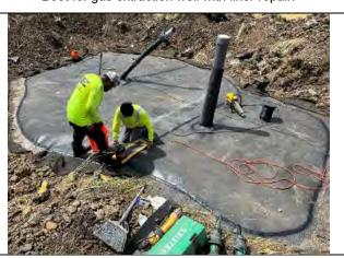
CEC perform vacuum box non-destructive testing for the geomembrane repair.
