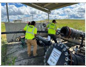
CEC placing the pump and upsized line back into LS-4
