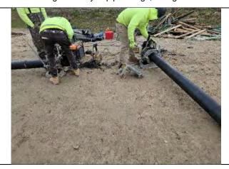
6-IN HDPE piping welding operations, facing east.
