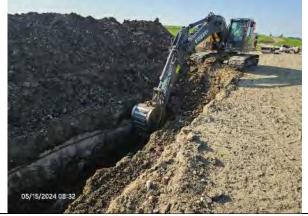
Excavator excavating the trench for the 12-IN HDPE gas header system, facing south.
