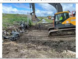
CEC backfilling Wednesday's excavation for the leachate pump tie-in and stormwater discharge repair
