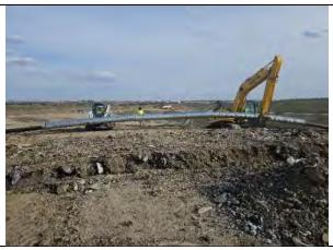
Excavator and Skid Steer setting CMP road crossing into the trench, facing southeast.
