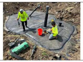
Completed extrusion weld for GW-16R repair, facing northwest.
