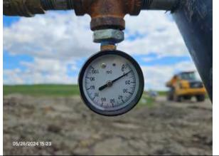
End of pressure test for 2-IN HDPE, facing south.
