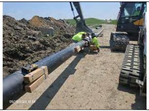
CEC installing wooden blocks under the 12-IN HDPE gas header in the road crossing, facing south.
