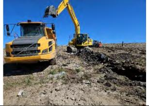
Excavator excavating a trench for the 6-IN HDPE gas lateral to remote well GW-37, facing north.
