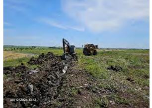
Excavator excavating the trench for the HDPE piping, facing south.
