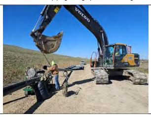
Excavator loading 10-HDPE piping onto the Fusion Machine, facing west.
