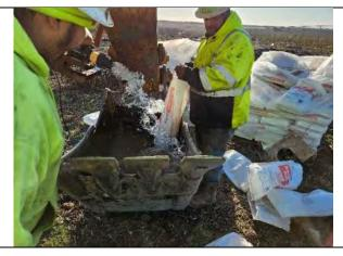
CEC hydrating bentonite in the bucket of excavator, facing west.
