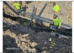
CEC placing trash bag and blind flange on northbound of existing header, facing northeast.
