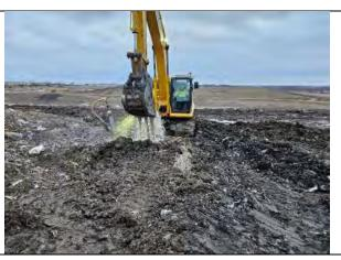
Excavator placing one of the bentonite seals for GW-27R, facing south.
