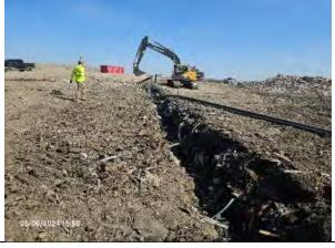
Excavator placing piping into the excavated trench, facing southeast.
