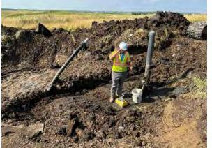
Terracon performing a density test on the GW-16R backfill.
