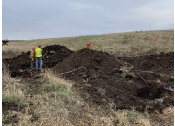
Excavation for existing leachate forcemain near leachate storage tank, facing southwest.
