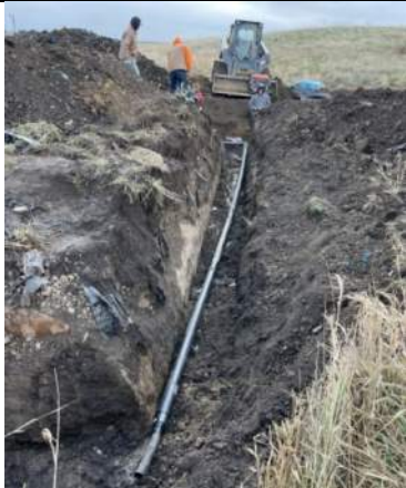
Installation of the leachate forcemain bypass, facing west.
