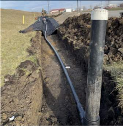
Toe drain piping in the trench, facing north.
