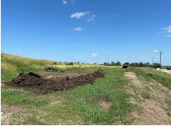
Topsoil being placed near the leachate tank, facing north.
