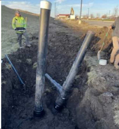
Toe drain removed from previous connection, facing north.
