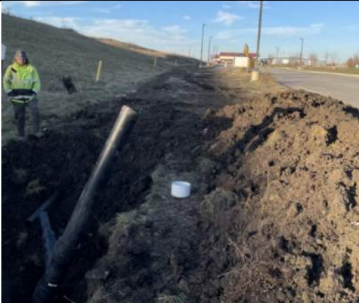
Final grading over toe drain, facing north.
