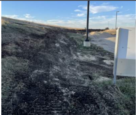
Final grading over toe drain, facing north.
