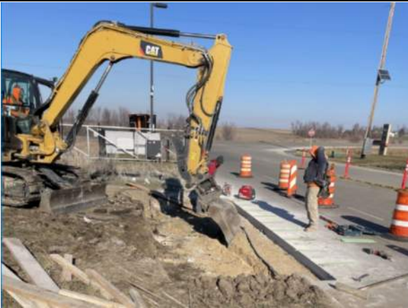
Excavator placing concrete subbase, facing northeast.
