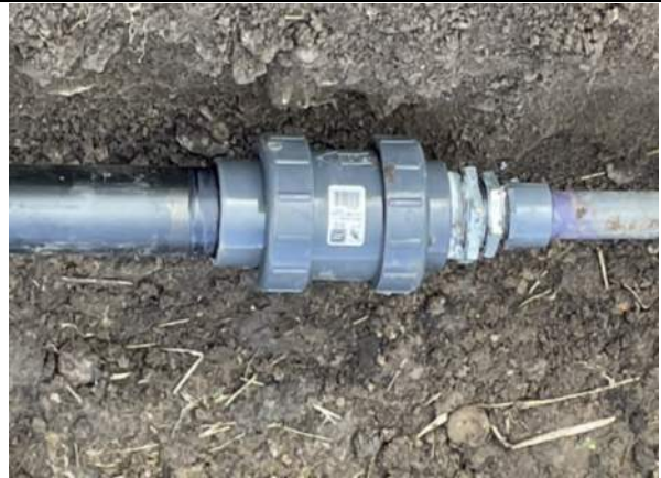
PVC to HDPE adapter, facing south.
