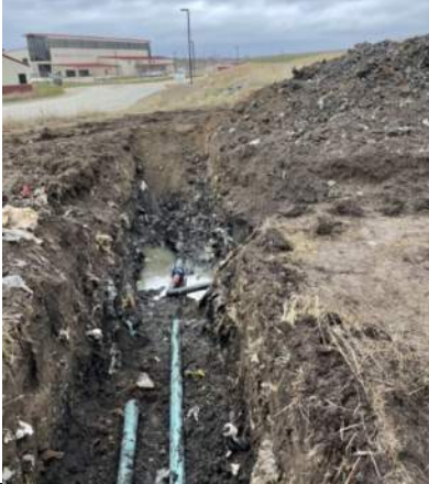
Newly installed bypass around leachate tank, facing south.
