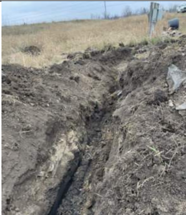
Excavation for existing leachate forcemain near leachate storage tank, facing north.
