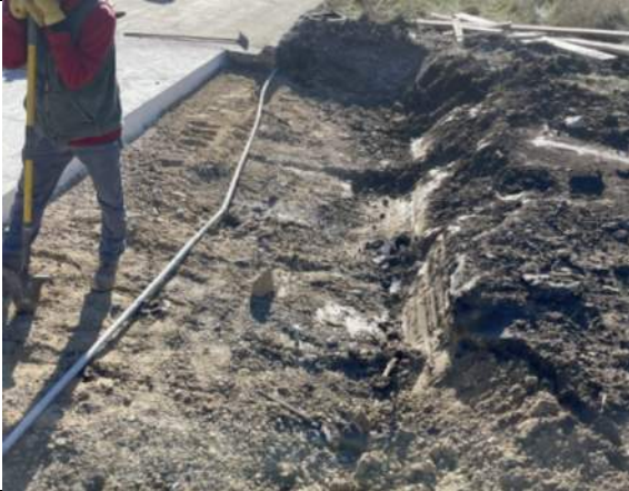
Soil removed for roadway transition, facing south.
