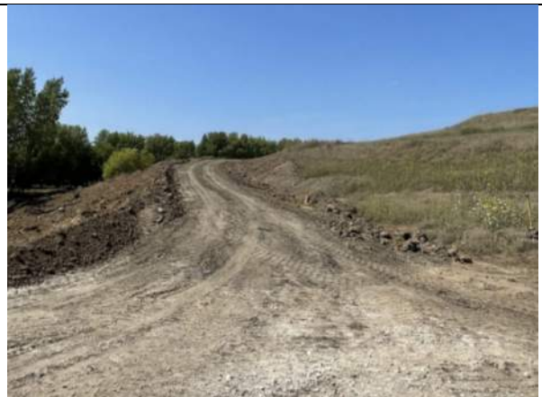
Final cover access road grading work on southern end, facing north.
