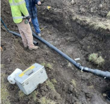
Connection to correct leachate access riser to toe drain, facing northeast.
