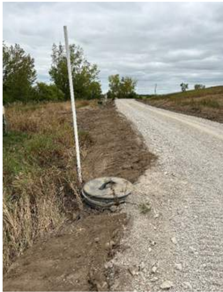
7 - Add markers to riser near edge of road
