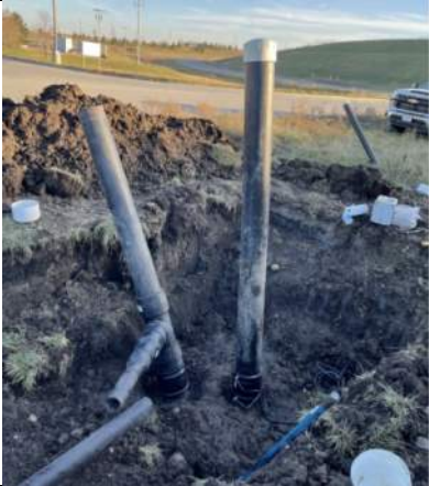
Toe drain removed from previous connection, facing southeast.
