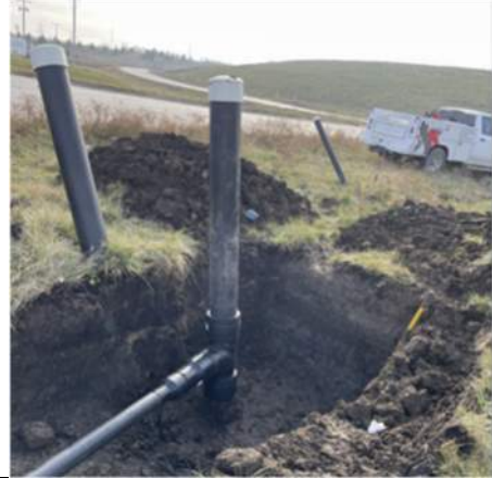
HDPE tee installed to toe drain piping, facing southeast.
