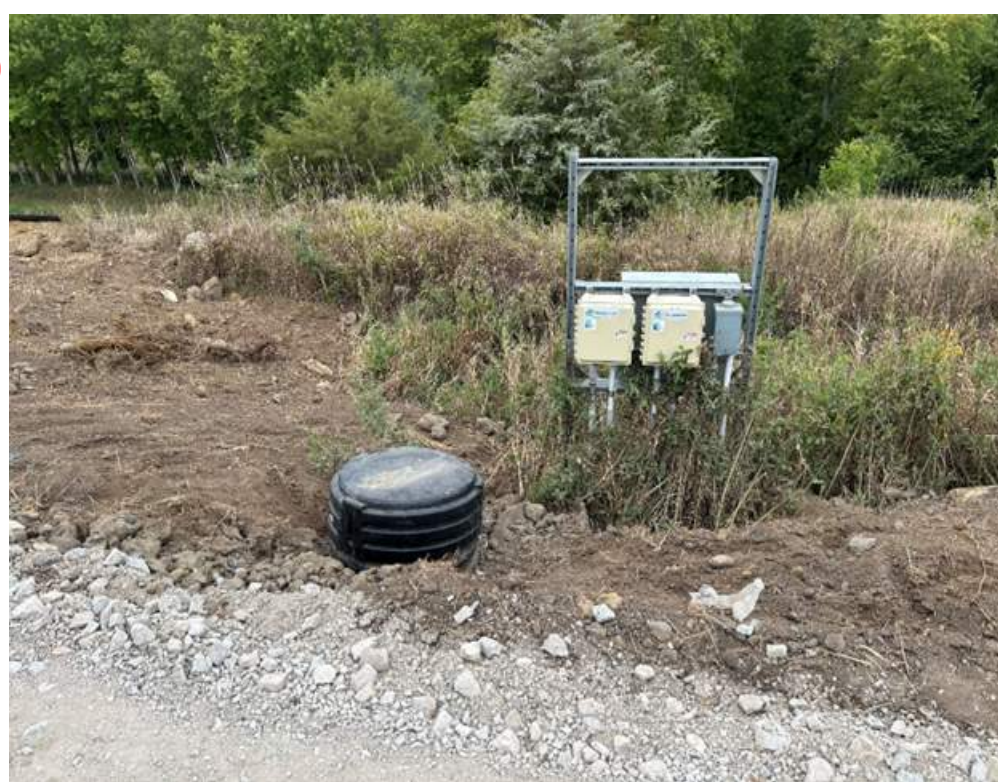
8 - Fill around electrical panel and grade area to drain
