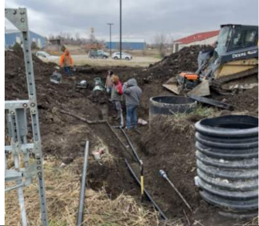
Installation of the leachate forcemain bypass, facing east.
