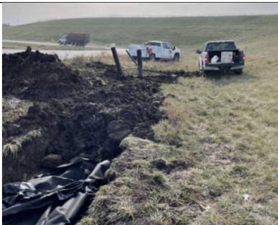
Soil backfill on the toe drain, facing south.
