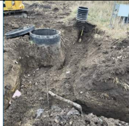
Exposed leachate forcemain near the leachate storage tank, facing north.
