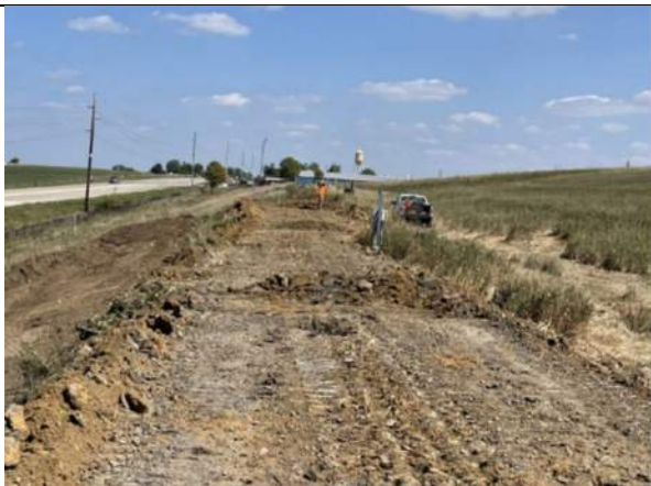
Final cover access road grading work, facing east.
