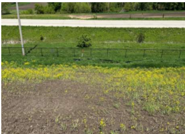
Seeding not taking on the north slope of the final cover access road, facing north.
