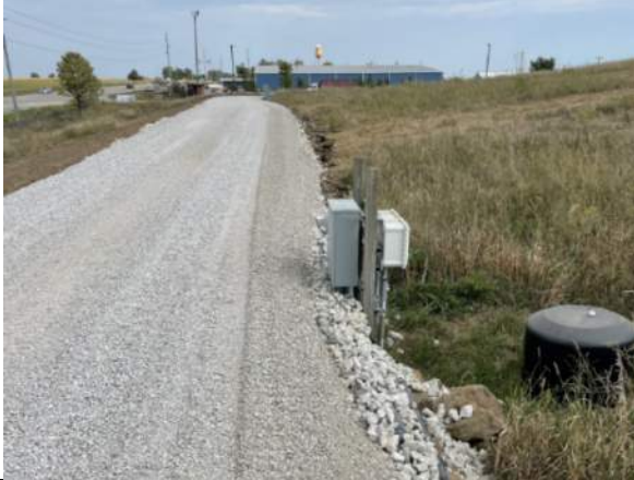
Final cover access road next to existing leachate well, facing east.
