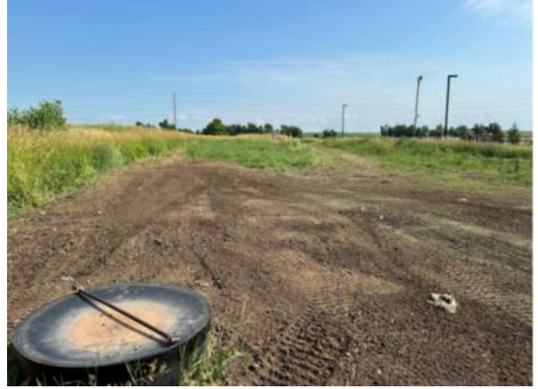
Final grading near leachate tank, facing north.
