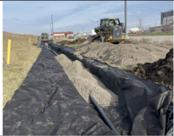
Aggregate being placed in the toe drain trench, facing north.
