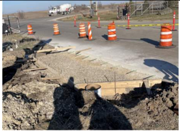
Concrete formwork installed, facing northeast.
