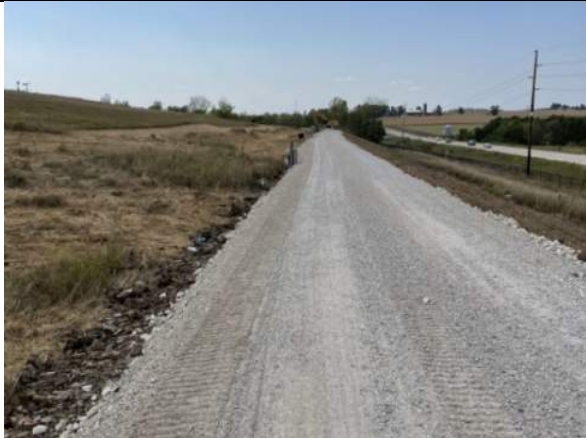
Surface course installed on final cover access road, facing west.
