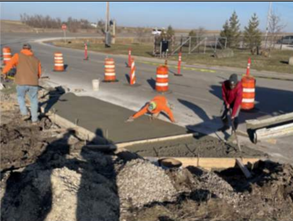
Gensini finishing the concrete, facing northeast.
