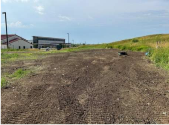
Final grading near leachate tank, facing southeast.
