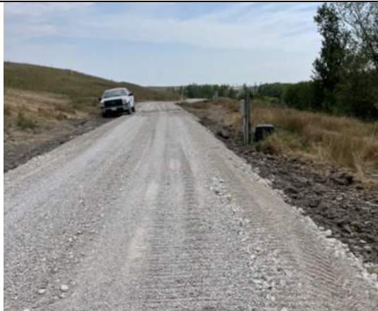
Final cover access road with surface course installed, facing south.
