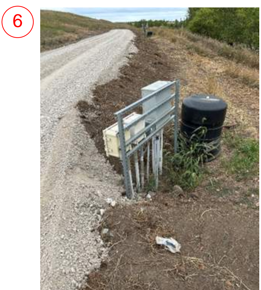
6 - Fill around electrical panel and grade area to drain
