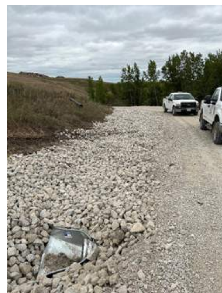
10 - Reshape erosion stone to maintain existing drainage to south
