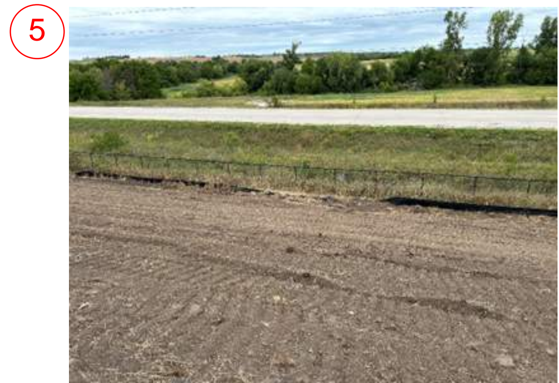
5 - Repair silt fence
