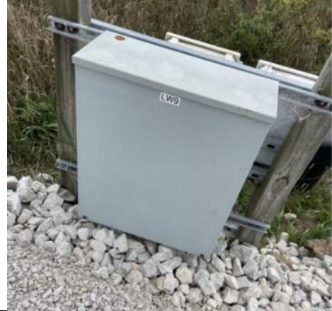
Roadway aggregate close to leachate well, facing southeast.
