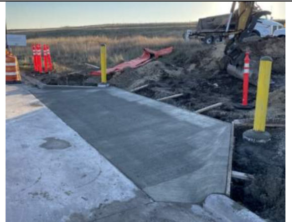
Finished roadway transition, facing southwest.
