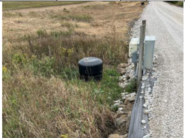
Roadway closed to leachate well, facing west.
