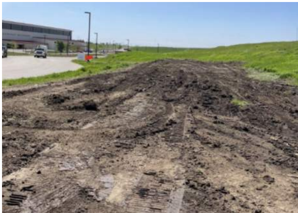
Grading over the leachate storage tank and bypass, facing south.
