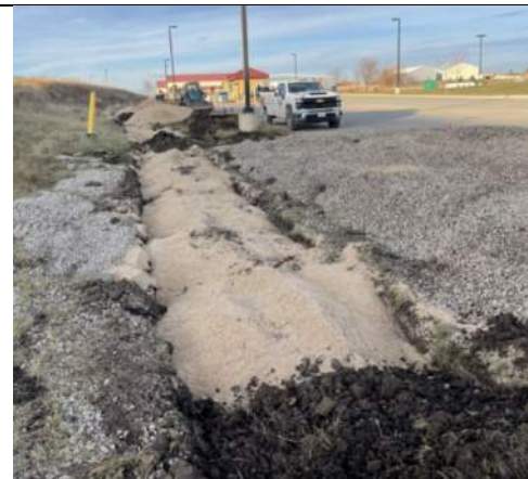
Sand backfill in the toe drain trench, facing north.
