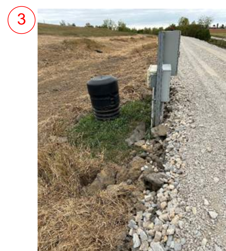
3 - Fill around electrical panel and grade area to drain
