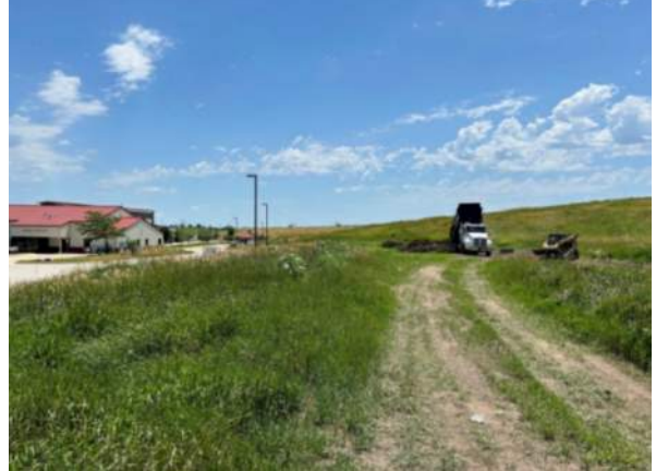
Dump Truck dumping top soil near the leachate tank, facing south.
