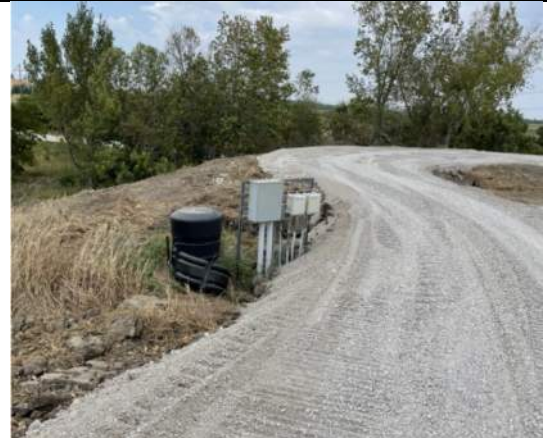
Final cover access road nearing leachate well, facing northwest.
