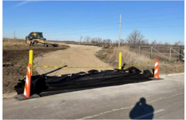
Roadway transition, facing northwest.
