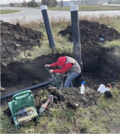
HDPE fusion operations to existing leachate access riser, facing southeast.
