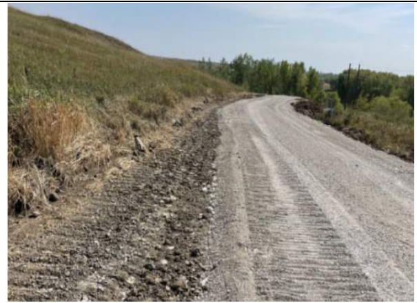
Final cover access road with surface course installed, facing south.
