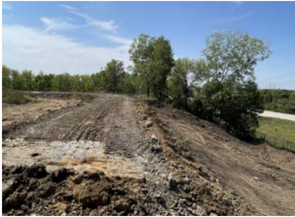
Final cover access road grading work, facing west.
