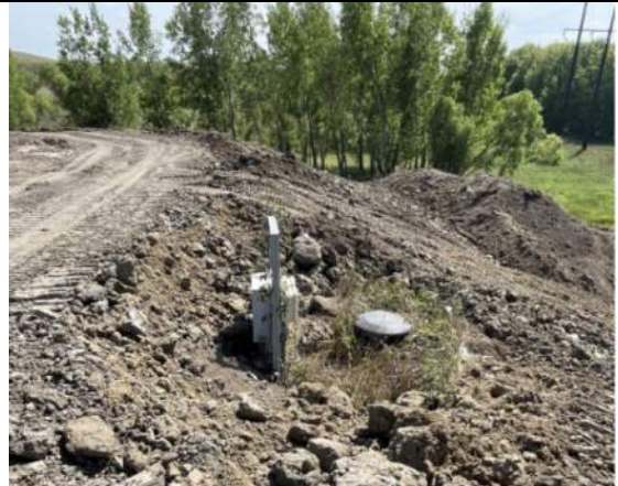
Final cover access road crowding leachate well, facing south.
