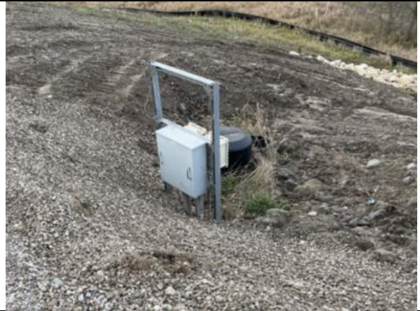
Grading fixed to drain area leachate well, facing southwest.
