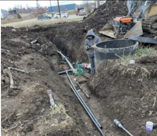
Fusion operations for HDPE piping, facing east.
