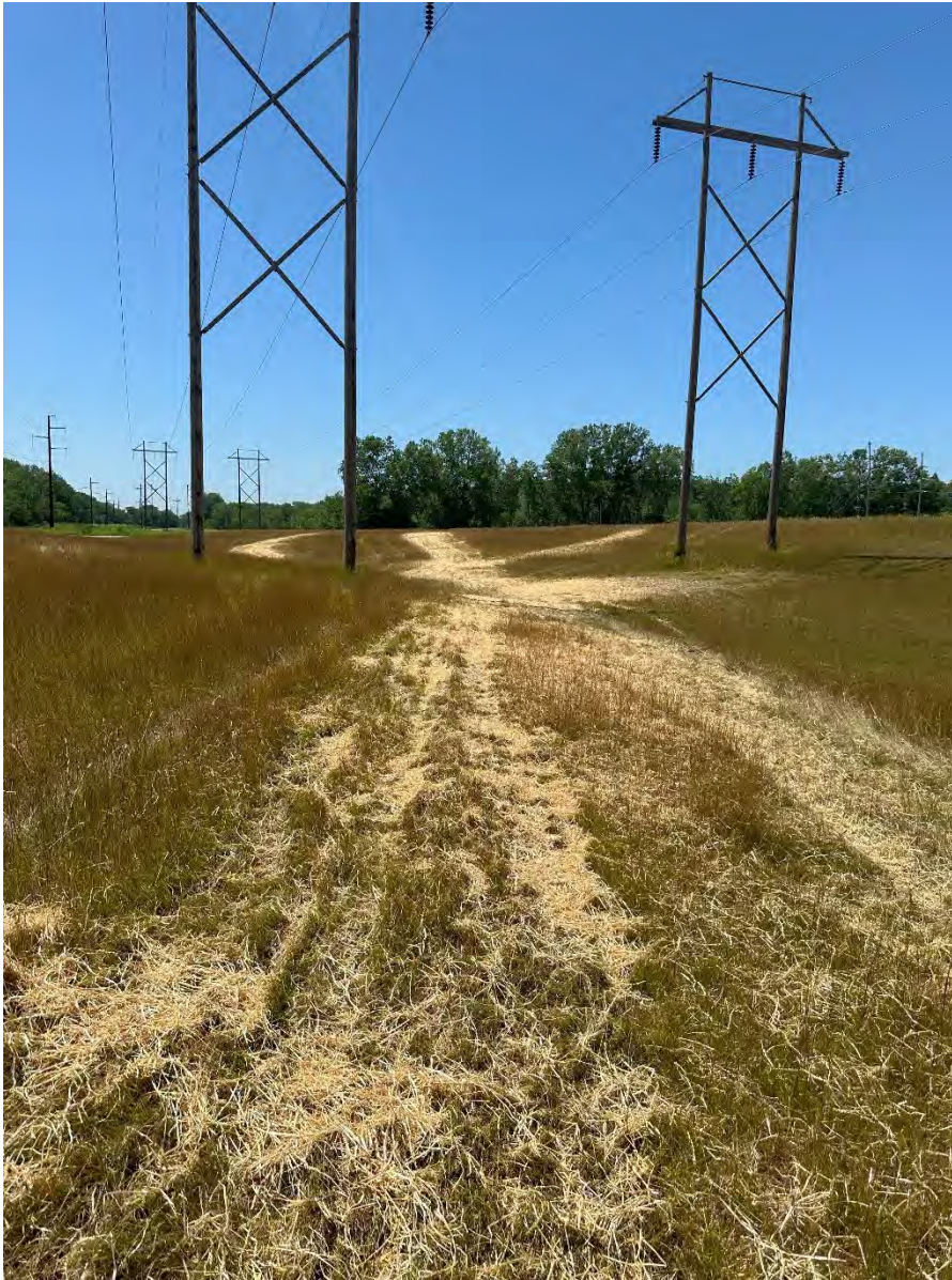
Photo 7: Rutting areas reseeded and mulched in the Main Ash Pond Closure Area (looking northwest).
