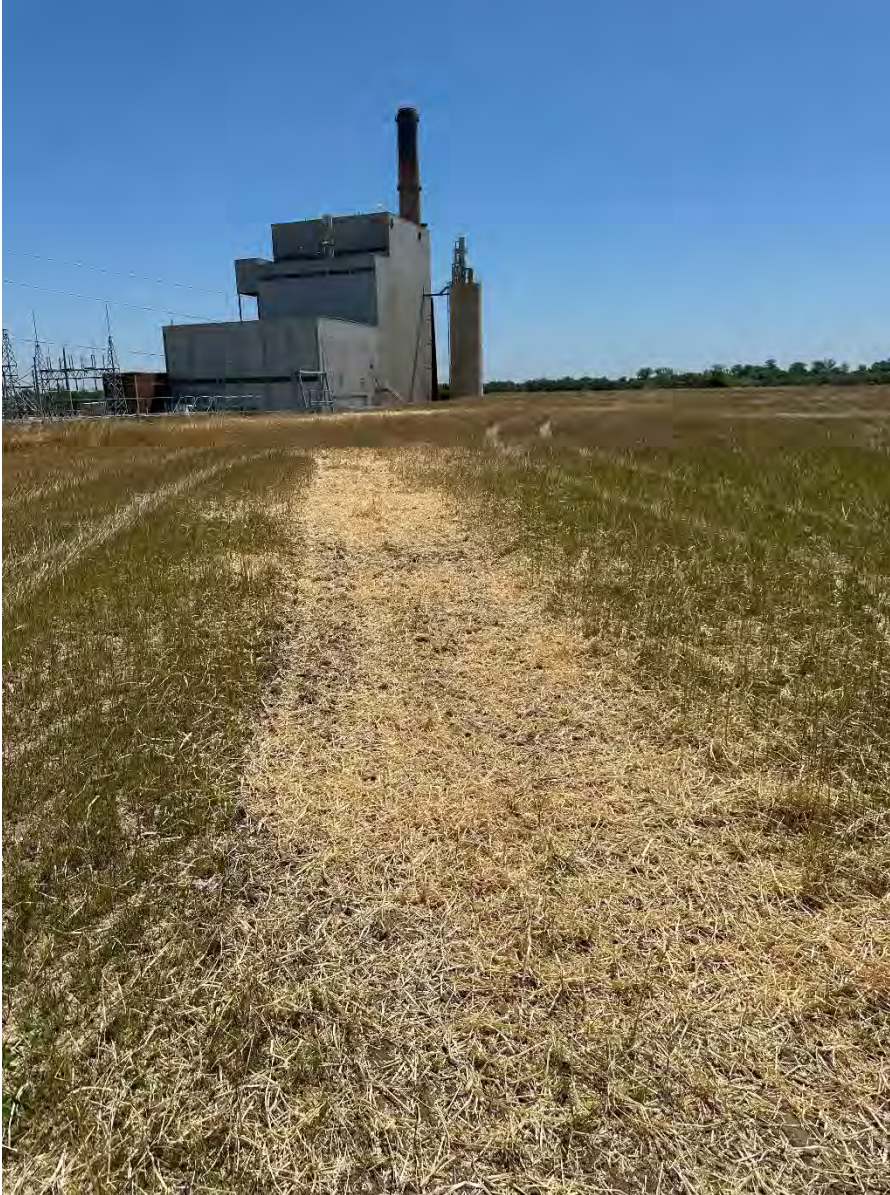
Photo 9: Seeded and mulched rutting on Economizer Ash Pond Closure Area (looking southeast).
