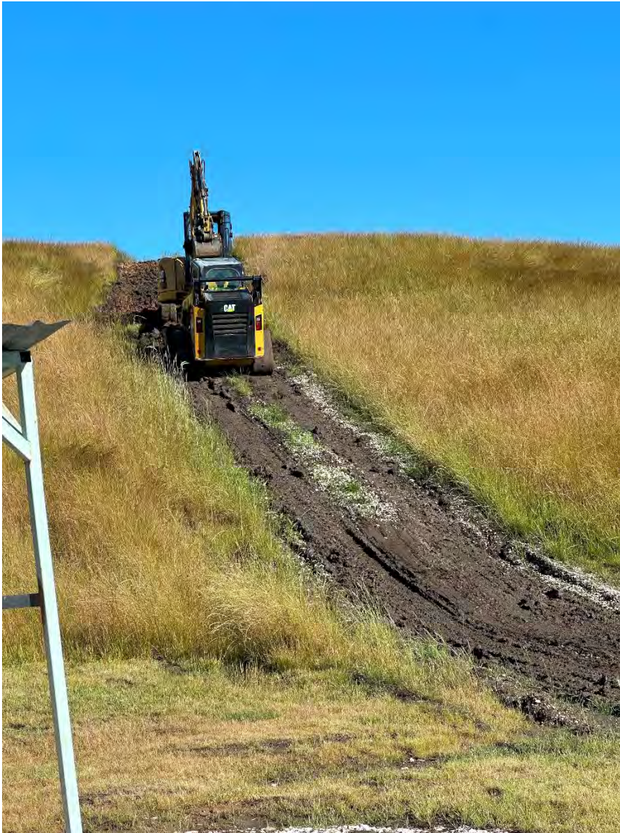
Photo 1: Precision removing topsoil from proposed ramp access (looking west).
