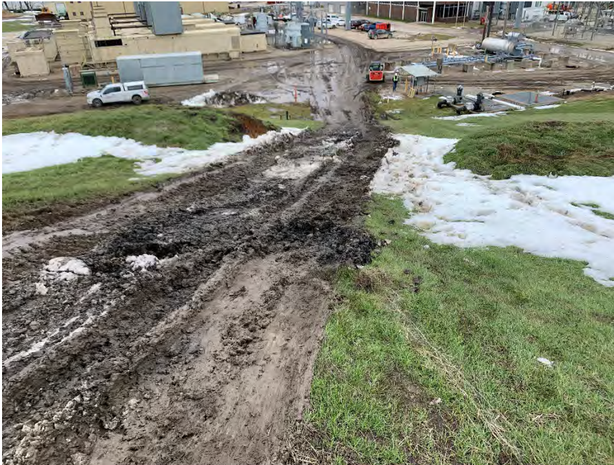
Photo 3: Economizer Ash Pond Closure Area access ramp (looking southeast).
