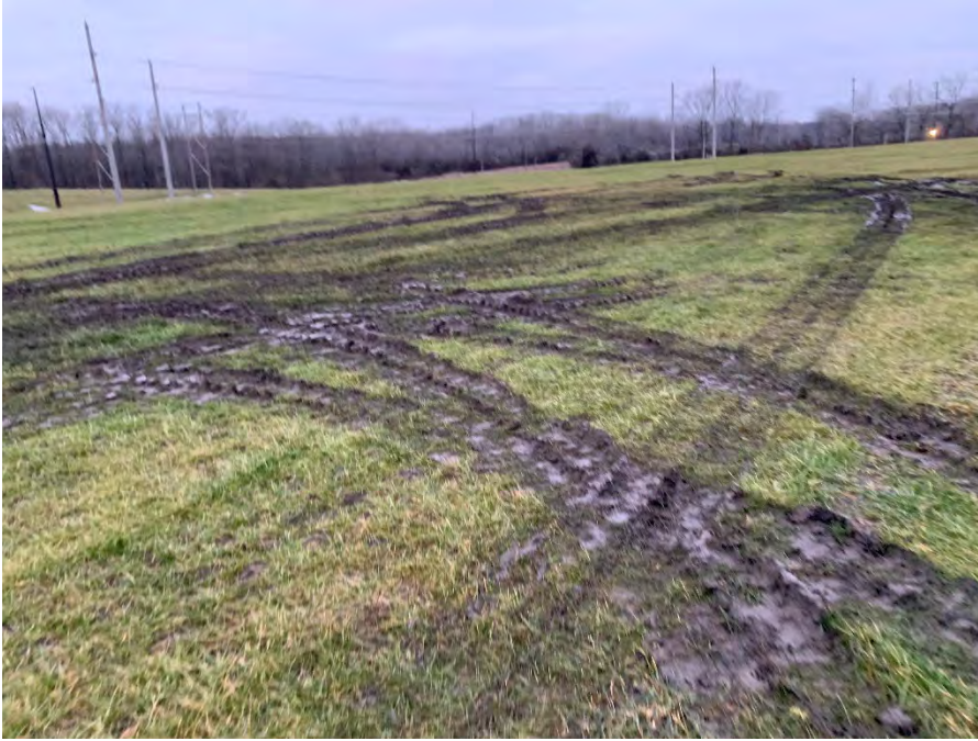
Photo 1: Rutting on the Economizer Ash Pond Closure Area (looking southwest).
