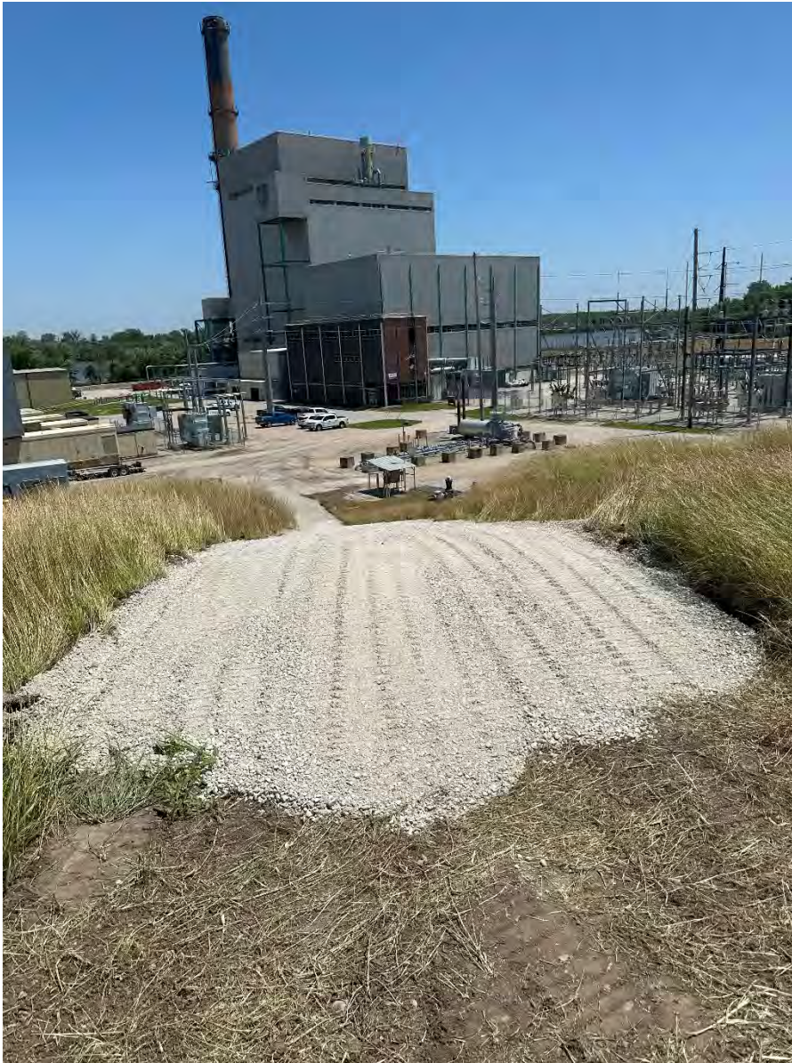
Photo 10: Completed ramp (looking southeast).
