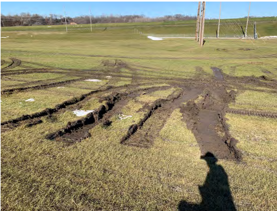
Photo 2: Rutting on the Main Ash Pond Closure Area (looking north).
