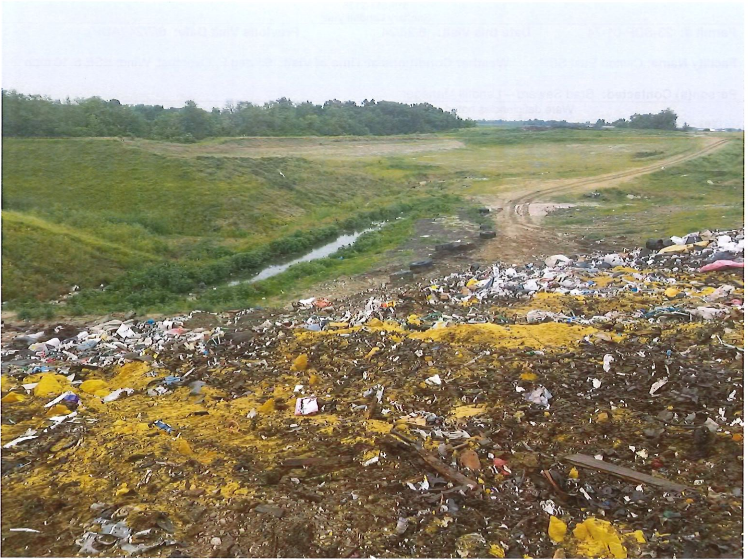
Picture 1. Looking west/northwest from the top of the active working face. No controls are in place across a majority of the toe for storm water that contacts the working face. The edge of the cell is unclear. The ponding in the central portion appears to be off the cell. If the ponding is over the current cell, the ponding will need eliminated.
