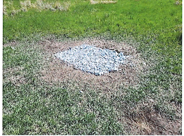
Photo 2: Repairs made after last inspection
