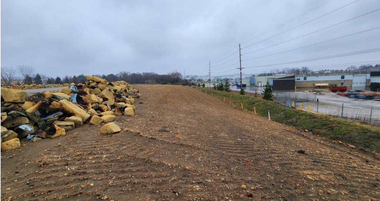
Photo 5. Example of crushed and spread foundry sand with uncrushed blocks on left, on the east side of the landfill.
