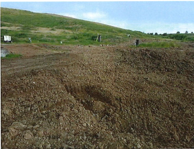
Picture 1: Storm-water Sediment Basin
