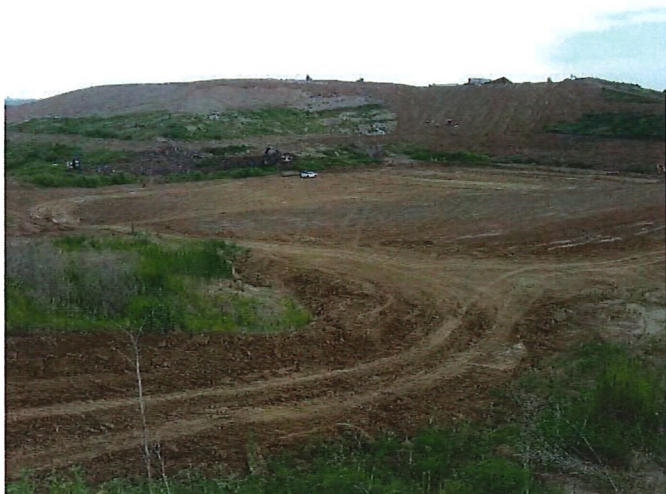
Picture 3: New cell and cover work in background
