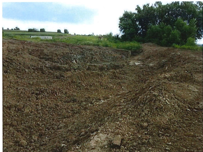
Picture 2: Storm-water Sediment Basin
