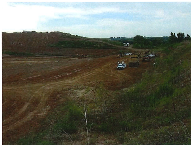
Picture 4: Contractors for new cell
