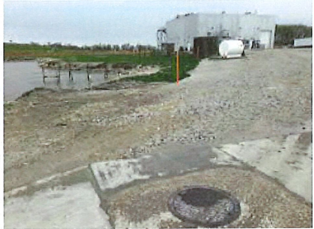
Photos 3 and 4: Looking at the manhole emergency overflow to the lagoon
