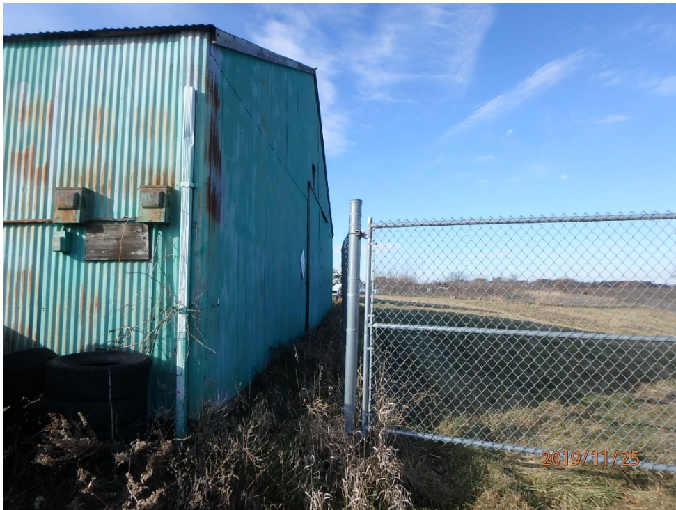
Photo 2 – View of outside of south fence line.
