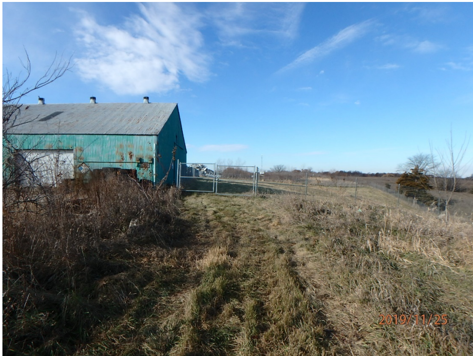
Photo 1 – View of east gate from outside of the capped area.
