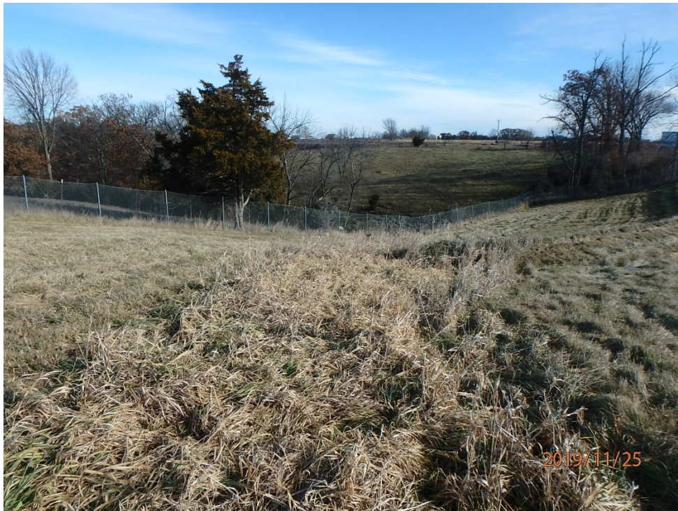
Photo 8 – Rip-rap lined drainageway.
