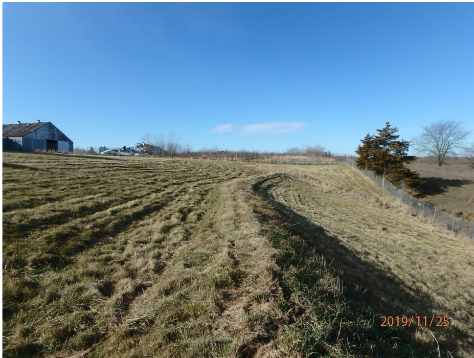
Photo 13 – View along terrace to the rip-rap lined drainageway.
