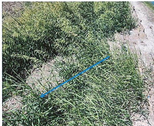
Photo #3: South side of basin with evidence of overflow on berm and dead grass present
