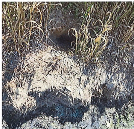
Photo #: Animal burrow just above waterline of basin
