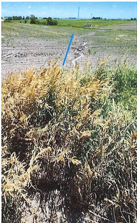
Photo #: Looking east from eastern berm with dry trench present
