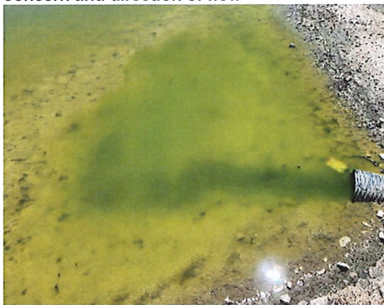
Photo #: Inlet pipe from primary retention basin with green water flowing in
