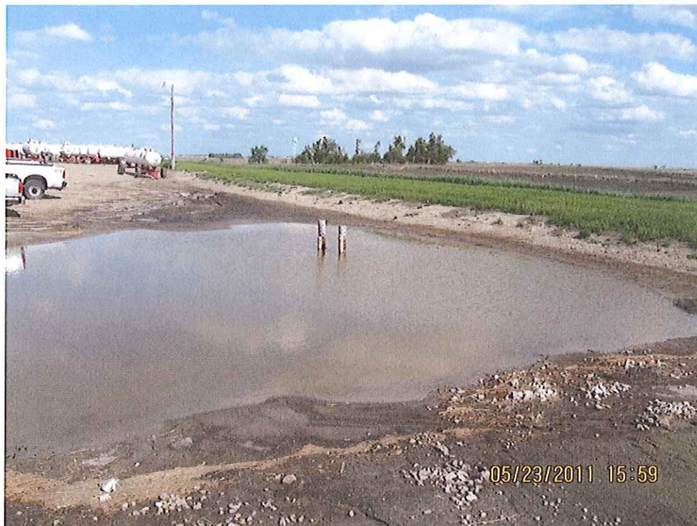
Above and Below: Photograph of Agriland catchment basin. Note the two intakes located inside the basin. These intakes are operated by a manual gate valve.
