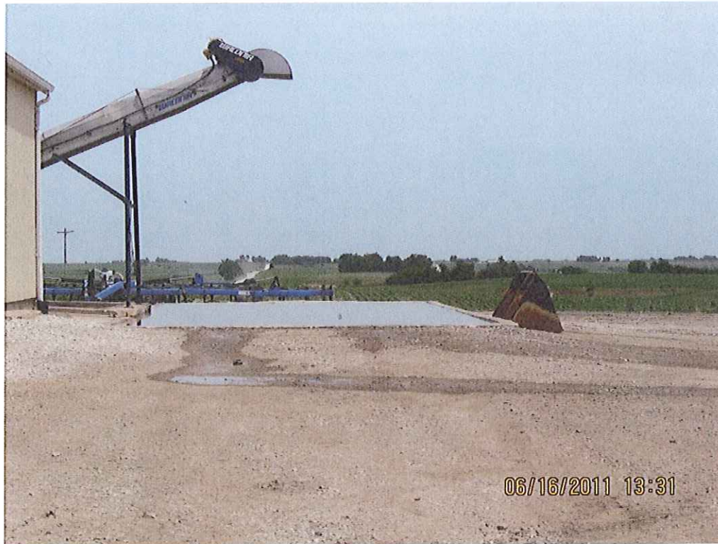
Above and Below: Concrete basin located beneath dry fertilizer load out filled to capacity with liquid. Liquid leaving basin on east and west sides. Liquid directed towards tile intake.
