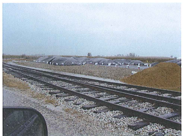
Soil stockpile area showing that the contaminated soil is contained and protected from the weather.
