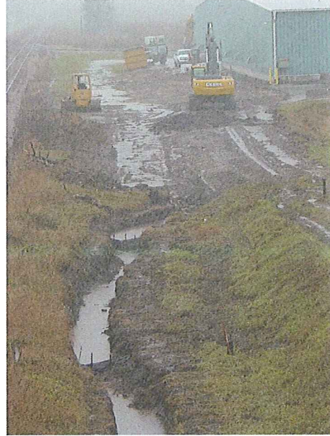
Upper end of ditch showing silt fences and the area where removal of the tile was occurring. Note: water was diverted around the west side of the work site.
