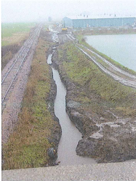
Ditch cleaned out from old tile outfall to where the spill had been stopped.
