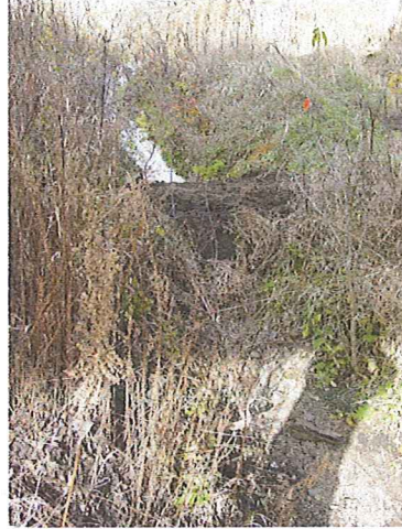
Dike to stop flow in ditch
