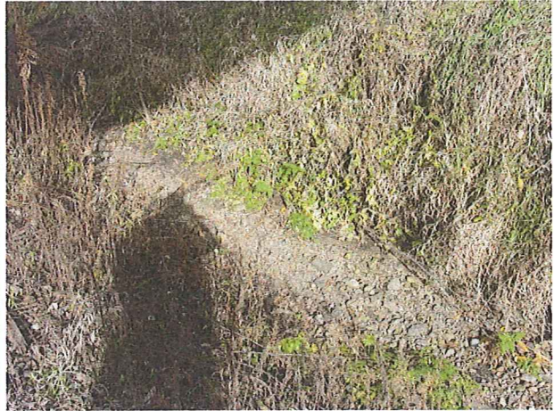
Dry ditch downstream of the dike
