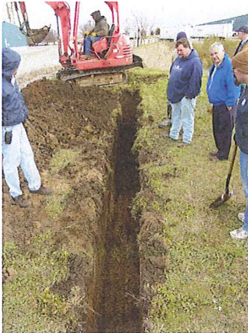
Locating the tile line closer to the building and plugging it
