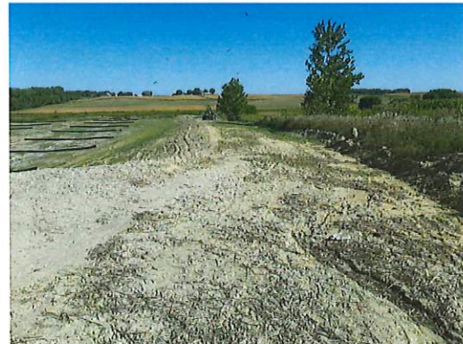
Gully erosion occurring on east berm of the new cell, no sediment leaving the site.
