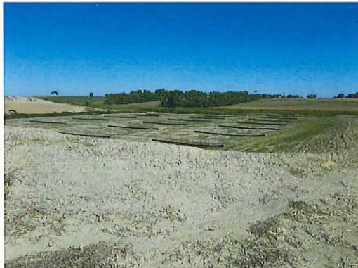
New cell constructed with silt fence installed.
