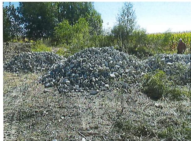
Rip rap that will be installed along south boundary and at the catchment outlet.
