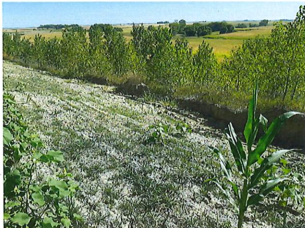
Picture taken looking northeast from east berm toward the crop field shows a cut bank with vegetation between the disturbed soil and the crop keeping sediment on the landfill property.
