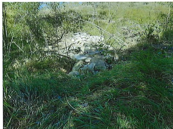
Rip rap installed in the channel leading to the storm water catchment to slow down flow and minimize sediment delivery to the catchment.
