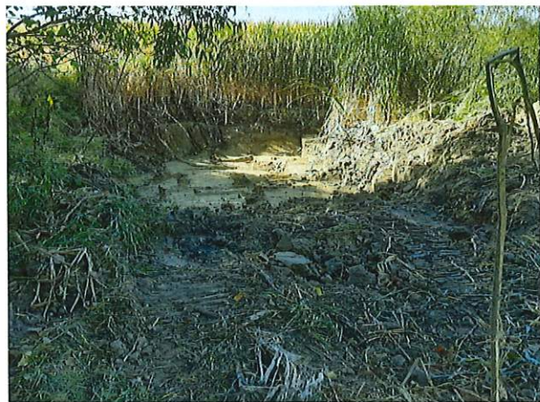
Silted-in stormwater catchment has been cleaned out.
