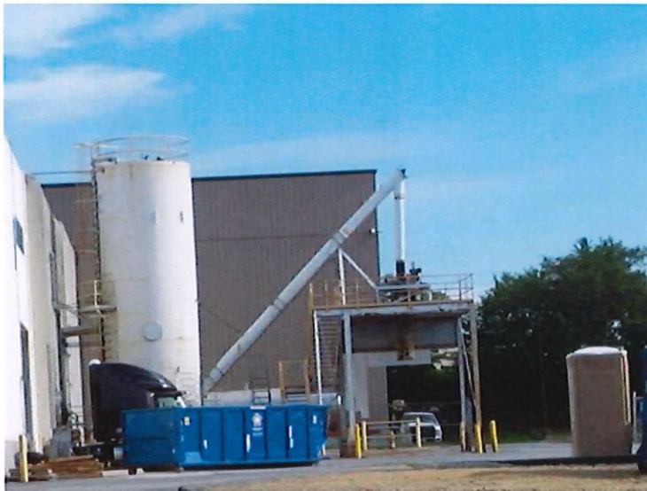
View looking north at the tissue loadout (EP-23) from the south.
