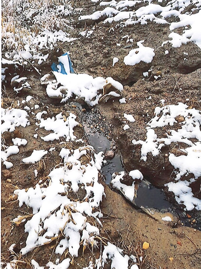
Photo 5. Example of seep found on side slope
