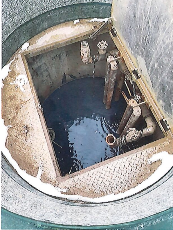
Photo 2. Leachate collection pit with leachate
