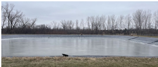
south lagoon cell looking south
