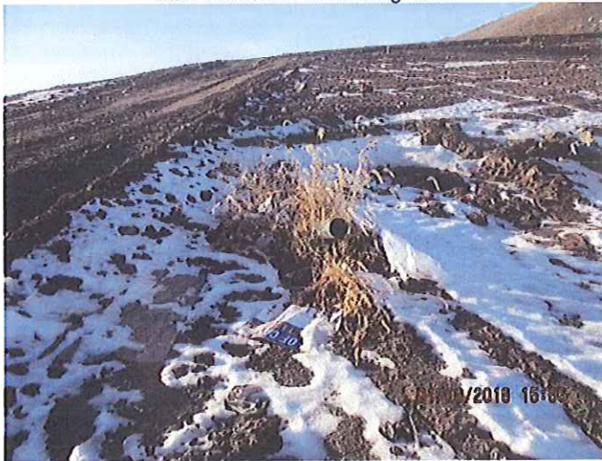
east end of Cell 2
