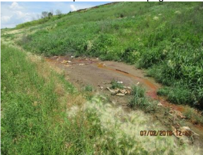
west slope leachate seepage
