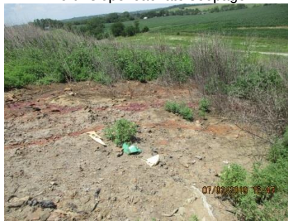
north slope leachate seepage
