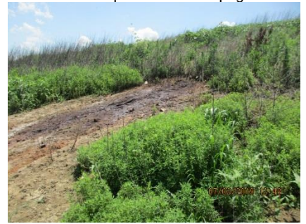
north slope leachate seepage
