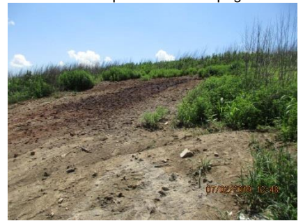
north slope leachate seepage
