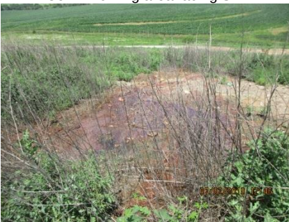
north slope leachate seepage
