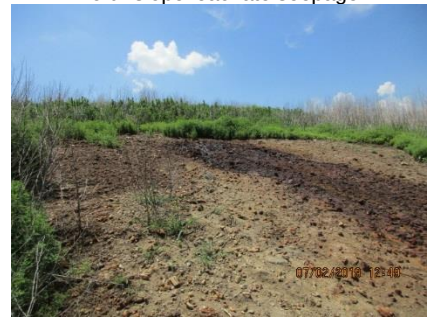
north slope leachate seepage
