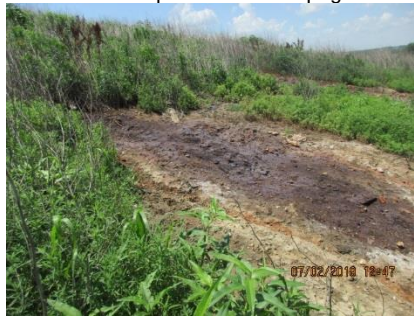
north slope leachate seepage
