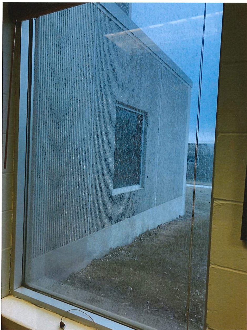
Picture 5 demonstrates an impacted window that is coated in dirty water droplets from the scrubber events.
