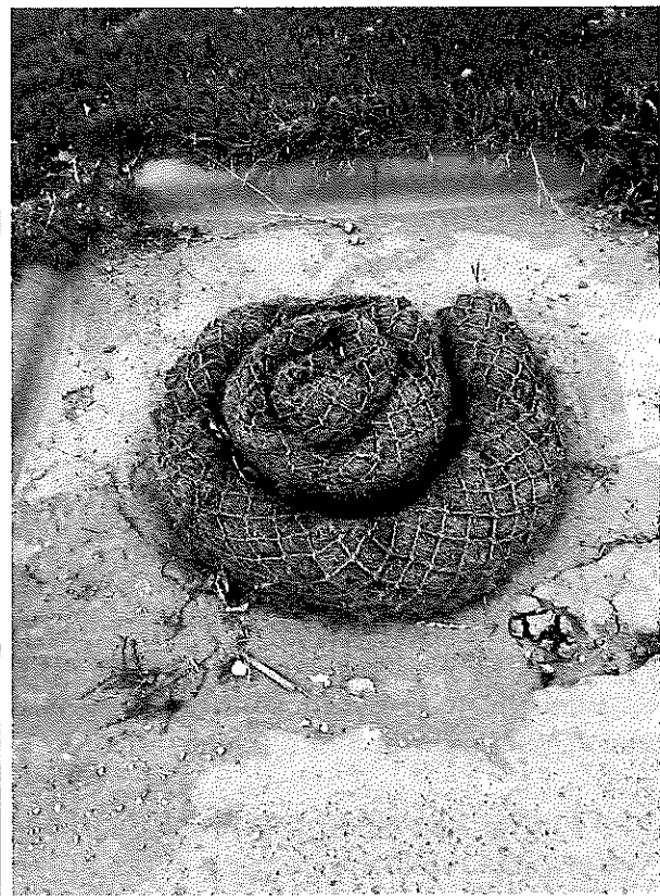
Pictures taken by David Knoll and Kayla Beck of FO #2 on December 14, 2020. Pictures 1 and 2 demonstrate two different storm water intakes at Lehigh Cement Company. Water flowing in Picture 1 is clear and free from sediment. Picture 2 shows the protection provided by straw wattles covering intakes.
